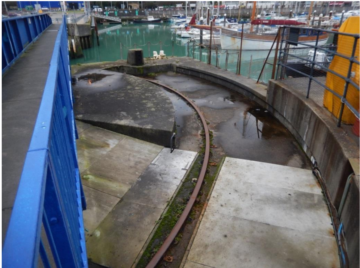
Plate 25: The swinging track of the swing bridge, looking west, 25/01/2016, DHB.
