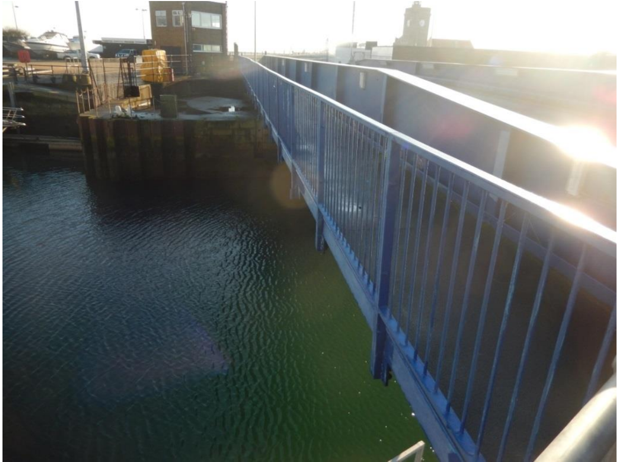
Plate 26: Image of the north side of the pedestrian walkway of the bridge, 25/01/2016, DHB.
