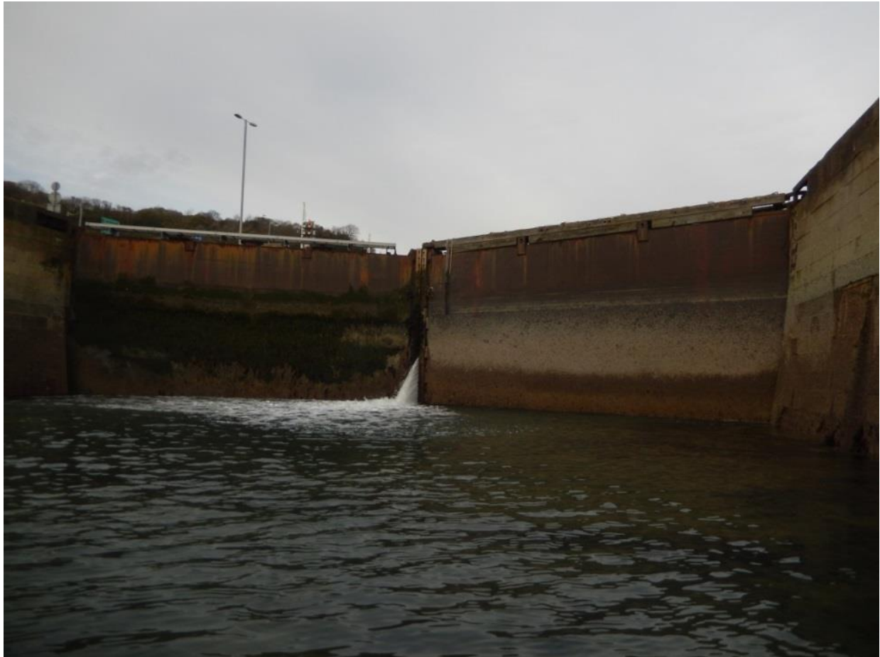
Plate 32: Water coming through the back of the Wellington Dock Gates, looking north, 25/01/2016, DHB.
