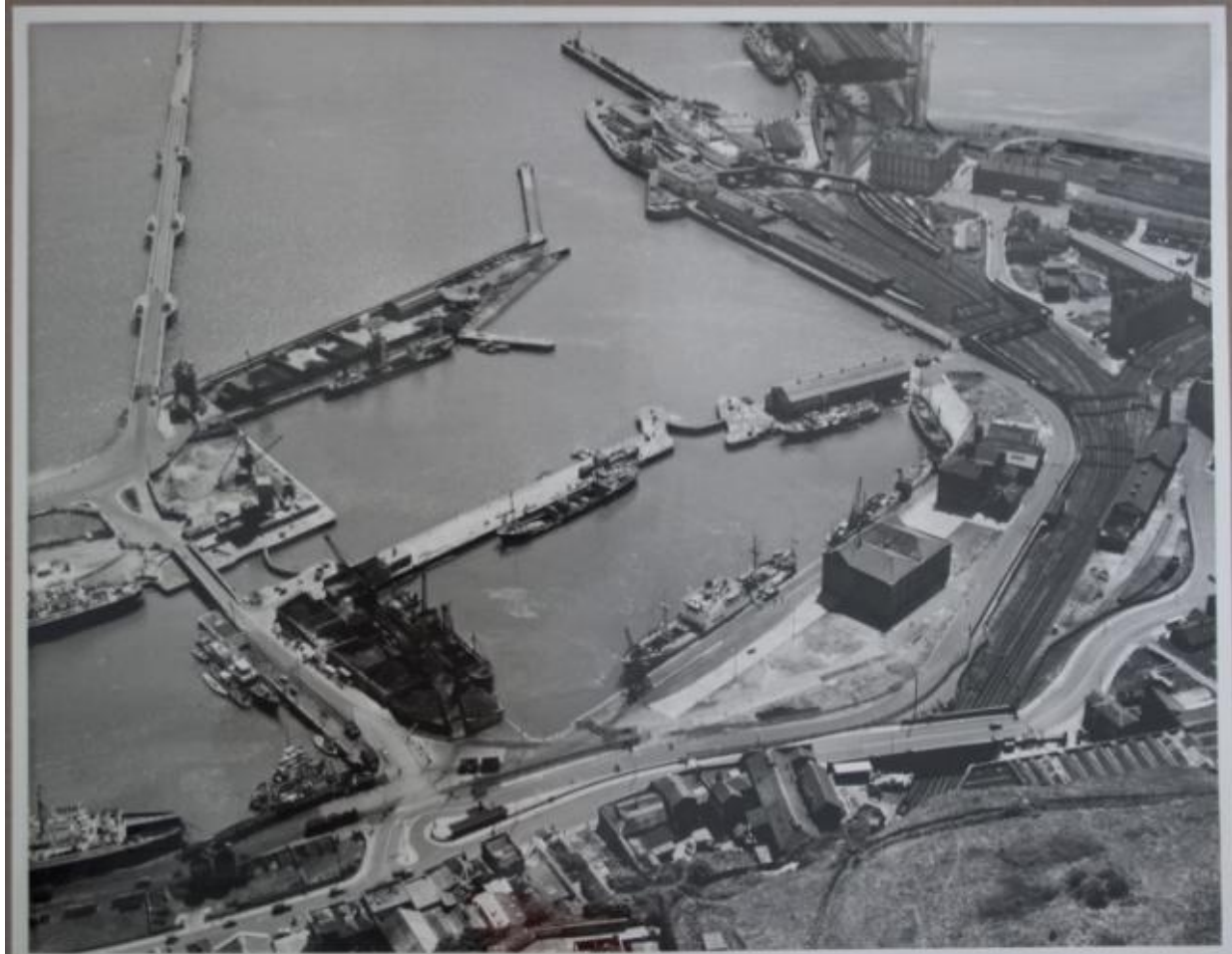
Plate 14: Aerial view overlooking the Western Dockyard, Union Street can be seen to the right of the image with the bridge and the gates visible. July 1956, DHB.
