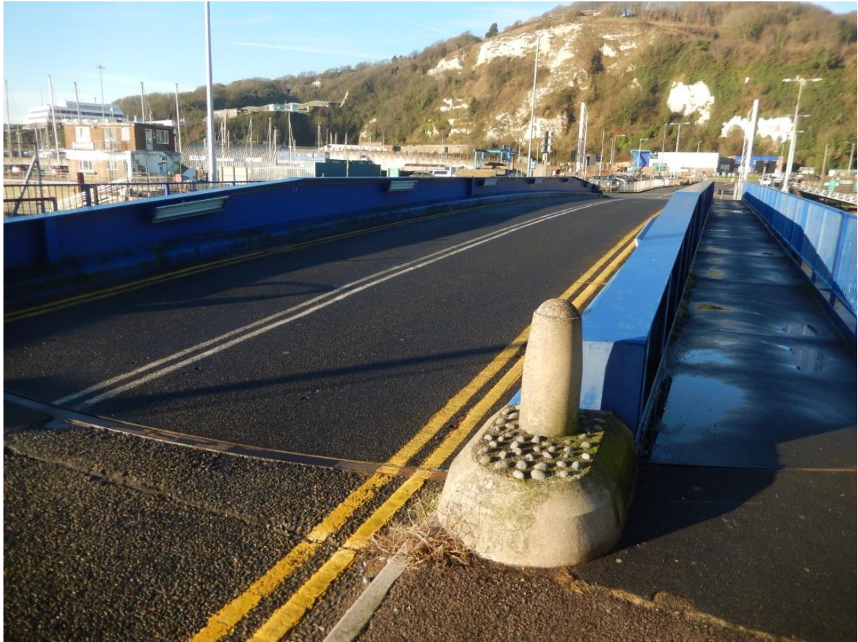
Plate 23: View looking west over the swing bridge, 25/01/2016, DHB.
