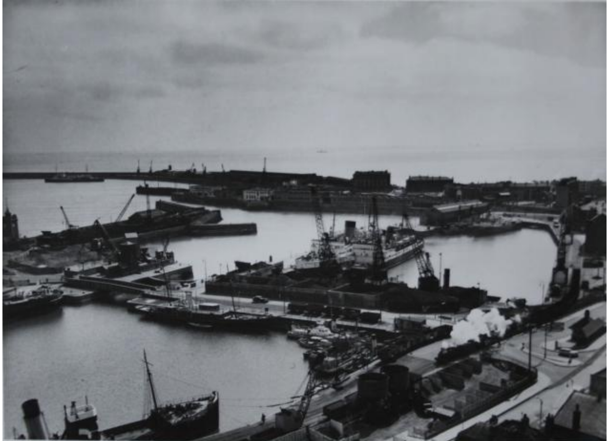
Plate 13: View looking towards the Admiralty Pier, south-east. Swing bridge can be seen in the foreground. 1955, DHB.
