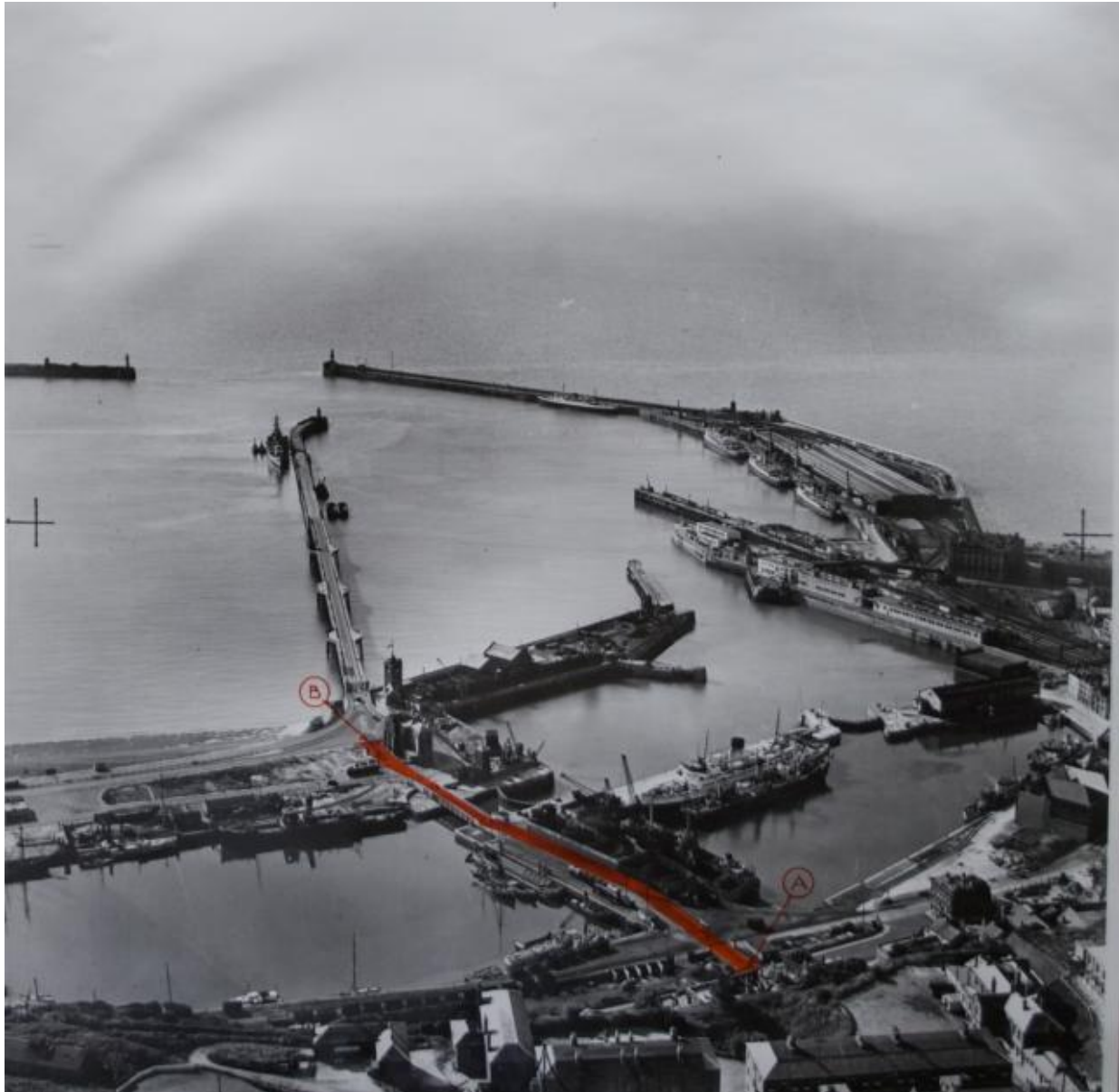
Plate 11: View of the Western Docks looking east towards the Prince of Wales Pier, Union Street has been highlighted in red, 1950, DHB.
