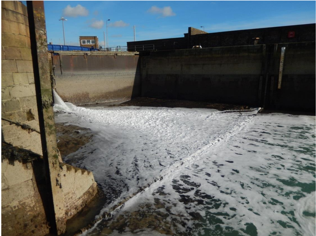
Plate 30: View of the back of the Wellington Dock Gates, looking north east, 25/01/2016, DHB.
