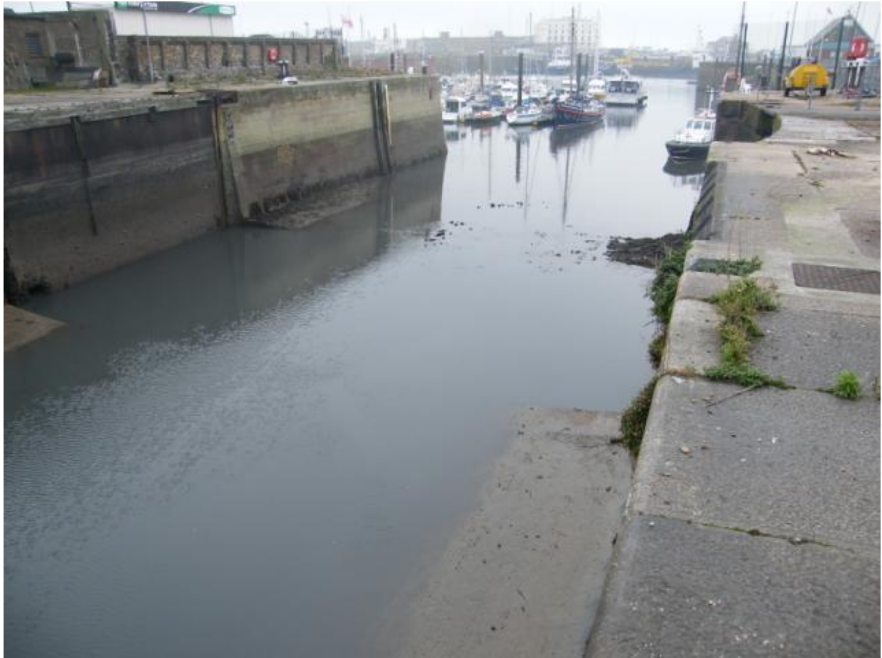
Plate 18: The location of the Wellington Dock Gates, with them removed for repair and the dock drained, looking South, 21/12/11, DHB.
