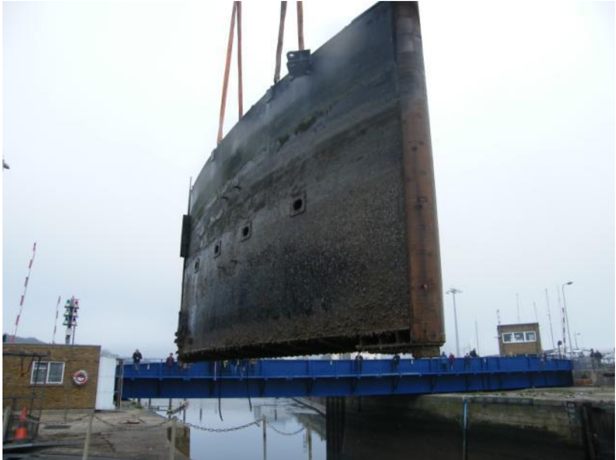
Plate 19: The dock gate being lifted from its position, looking North, 21/12/11, DHB.
