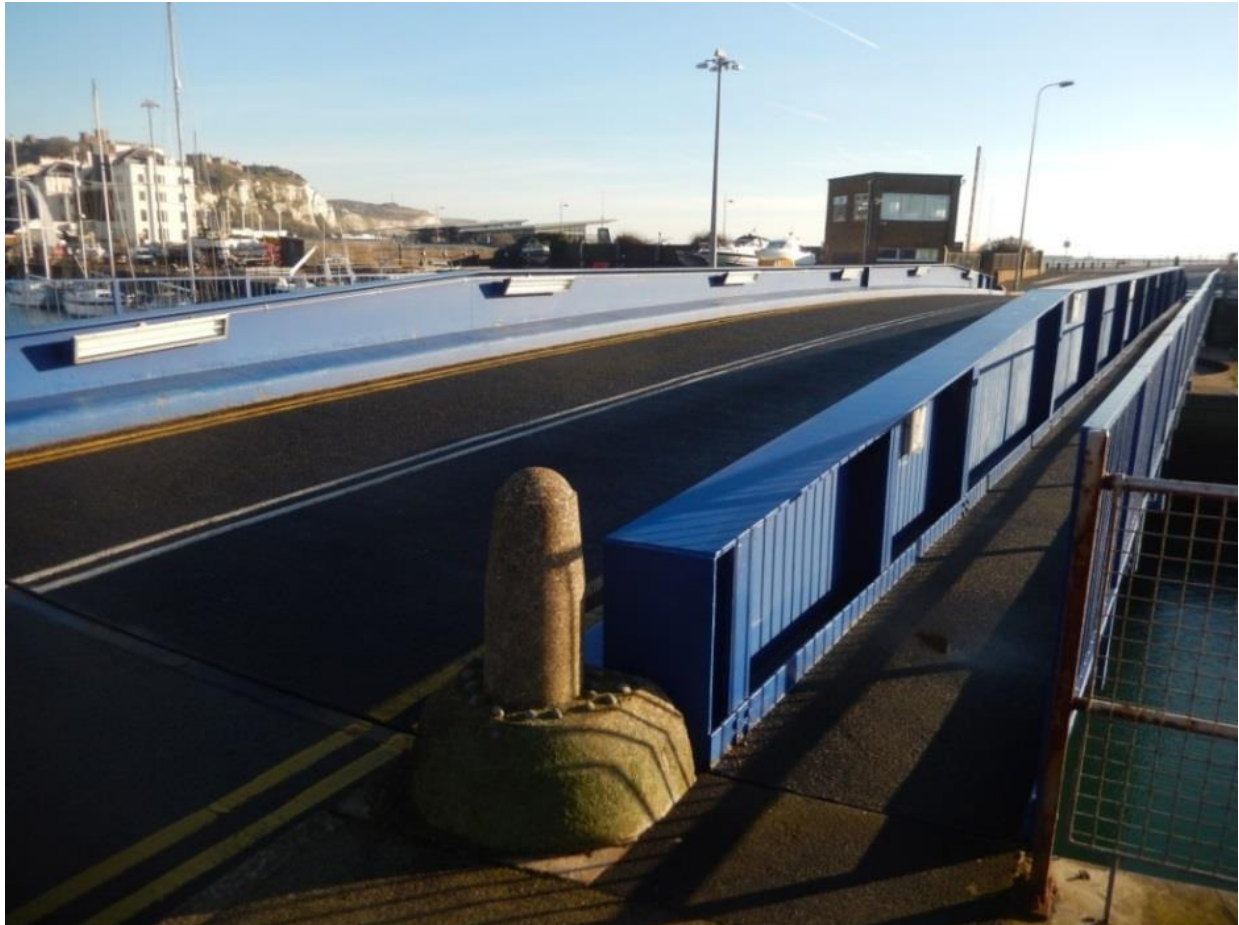
Plate 21: View looking east over the swing bridge, 25/01/2016 , DHB.
