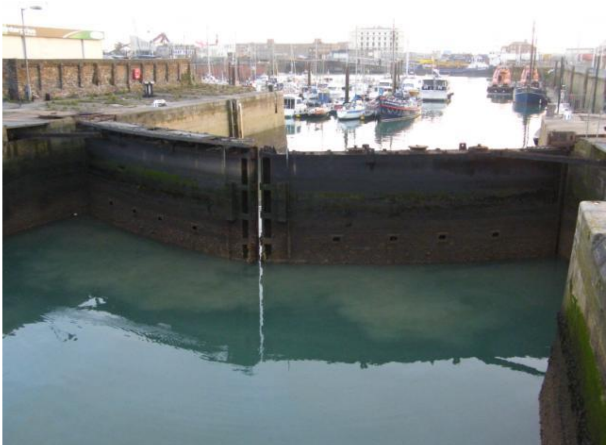
Plate 20: The Wellington Dock Gates in an closed position, looking South, 10/10/11, DHB.
