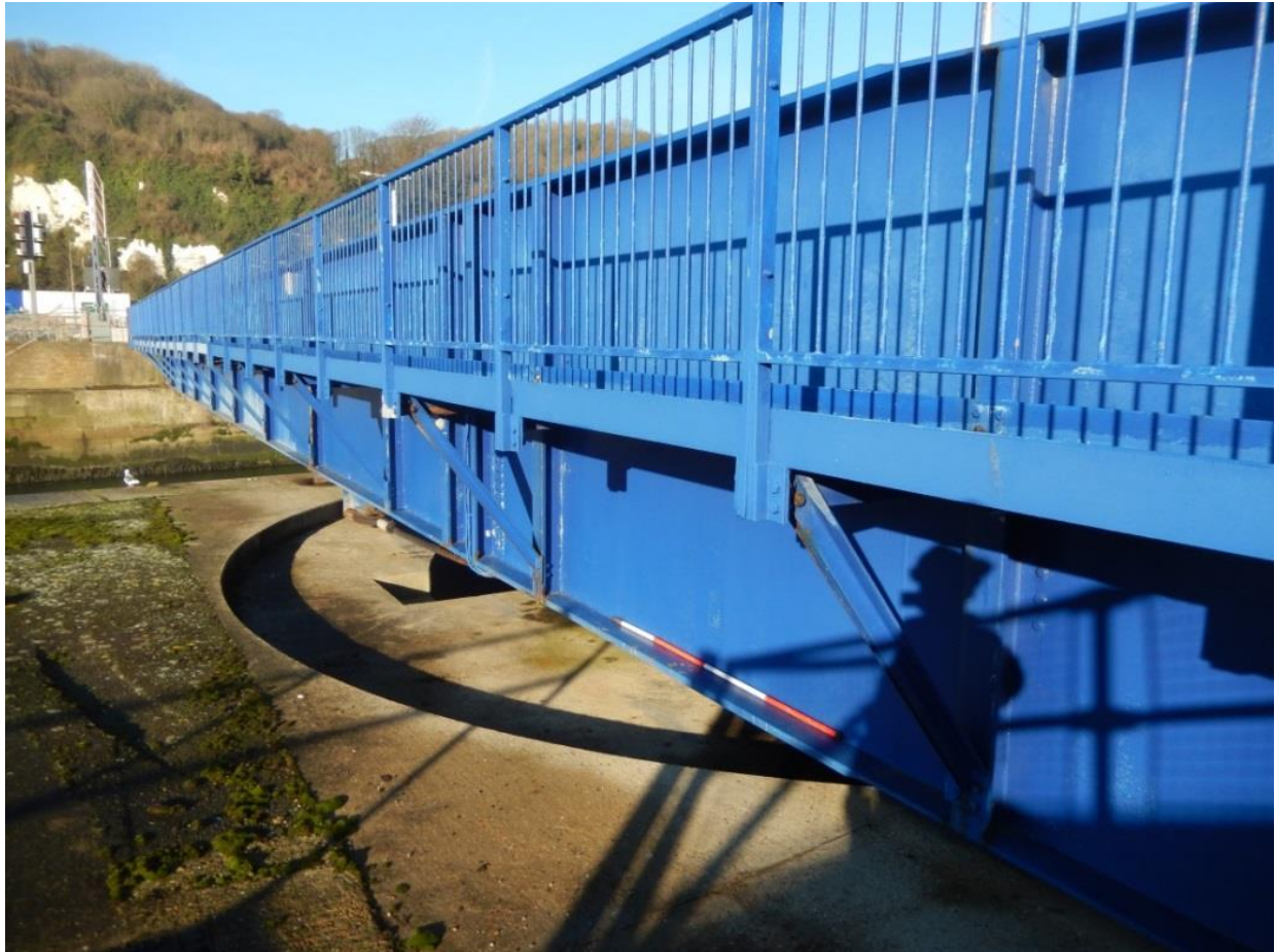
Plate 24: Image of the south side of the bridge, showing the walkway, 25/01/2016, DHB.
