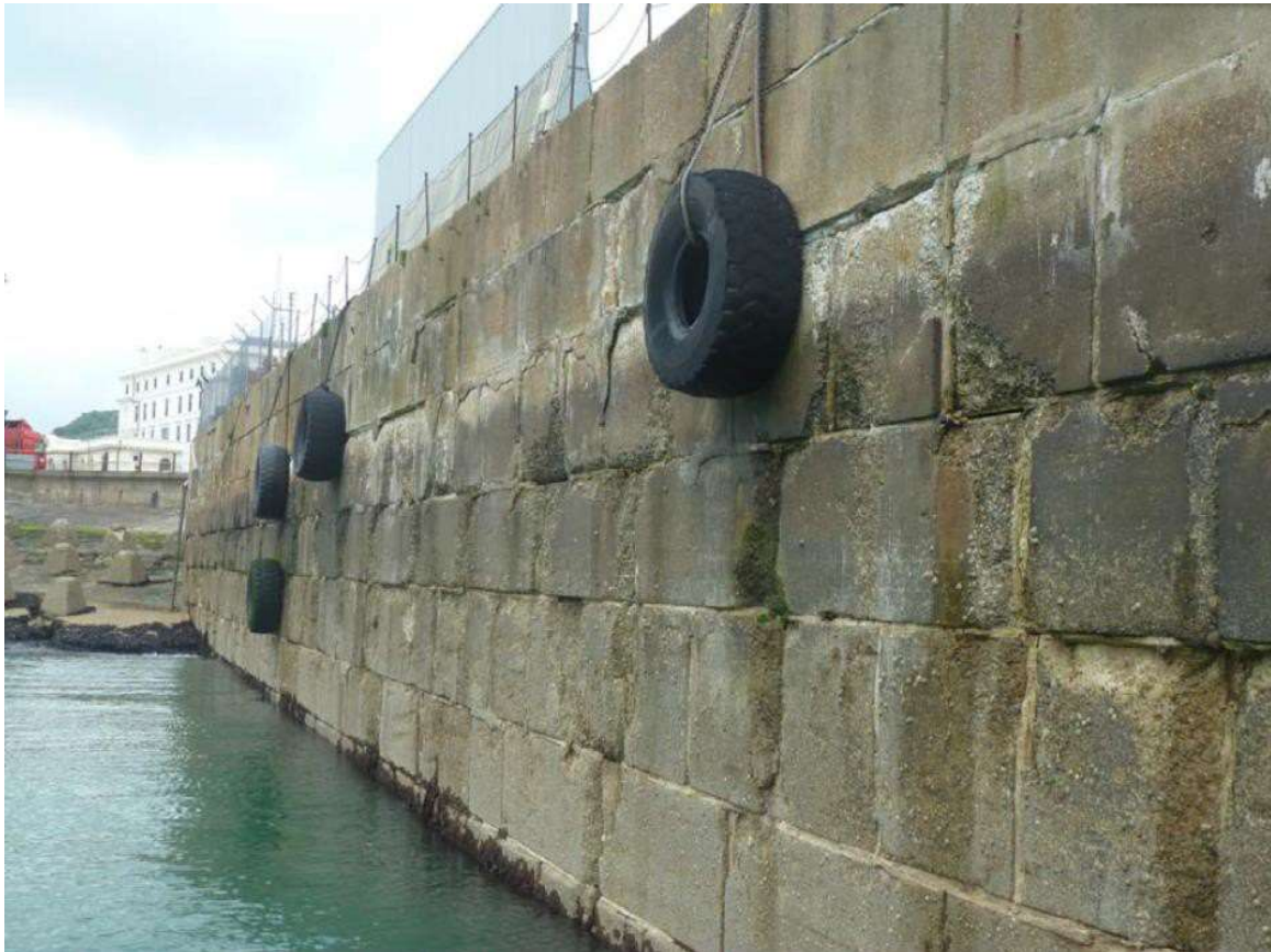
Plate 29: South site, external vertical wall of the Train Ferry Dock with 'wavebreaker toe' to the rear, looking west, 2014, Atkins 2014b: 3.
