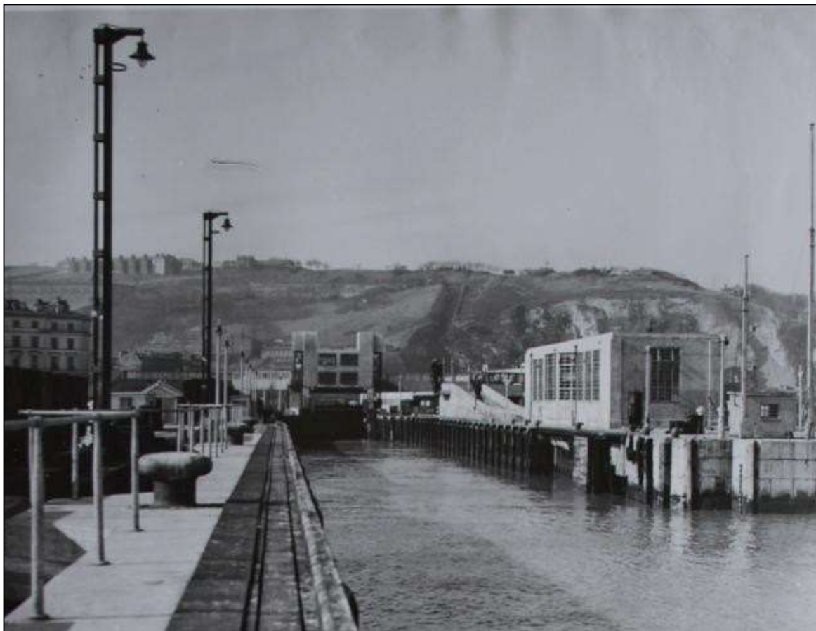
Plate 5: Western Dock: View of the Train Ferry Berth with the Berth Gates Open at High Tide 01/03/1938, DHB.
