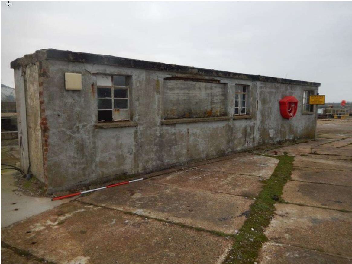
Plate 22: Building at landward end of jetty 25/01/2016, DHB 2016a: 160.
