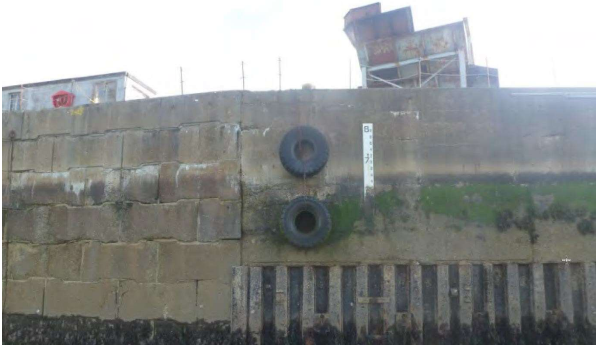
Plate 25: Change in construction at landward end of jetty (southern side), 2014, Atkins 2014a: 27.
