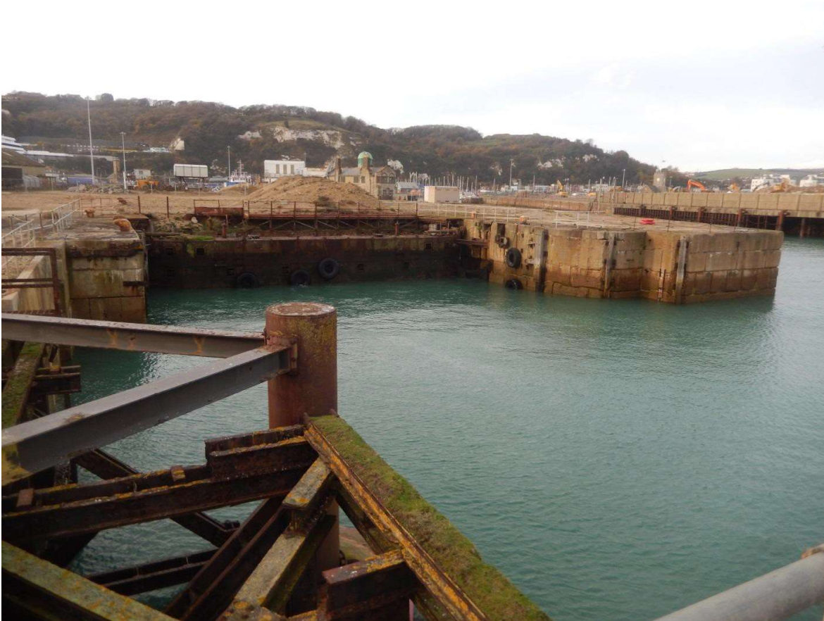
Plate 38: View of Train Ferry Dock Gates from Dunkirk Jetty, looking west, 16/11/2016, DHB.
