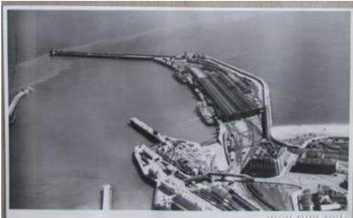
Plate 11: General View of the Admiralty Pier, Marine Station and the Train Ferry Berth, 1950, DHB.
