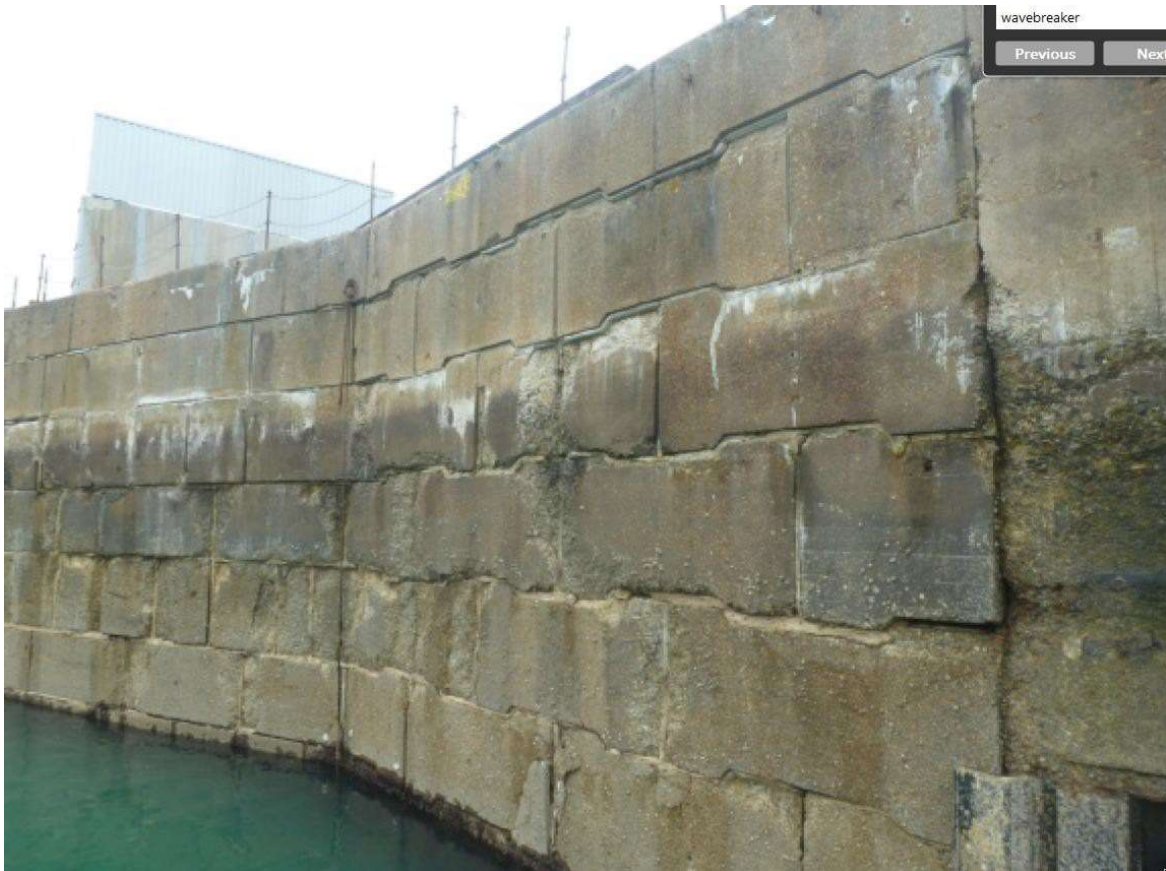
Plate 30: South site, external vertical wall of the Train Ferry Dock at change in orientation and change from keyed to plain blocks, 2014, Atkins 2014b: 16.
