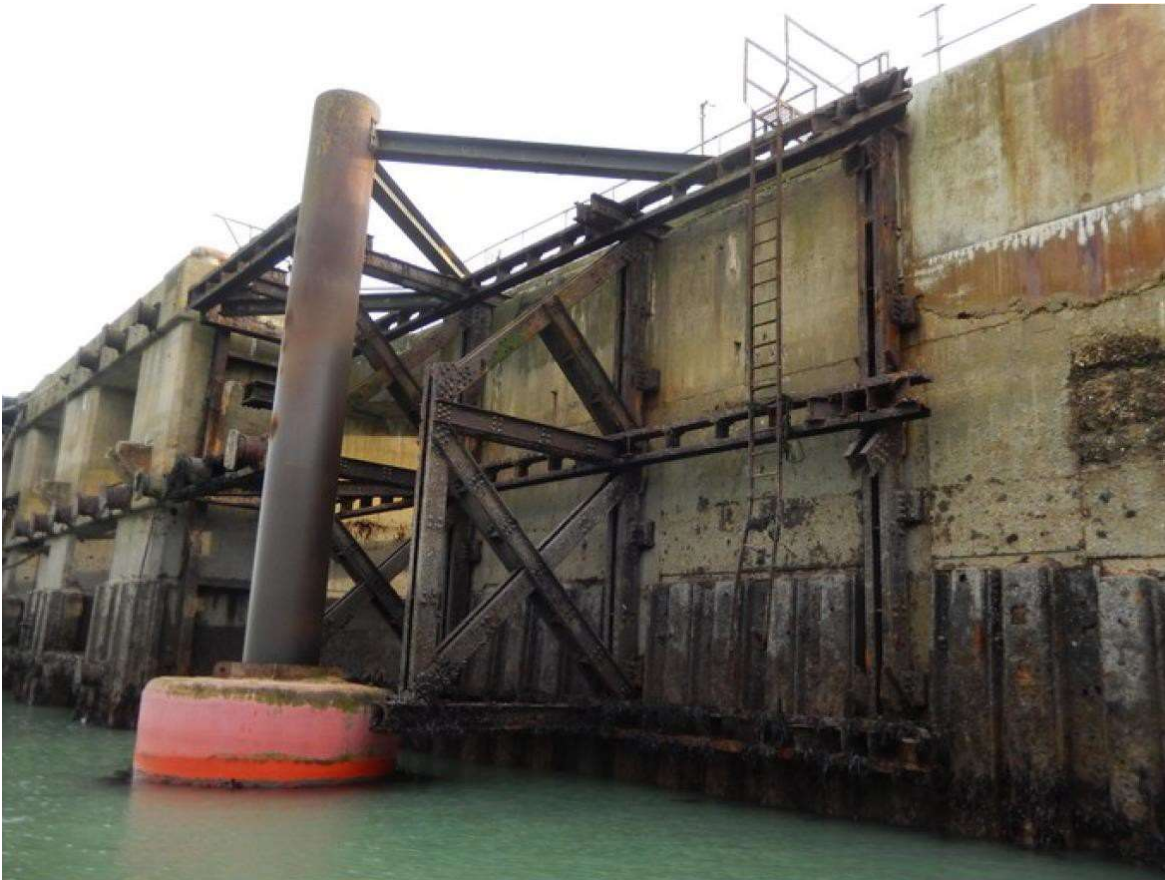
Plate 26: Ladder and partially removed steel framework 23/11/15, DHB 2016a: 3.
