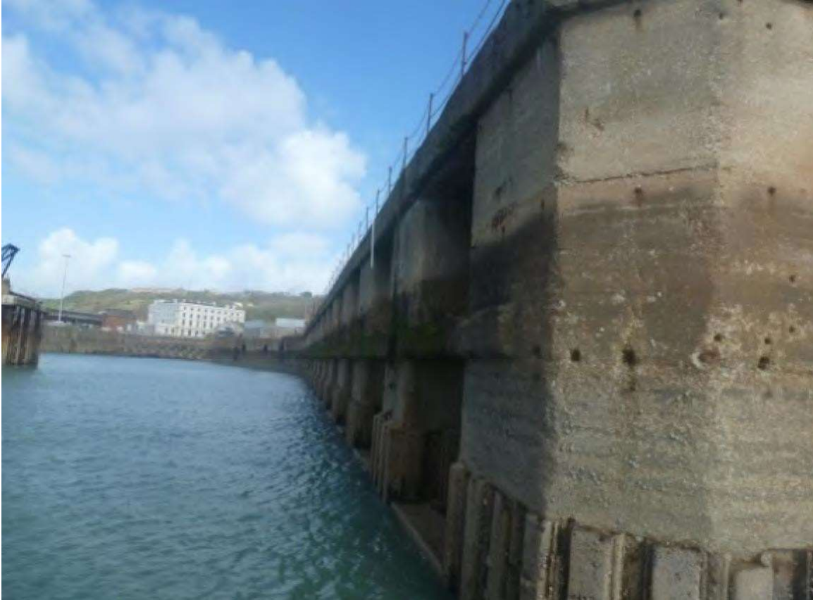
Plate 28: Southern side of the jetty, looking west, 2014, Atkins 2014a: 22.
