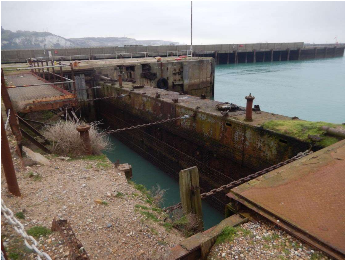
Plate 34: Detail of Train Ferry Dock Gates, looking east, 25/01/2016, DHB 2016a: 200.
