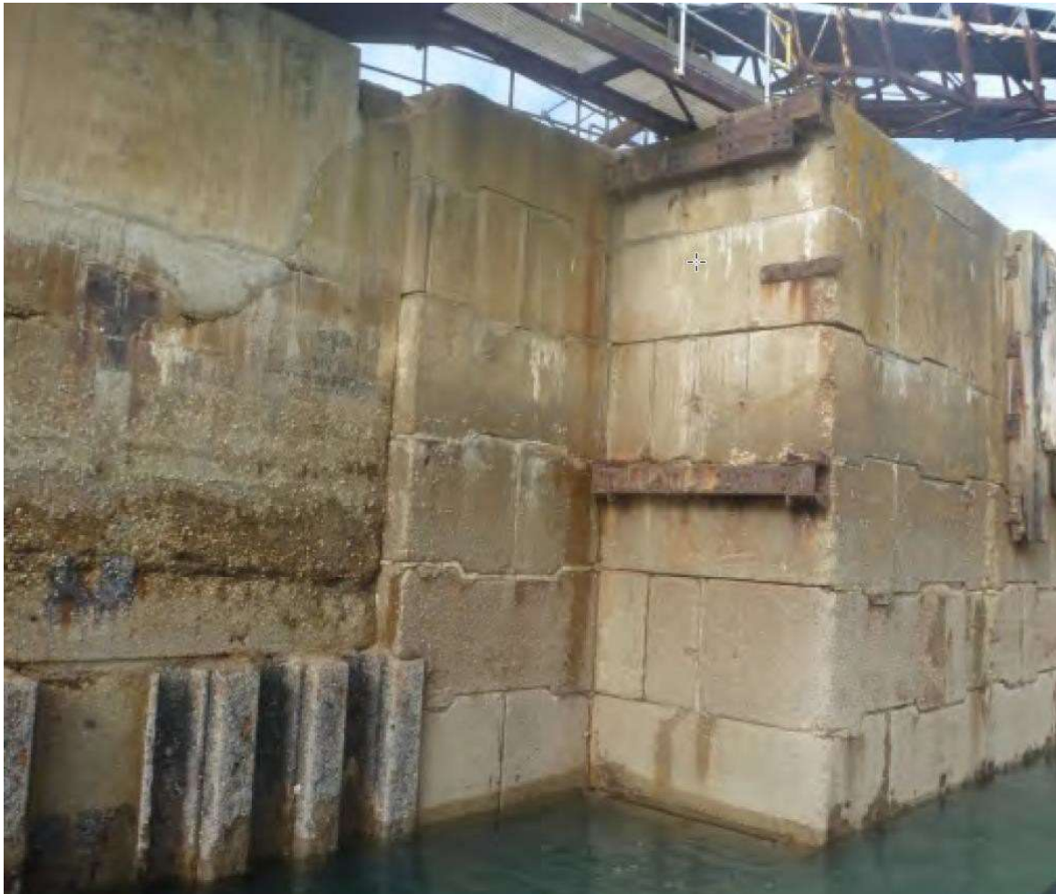
Plate 24: Change in construction at landward end of jetty (northern side), 2014, Atkins 2014a: 17.
