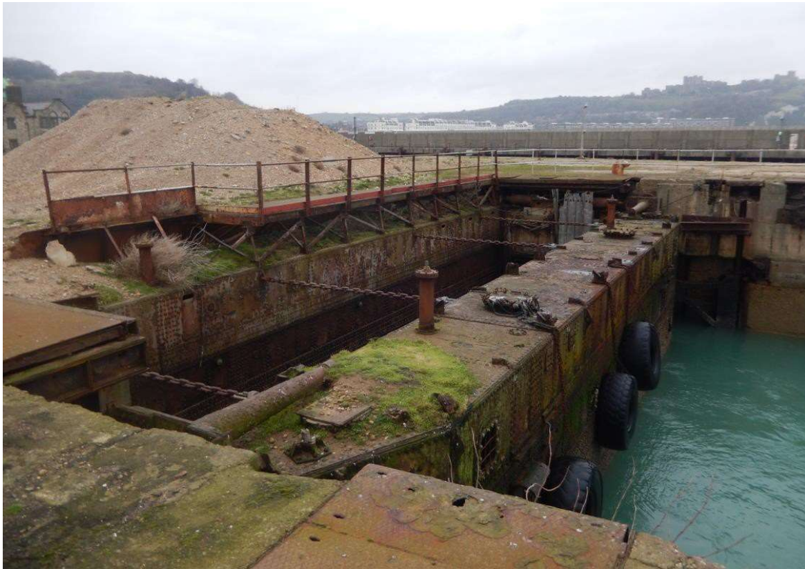
Plate 33: Detail of Train Ferry Dock Gates, looking north, 25/01/2016, DHB 2016a: 198.
