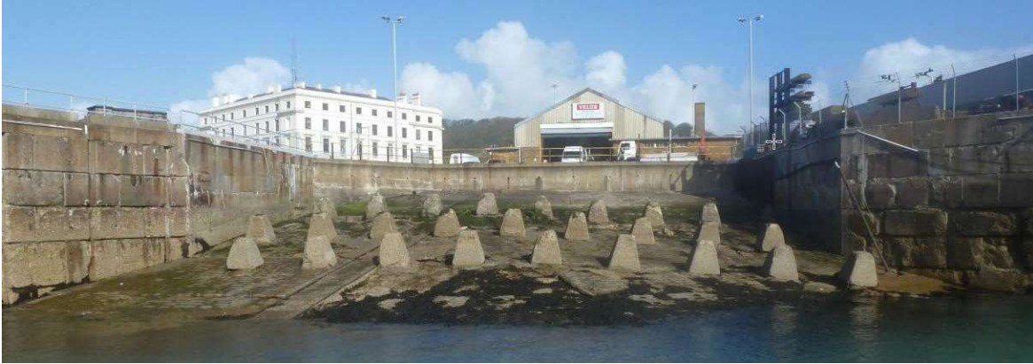
Plate 31: Wavebreaker Toe concrete slipway, with wave breaker units or anti-tank 'pimples', 2014, Atkins 2014b: 21.
