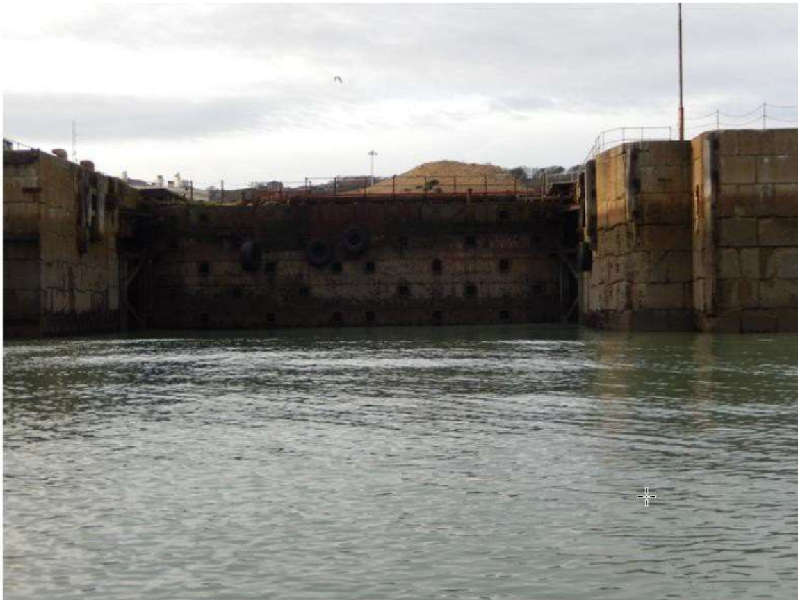
Plate 36: Train Ferry Dock Gates, looking west, 23/11/2015, DHB 2016b: 75.
