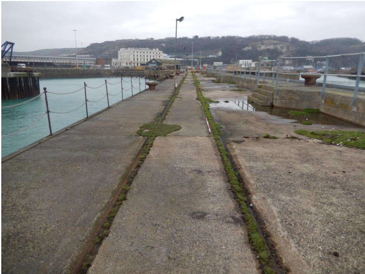
Plate 20: Dunkirk Jetty looking west, 25/01/2016, DHB 2016a: 66.
