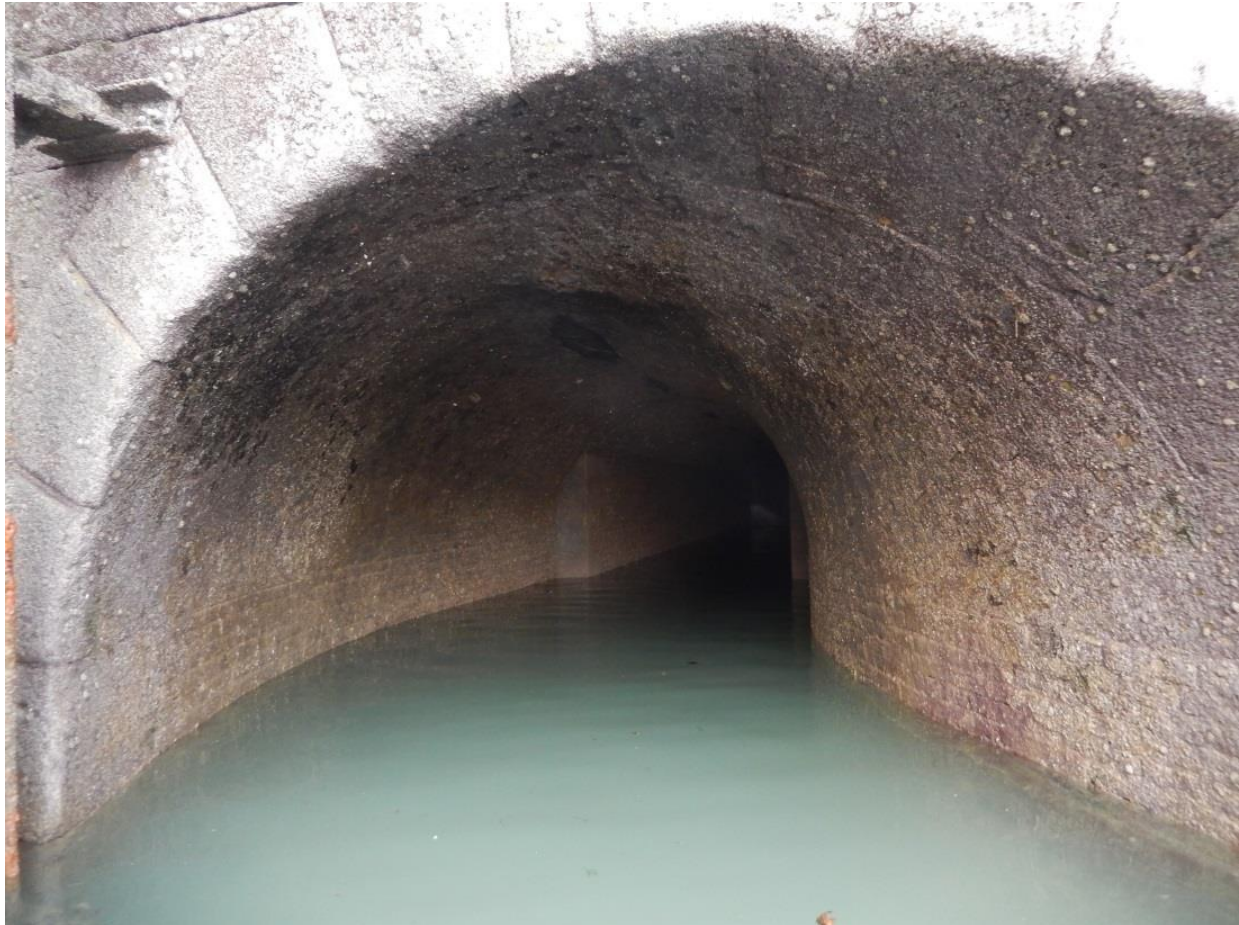
Plate 16: A look inside the culvert that is associated with Sluice A, which would have controlled the water within The Wellington Dock, looking North, DHB.
