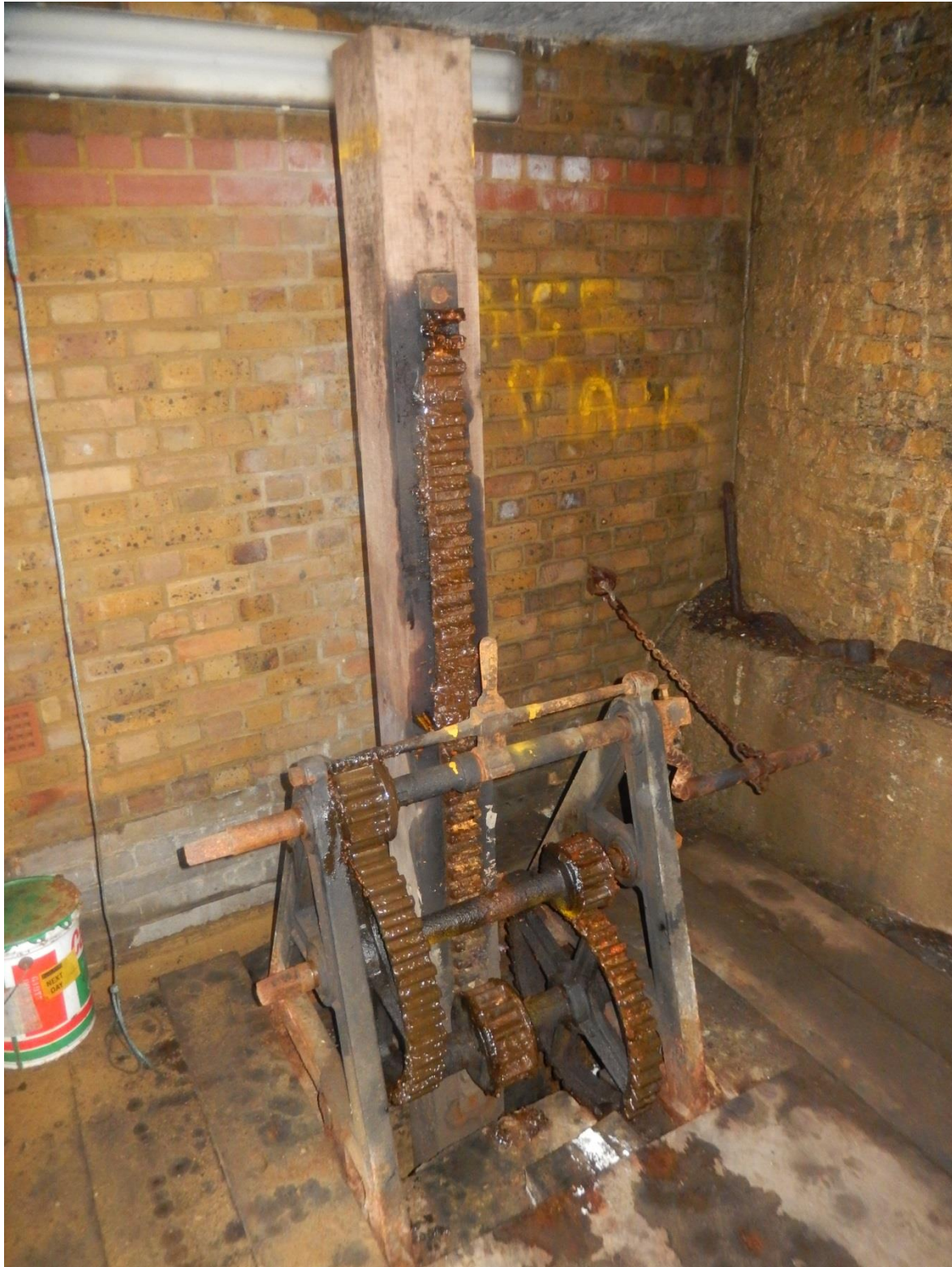
Plate 19: One half of the two mechanisms that form sluice B, DHB.
