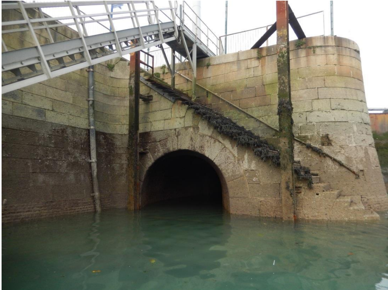
Plate 15: The culvert that operated with the mechanisms of Sluice A, controlling the water within the Wellington Dock, dating to 1845, looking North, DHB.
