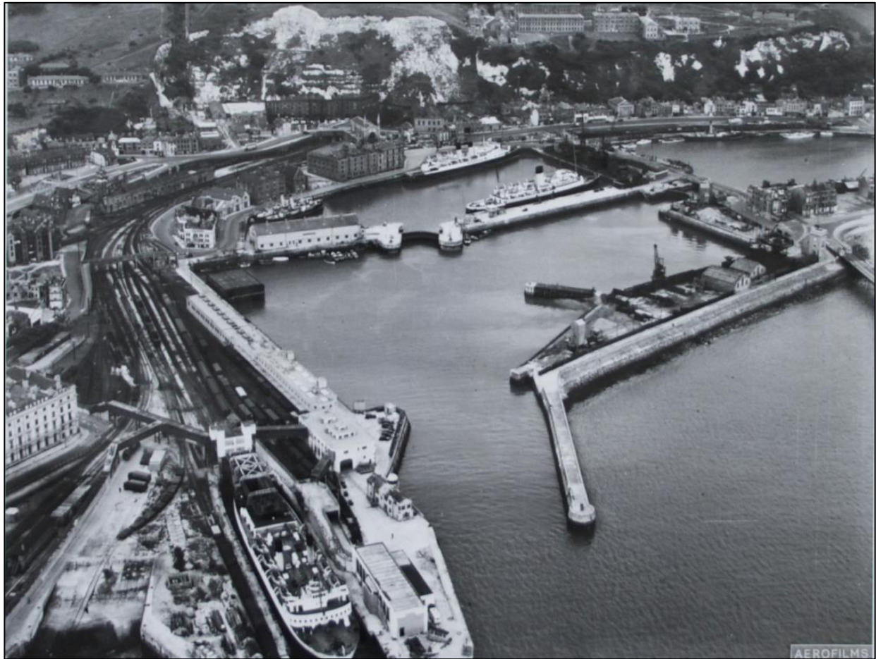
Plate 10: Entrance to Western Docks, View of the Train Ferry Dock, Tidal Basin Entrance, The Granville and Waterloo Dock, 1950, DHB.
