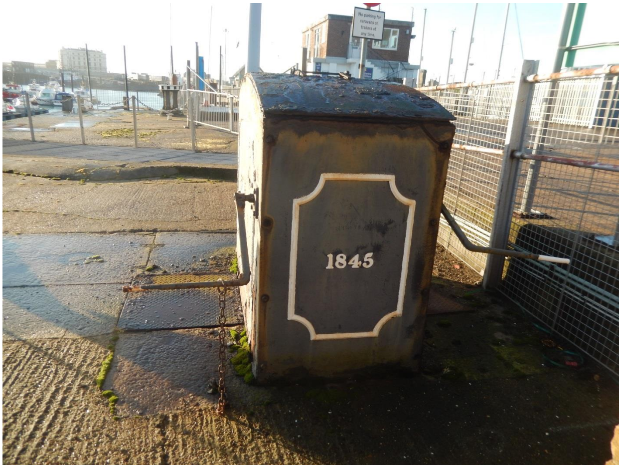
Plate 13: Back view of sluice A with visible crank mechanisms, looking North, DHB.
