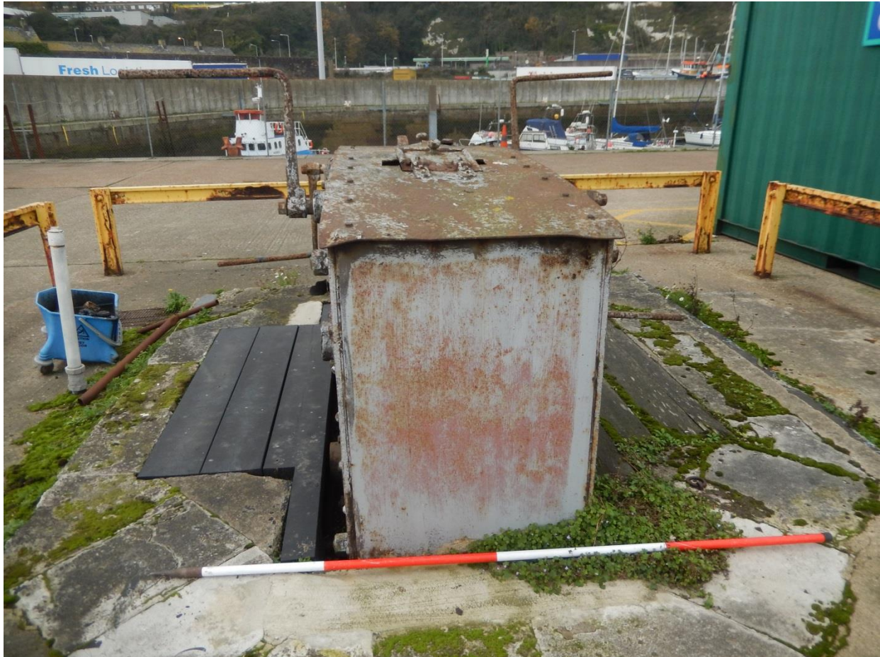
Plate 27: Sluice C positioned on the Crosswall, 2016, Scale 2m, looking West, DHB.
