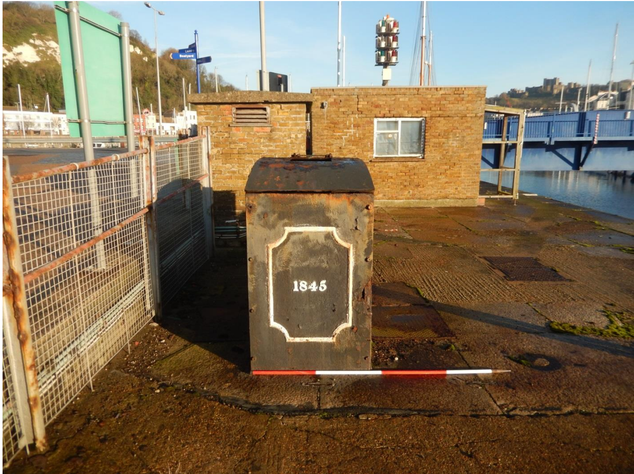
Plate 12: Front view of sluice A showing date of 1845, looking North, 2m Scale, DHB.
