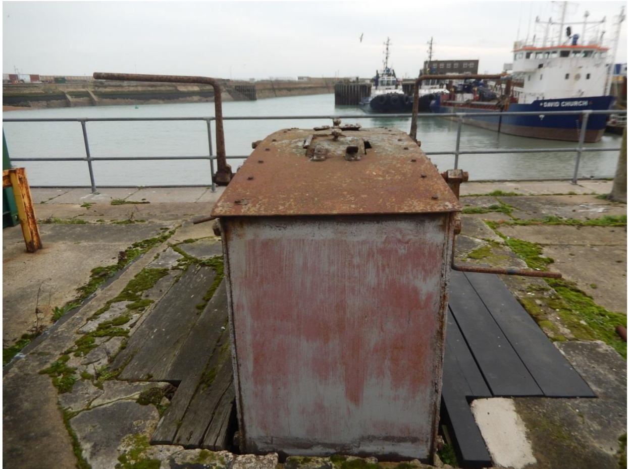
Plate 29: Sluice C positioned on the Crosswall, 2016, looking East, DHB.
