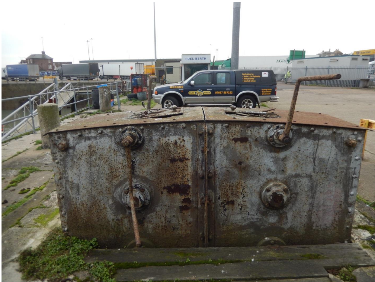
Plate 28: Sluice C positioned on the Crosswall, 2016, Scale 2m, looking South, DHB.
