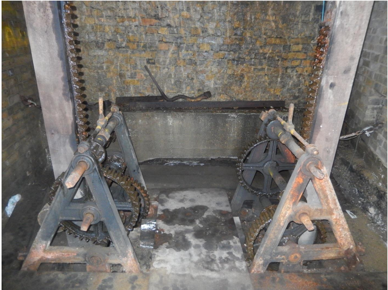
Plate 18: The two mechanisms which form sluice B, DHB.
