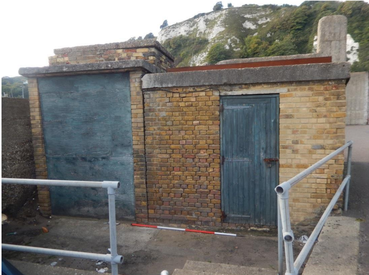
Plate 17: The small brick building which holds sluice B, looking West, 2m Scale, DHB.
