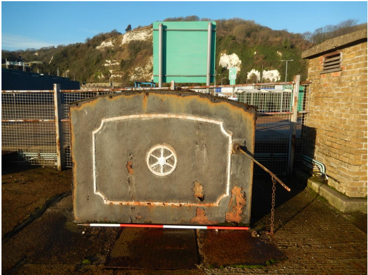
Plate 11: Side view of sluice A with crank mechanisms to the right, looking West, 2m Scale, DHB.
