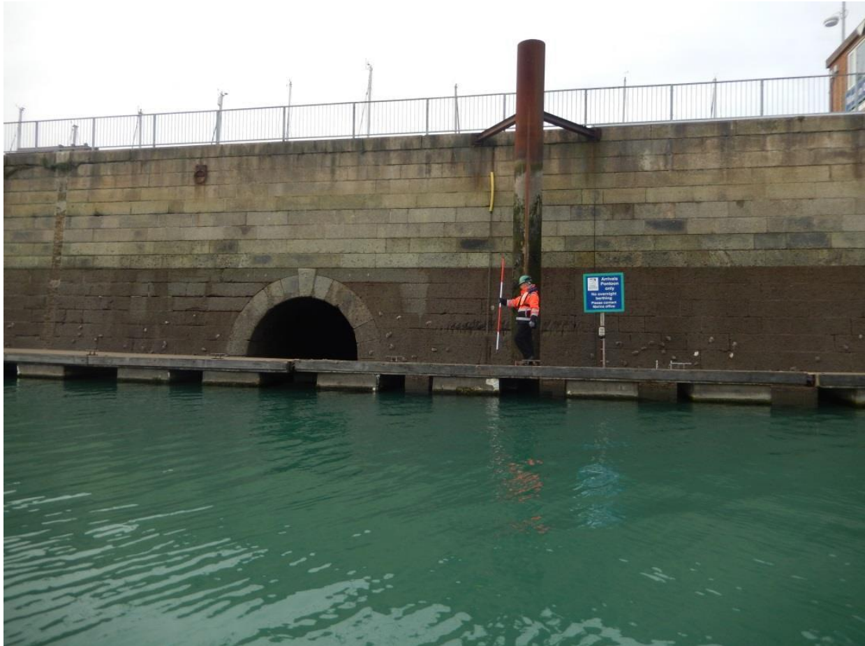
Plate 31: The culvert present on The Crosswall, no longer in use or attached to sluice mechanism, 2016, looking north-east, DHB.
