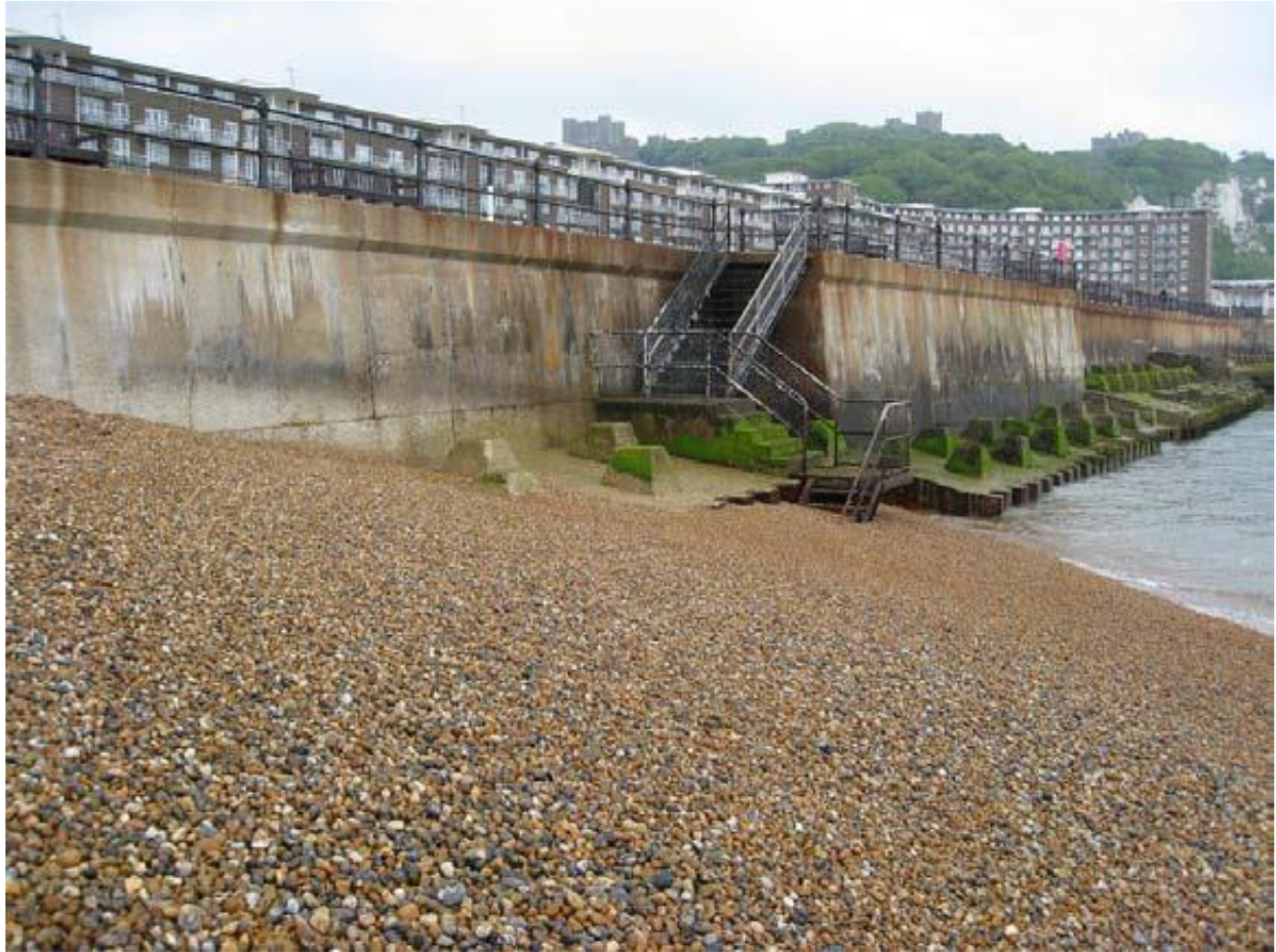
Plate 60: Looking down onto the dragons teeth which were installed into concrete, 2013, Atkins 2014, 25.
