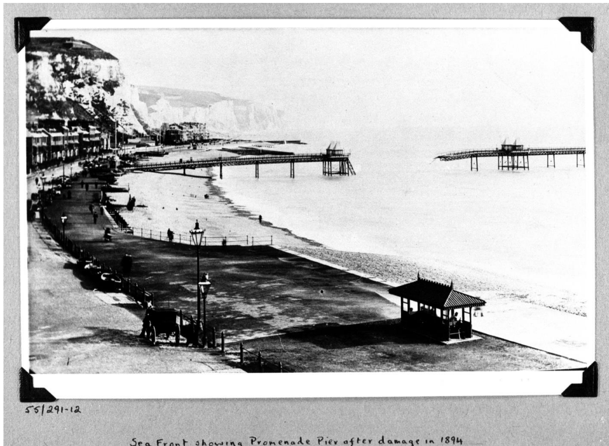
Plate 2: The Pleasure Pier after it had suffered damage by storm, c.1894, looking North, Dover Museum d22111.
