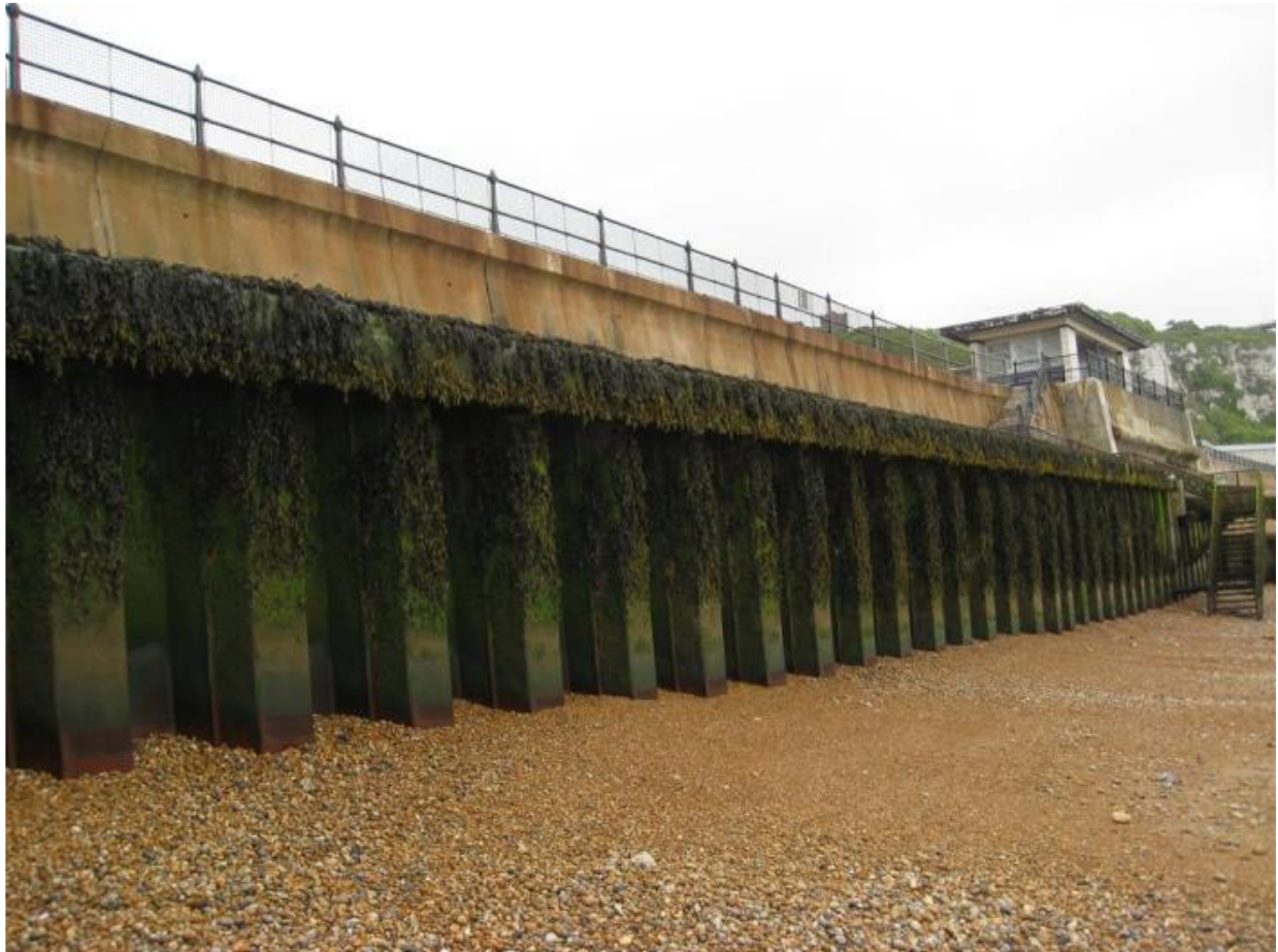
Plate 58: Steel sheeting covers the sea wall, looking towards the direction of the Eastern Docks, 2013, looking north-west, Atkins 2014, 24.
