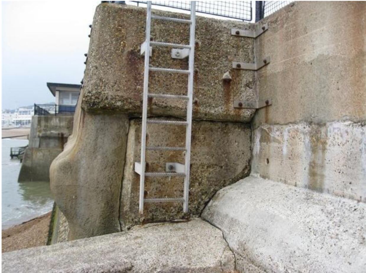
Plate 56: A ladder providing access to the beach covering different additions of the seawall, 2013, looking South, Atkins 2014, 21.
