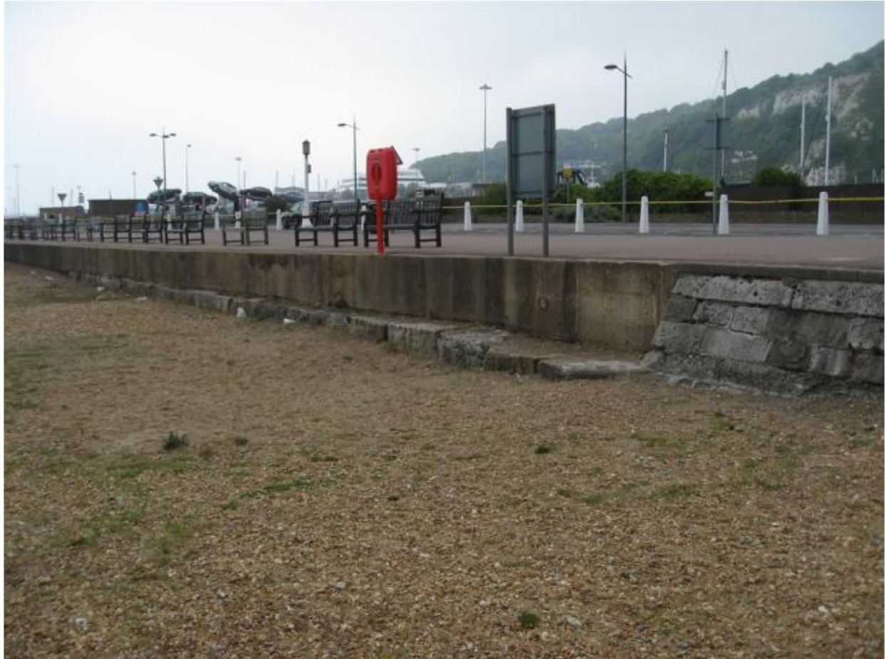
Plate 65: A much older section of wall opposite the sea sports centre and outside Harbour House, looking south-west, 2013, Atkins 2014, 32.
