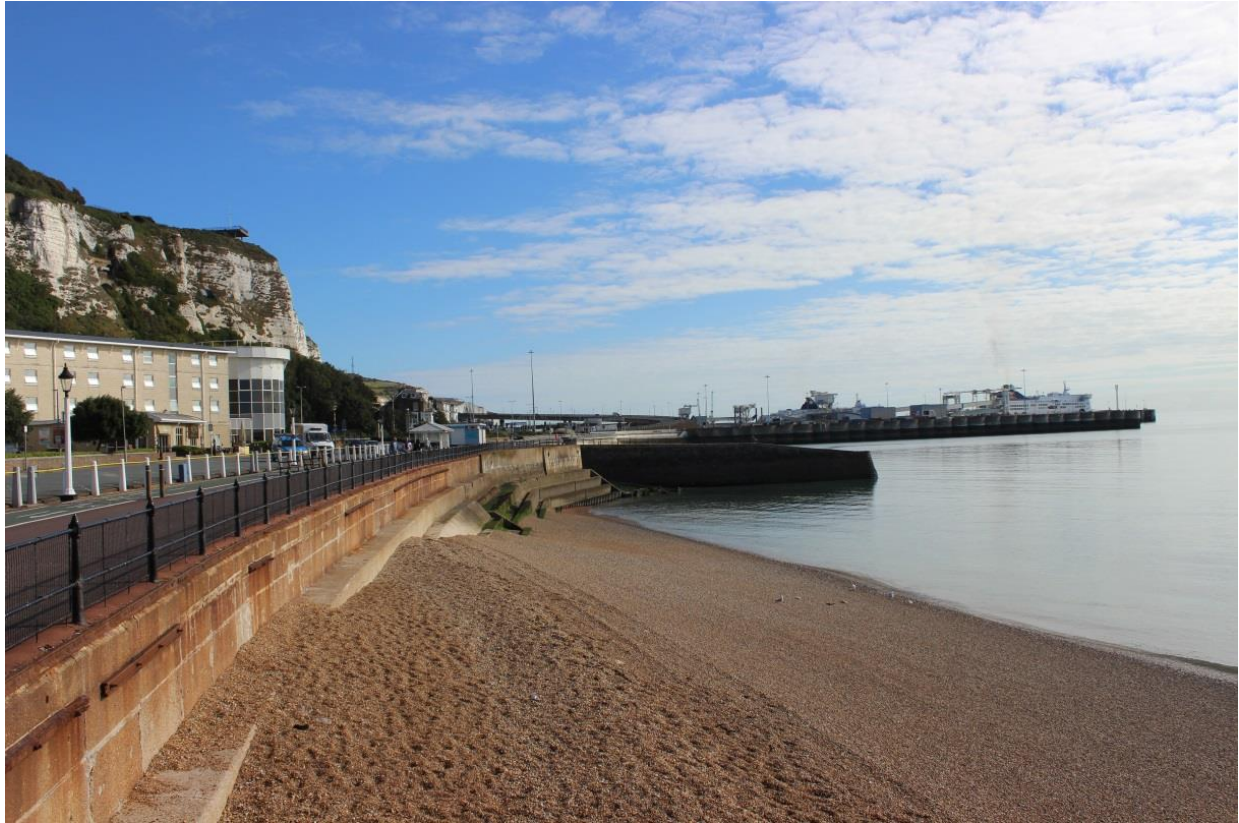
Plate 44: The Eastern Docks can be seen in the background with the Premier in to the left of the image, 23/09/2016, looking north-east, DHB.
