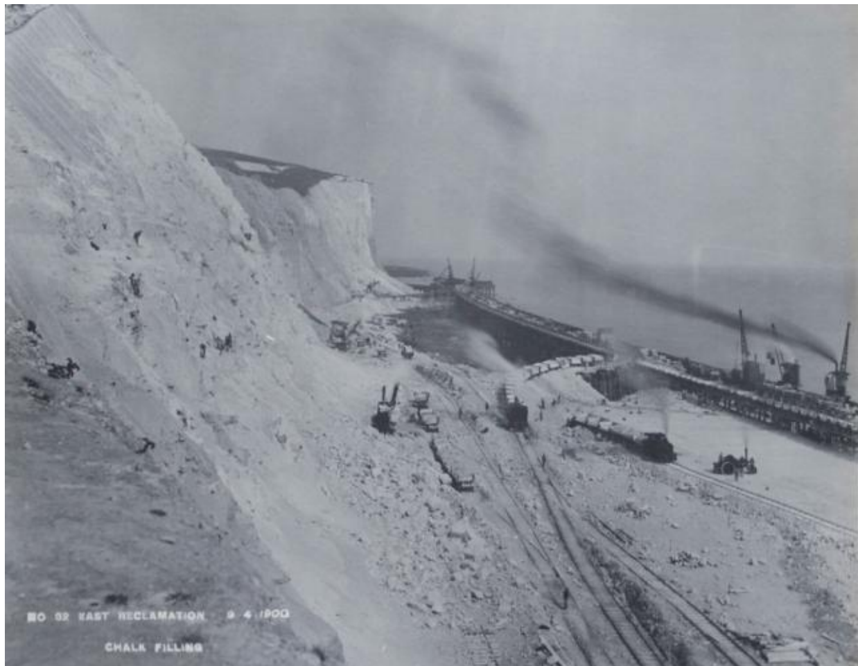
Plate 7: The land that would be reclaimed to become the Eastern side of the Dockyard, 09/04/1900, looking North, DHB.
