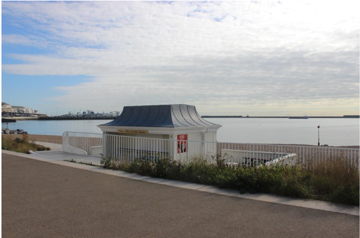
Plate 38: One of two kiosks positioned along The Promenade, 23/09/2016, looking north-east, DHB.
