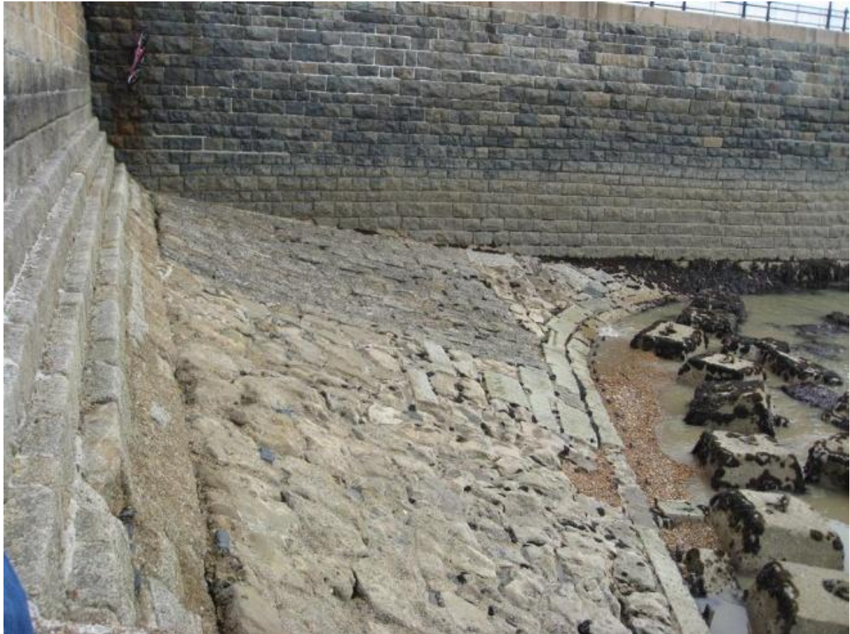
Plate 52: Sloping blockwork revetment, the seawall can be seen on the left, 2013, looking North, Atkins 2014, 15.
