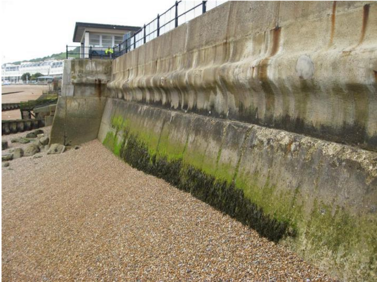
Plate 57: Looking along to seawall towards the direction of Waterloo Crescent, 2013, looking South, Atkins 2014, 22.
