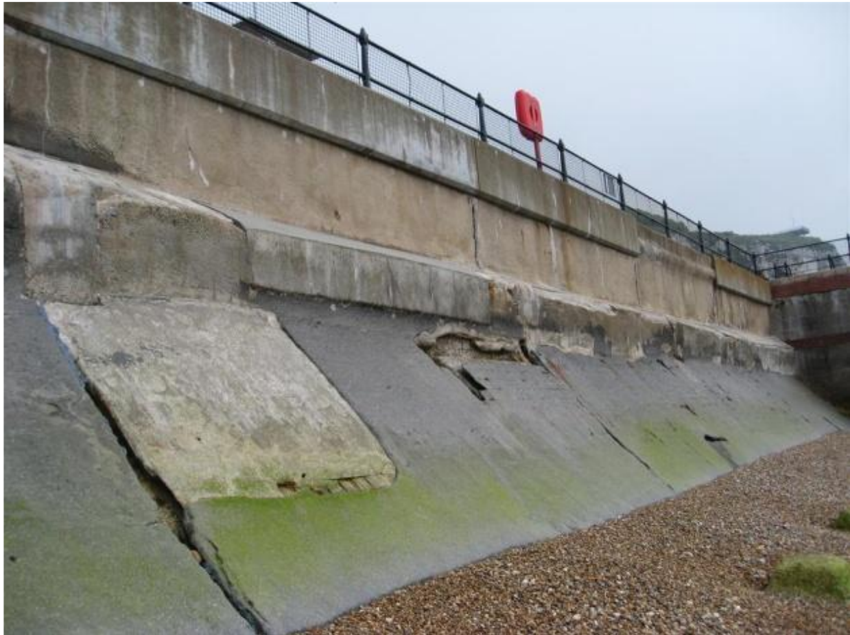
Plate 55: A section of the sea wall, 2013, looking North, Atkins 2014, 20.
