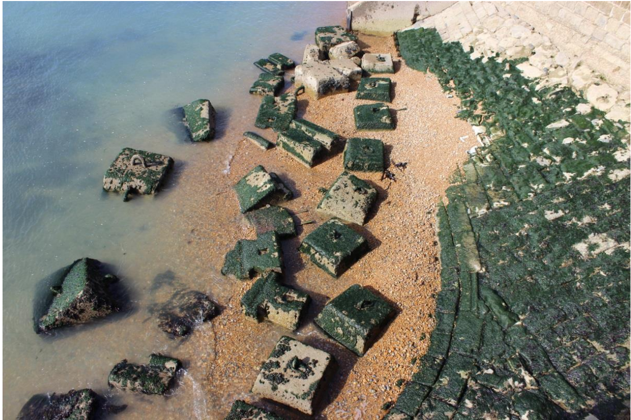
Plate 47: Detail of a collection of stones used as defences- date installed unknown, 23/09/2016, looking north-east, DHB.
