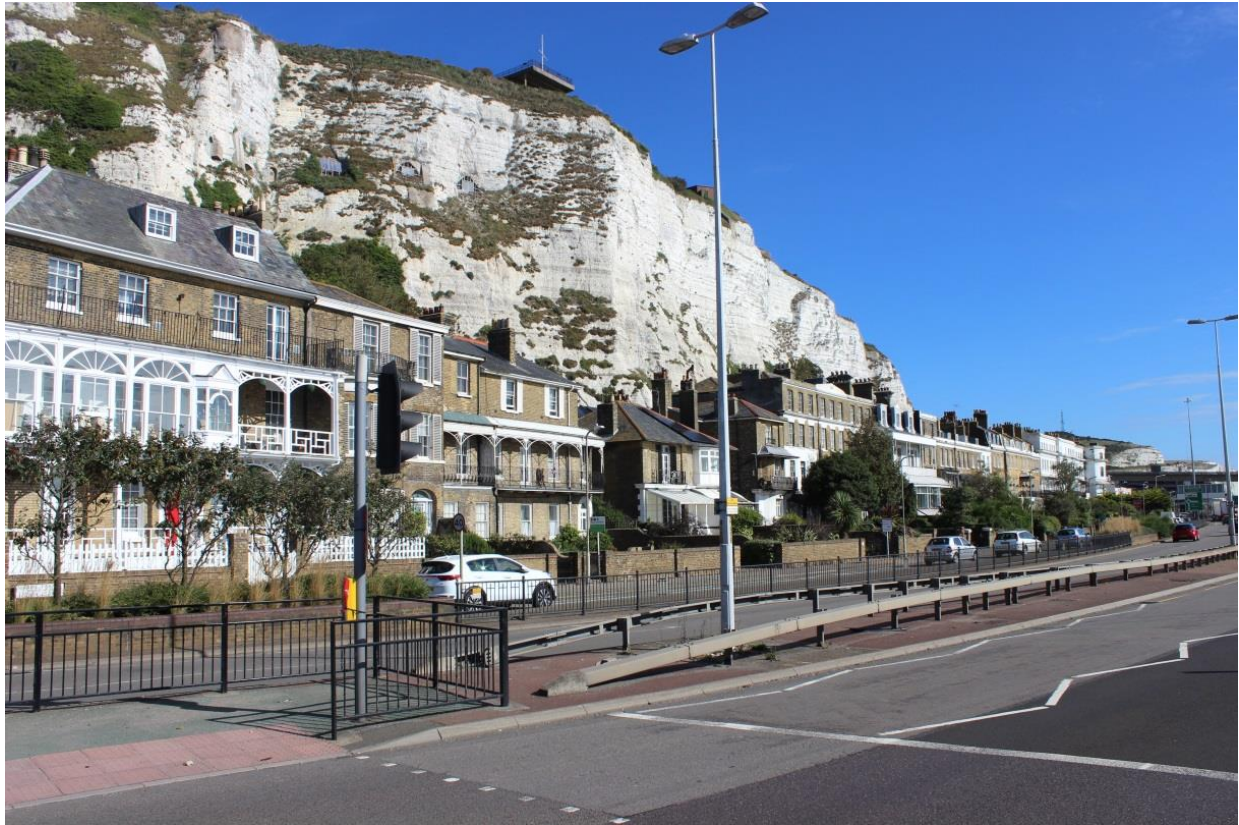
Plate 50: The base of the White Cliffs and the start of East Cliff Terrace, 23/09/2016, looking north-west, DHB.
