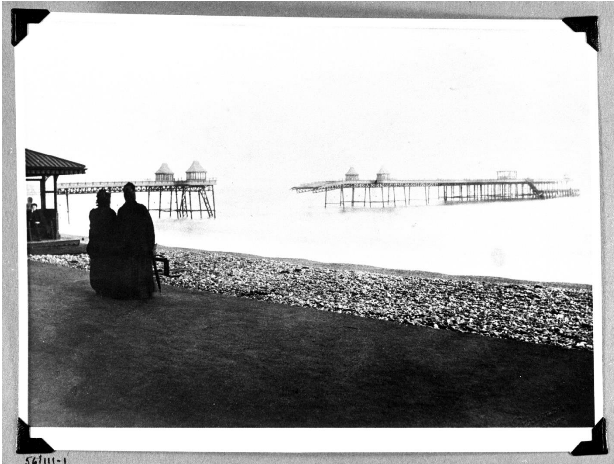
Plate 1: The Pleasure Pier after it had suffered damage by a storm, c.1894, looking north-east, DHB.
