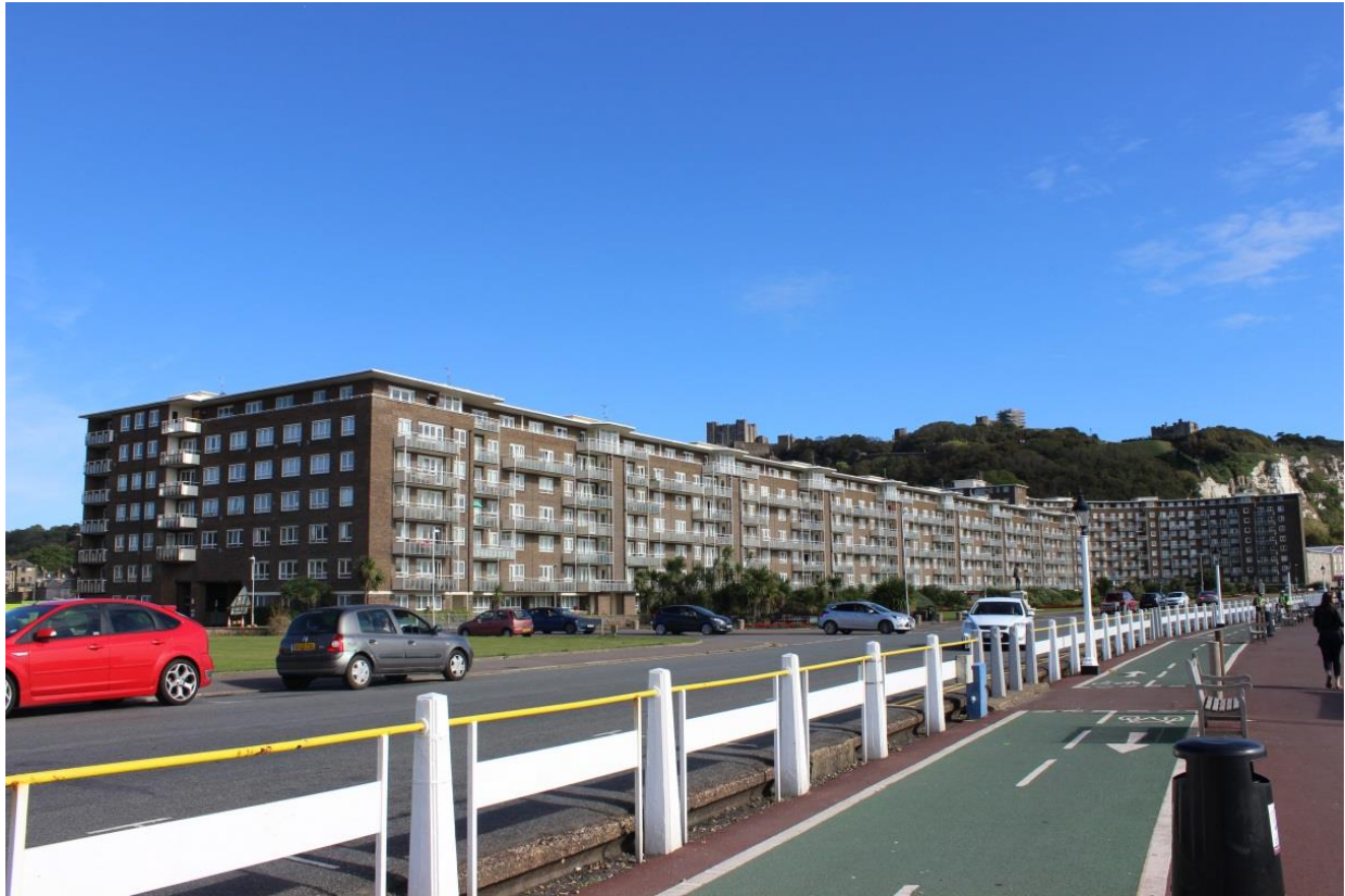
Plate 40: The Gateway Flats with the castle and cliffs in the background, 23/09/2016, looking North, DHB.
