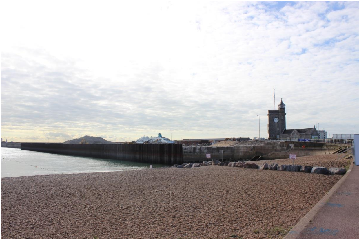
Plate 32: The Prince of Wales Pier and Clock House whilst construction works for the redevelopment are taking place, 23/09/2016, looking South, DHB.
