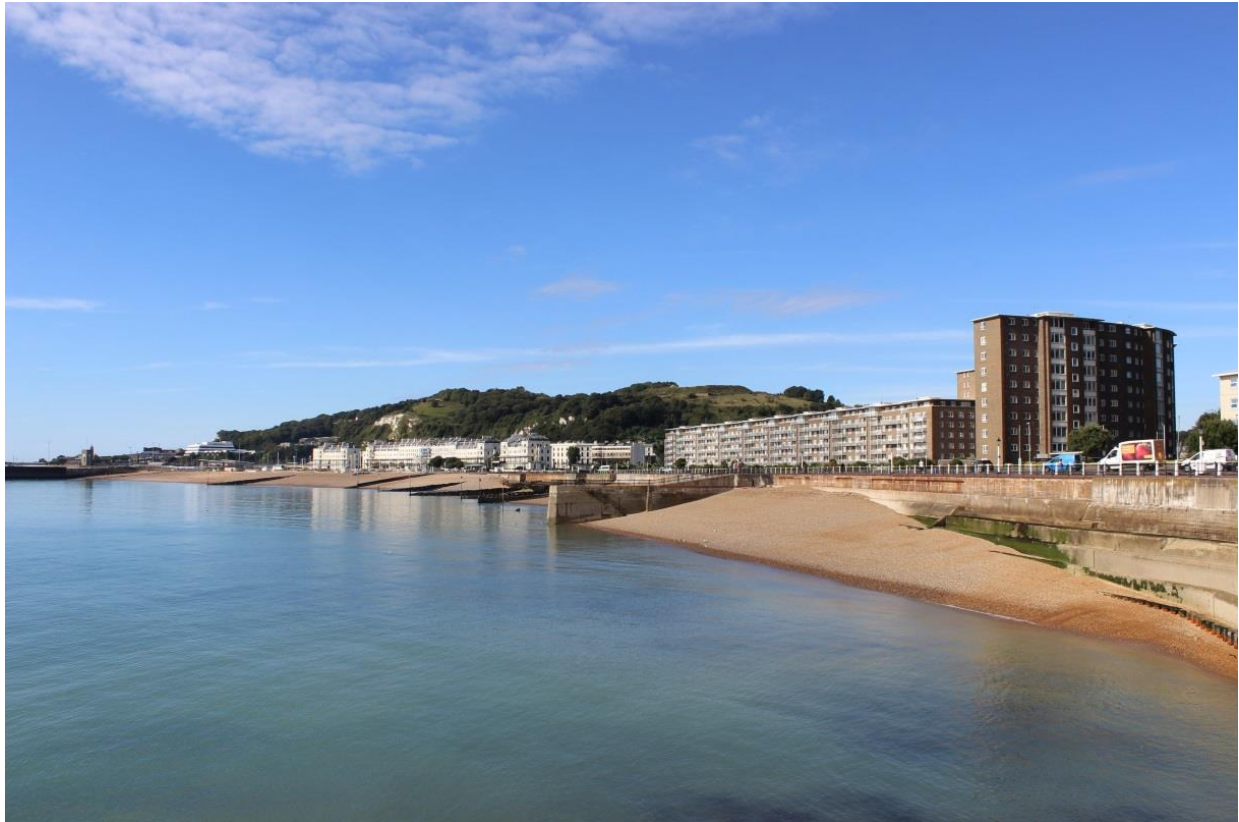
Plate 49: A look back at the Western Docks including the Waterloo Mansions and the Gateway Flats, 23/09/2016, looking south-west, DHB.
