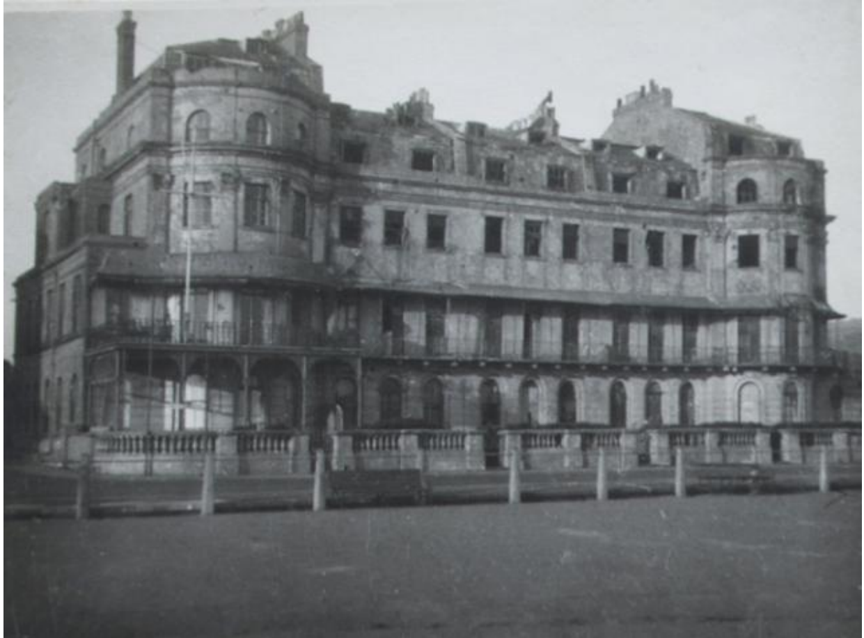
Plate 20: 3 Waterloo Crescent showing damages and dilapidation after WWII, c.1950, looking north-west, DHB.
