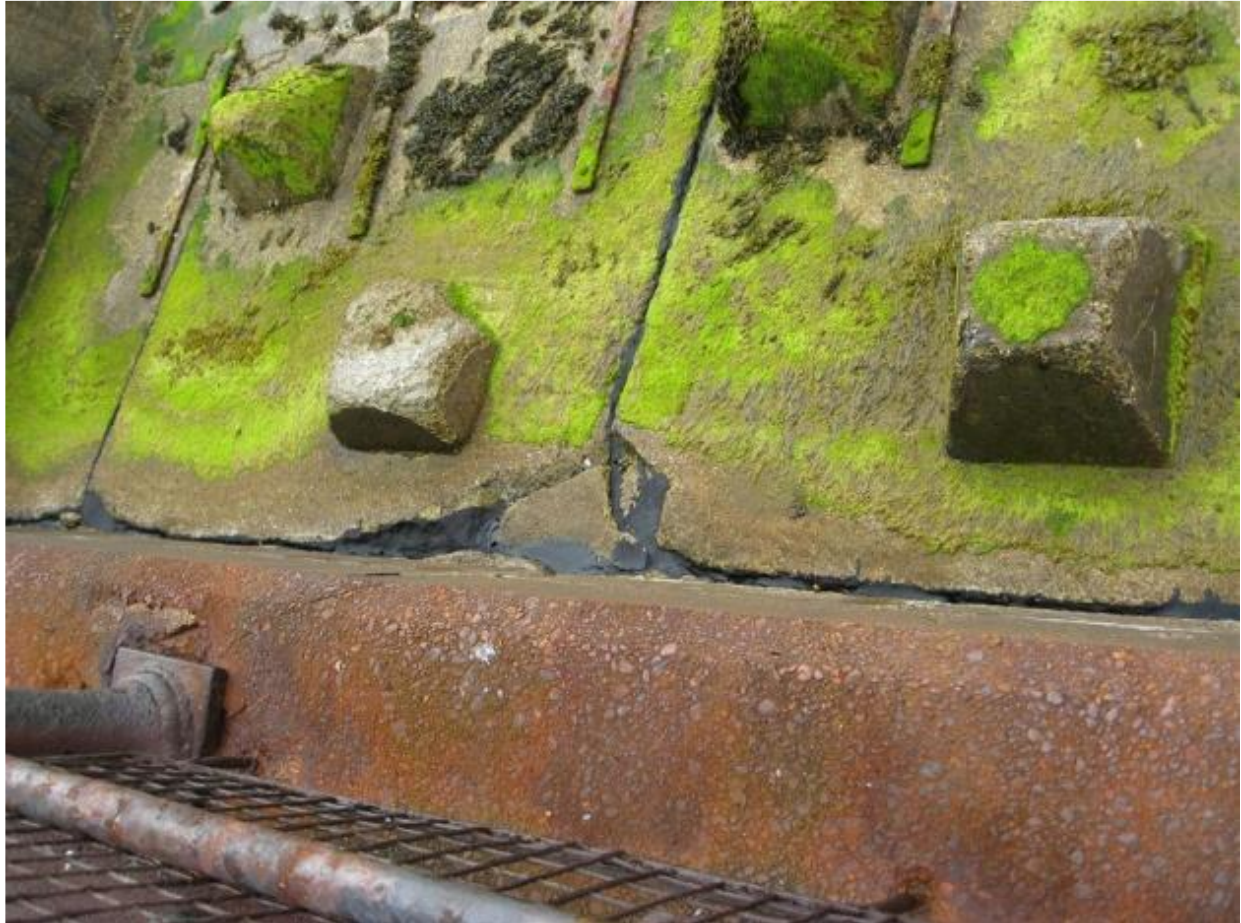
Plate 59: Looking down onto the dragons teeth which were installed into concrete, 2013, Atkins 2014, 25.
