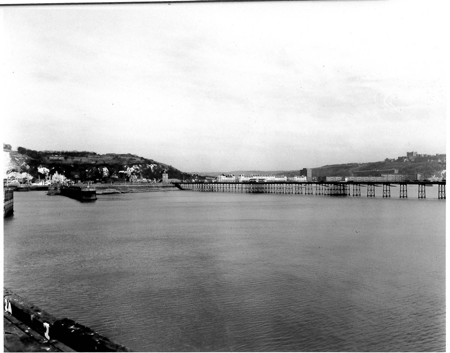
Figure 3: View from the Admiralty pier, of the Prince of Wales Pier before the reclamation works had started, the original Victorian lattice structure can be seen clearly, looking north-west, 05/04/1976, DHB.
