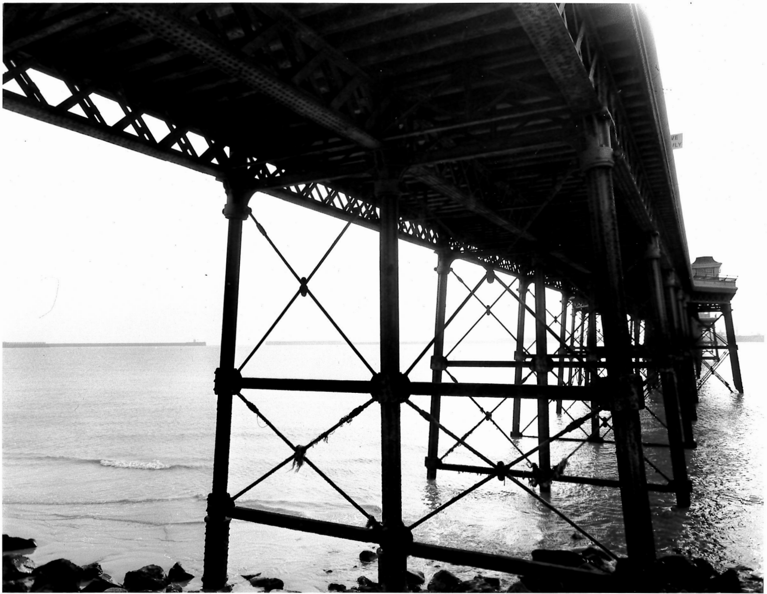
Figure 6: The original lattice steel structure that would have formed a large section of the Prince of Wales Pier, looking south-east, 05/04/1976, DHB.
