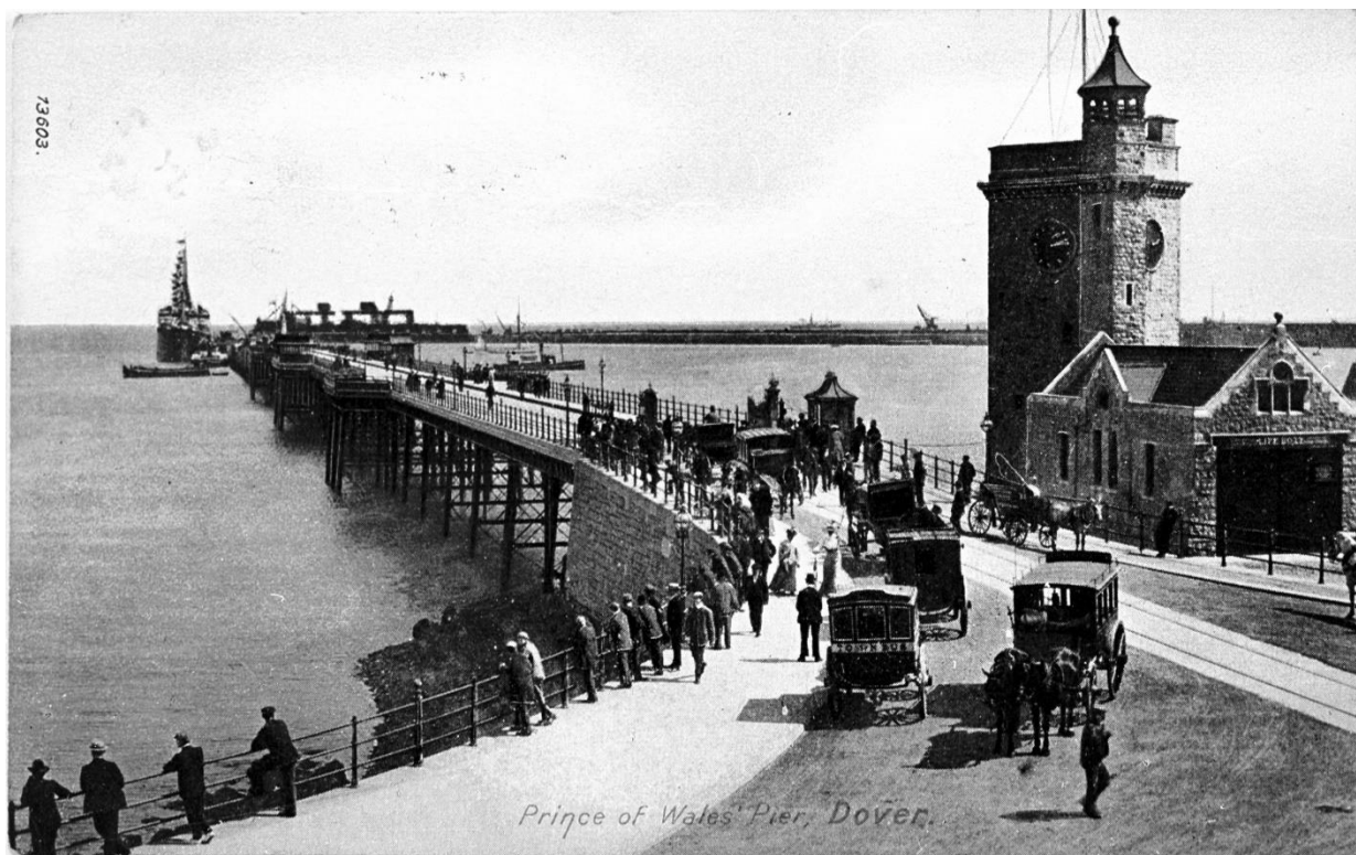
Plate 20- The newly completed pier and the existing clock tower, c.1903, Looking south-east, Clinton Collection Dover Museum d00616.
