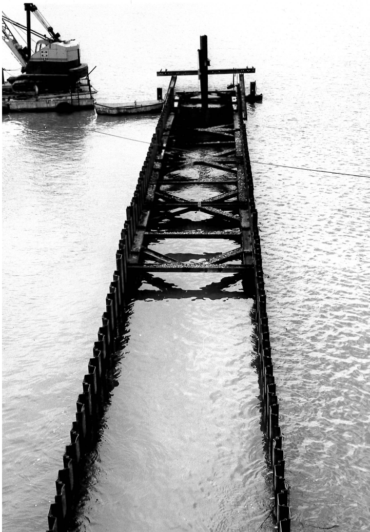
Figure 15: Staging for the construction works, 02/08/1976, DHB.
