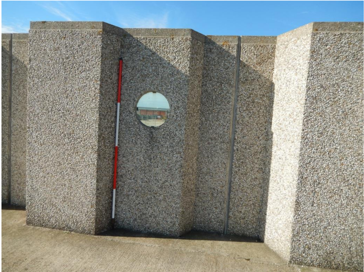
Plate 39: The windbreaker wall with added windows, this shows views of the Hoverport Apron, 03/09/15, looking South, DHB.
