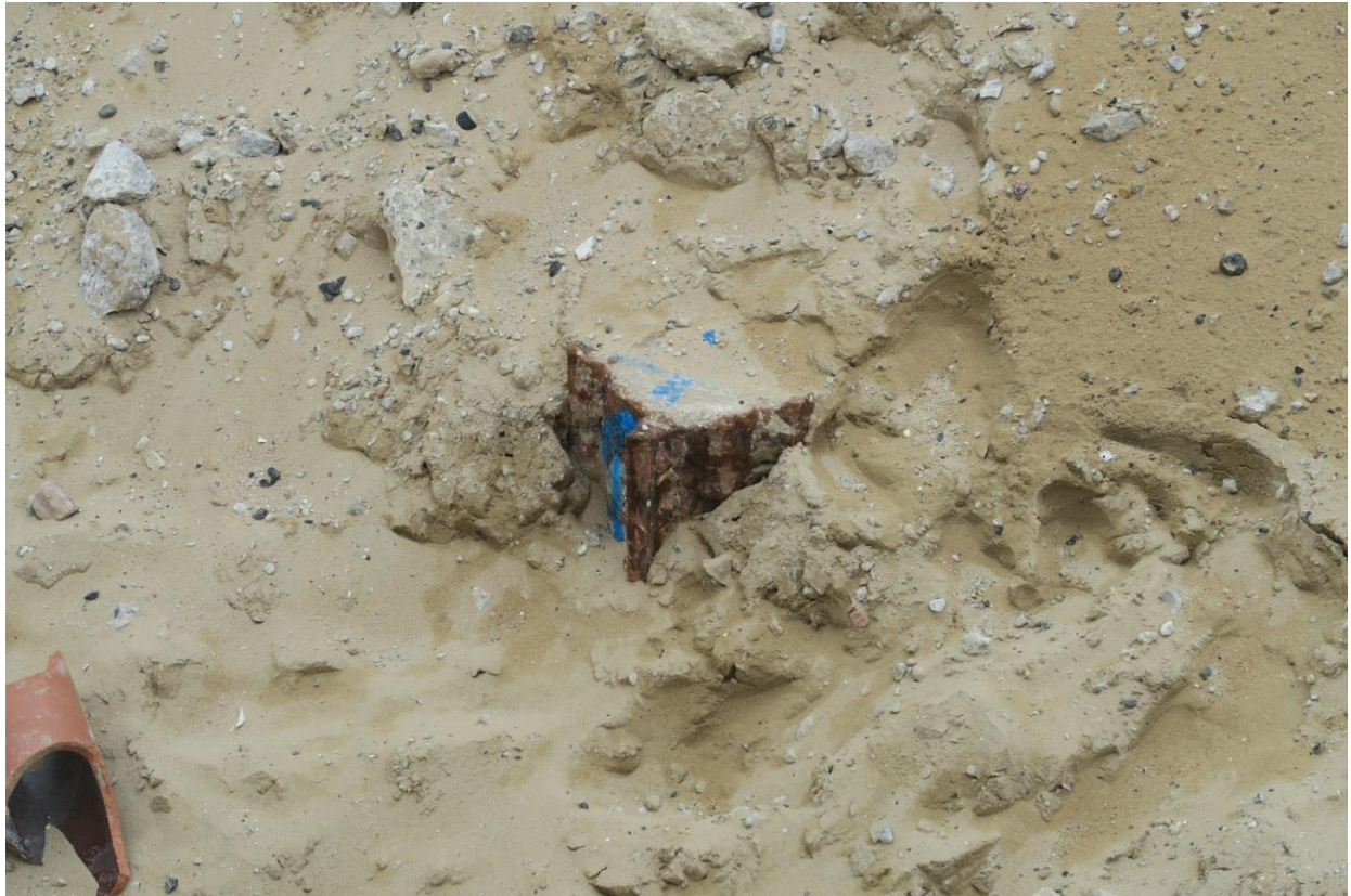
Plate 60: One of the original pile foundations for the Prince of Wales Pier, 14/10/16, DHB.
