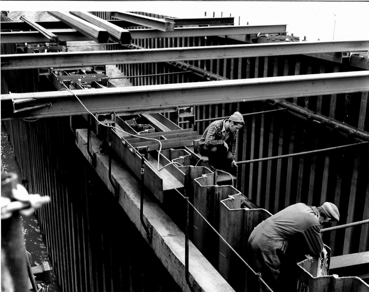
Figure 18: Construction workers attaching the sheet piling, 02/08/1976,, DHB.
