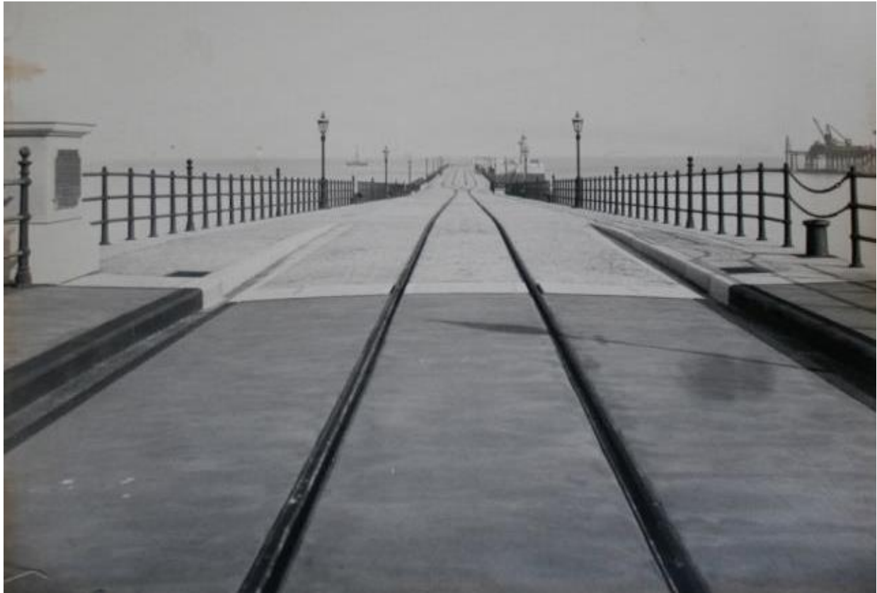
Plate 22- The train lines running centrally down the pier allowed passengers to directly get on or off liners when travelling c.1903, Looking south-east, DHB.
