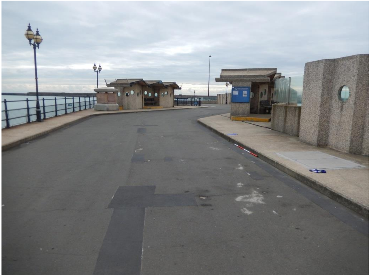
Plate 41: Concrete shelters, added alongside the Hoverport developments, 04/09/15, looking south-east, DHB.
