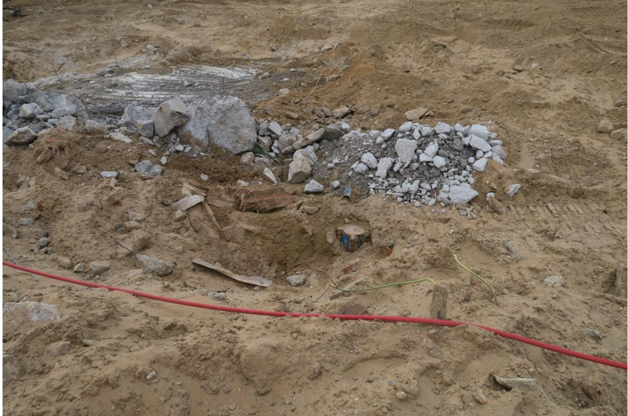
Plate 62: One of the original pile foundations for the Prince of Wales Pier, 26/10/16, DHB.
