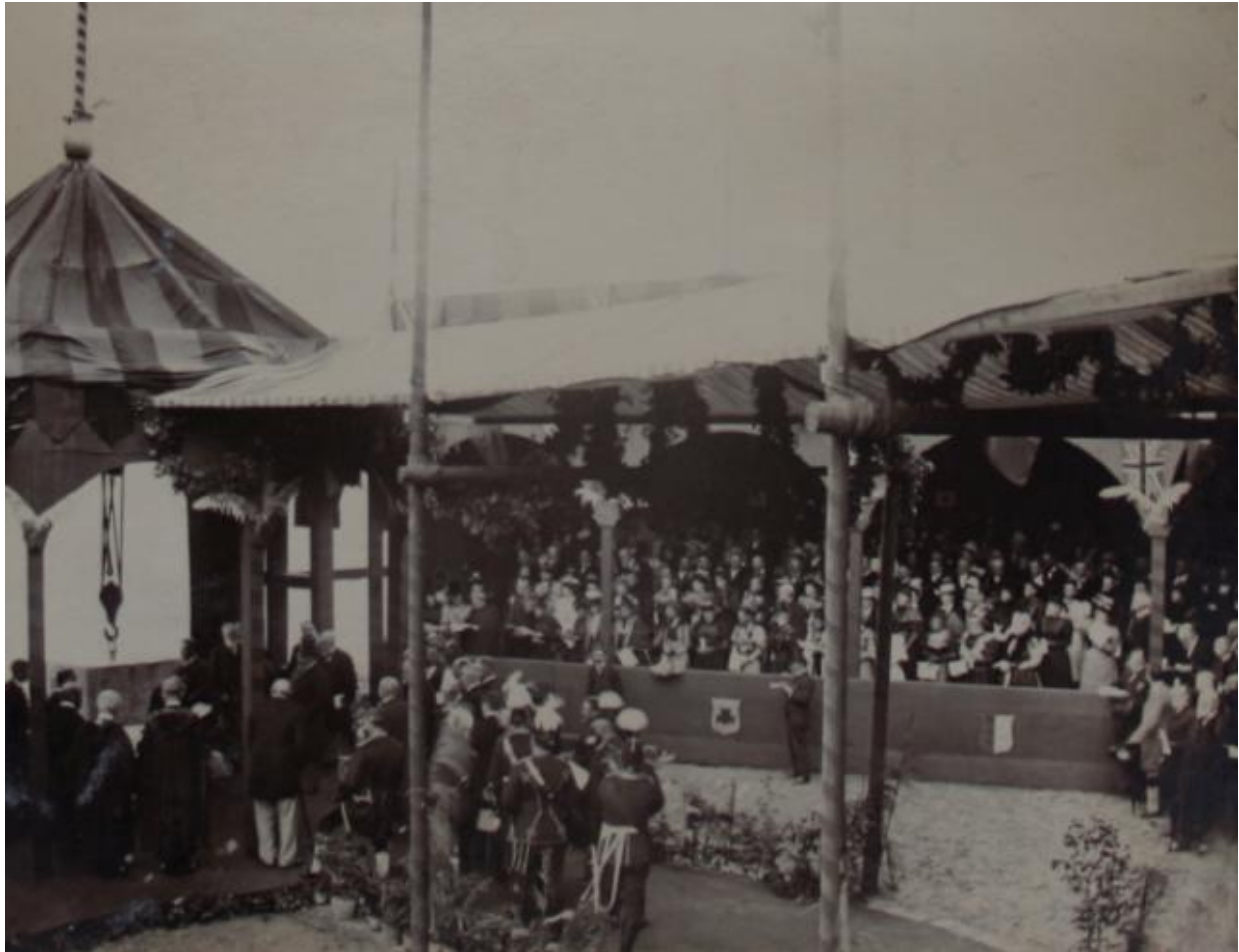
Plate 2- The stands for the crowds watching the foundation stone being laid, the stone is visible to the left hand side of the image, 14/07/1893, DHB.
