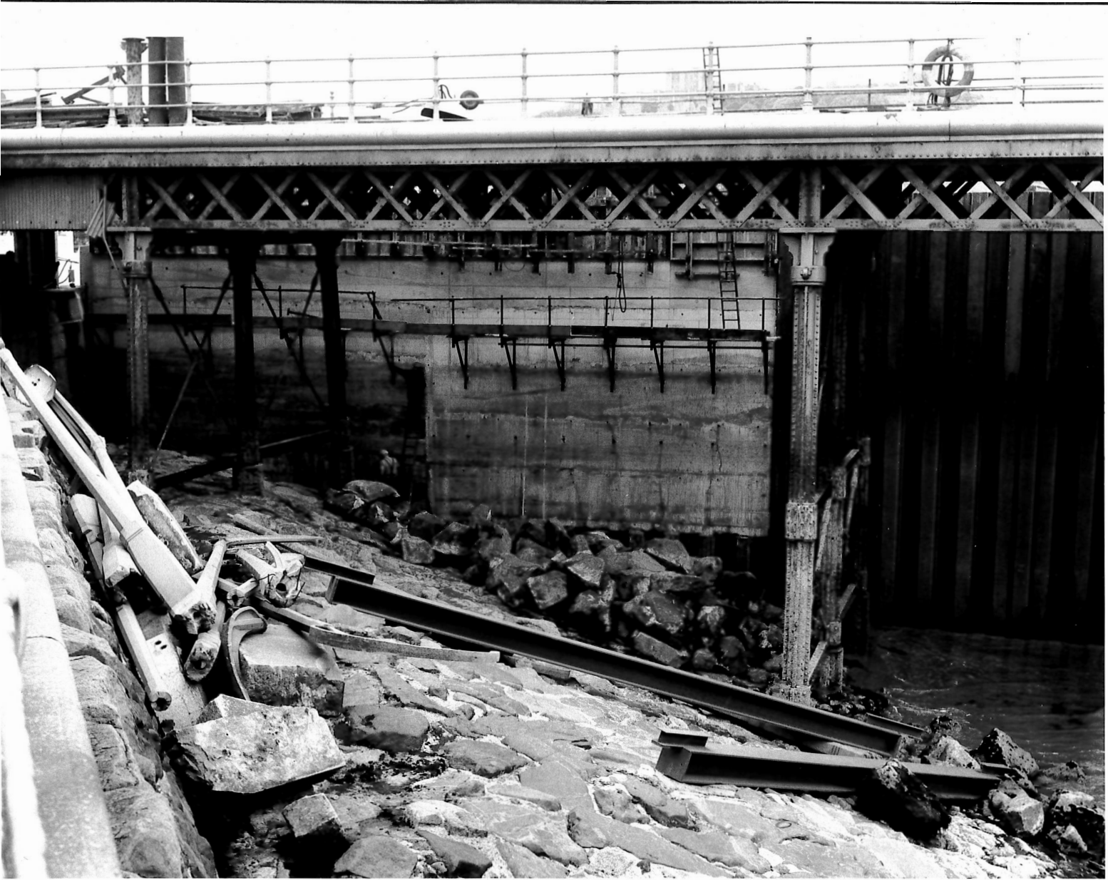
Figure 19: Both original and added material to the pier, concrete and steel structures can be seen, looking North, 02/08/1976, DHB.
