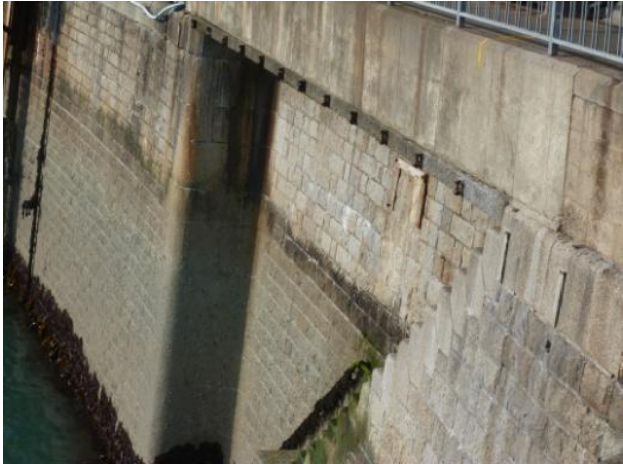
Plate 48: A stepped recess which is no longer in use as a suspended masonry deck has been added over the top of it, looking North back at the side of the pier, Atkins 2014B: 21.
