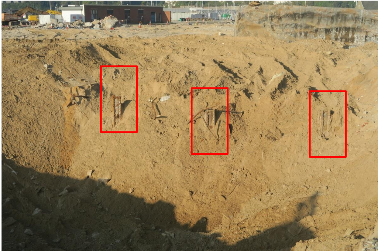
Plate 64: Three of original pile foundations for the Prince of Wales Pier, highlighted in red, 26/10/16, DHB.
