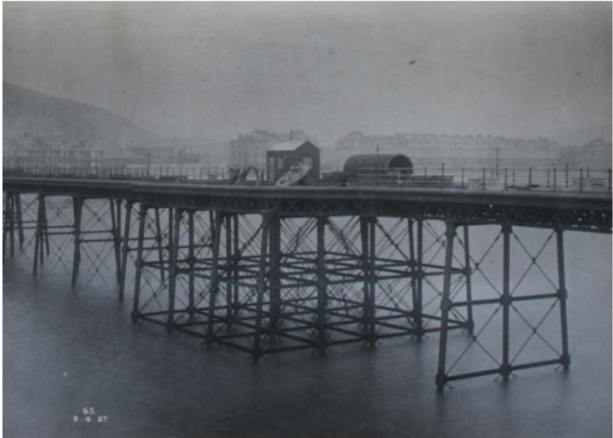
Plate 15- The finished iron structure can be seen here with some works still taking place on the pier 9/04/1897, Looking north-west, DHB.
