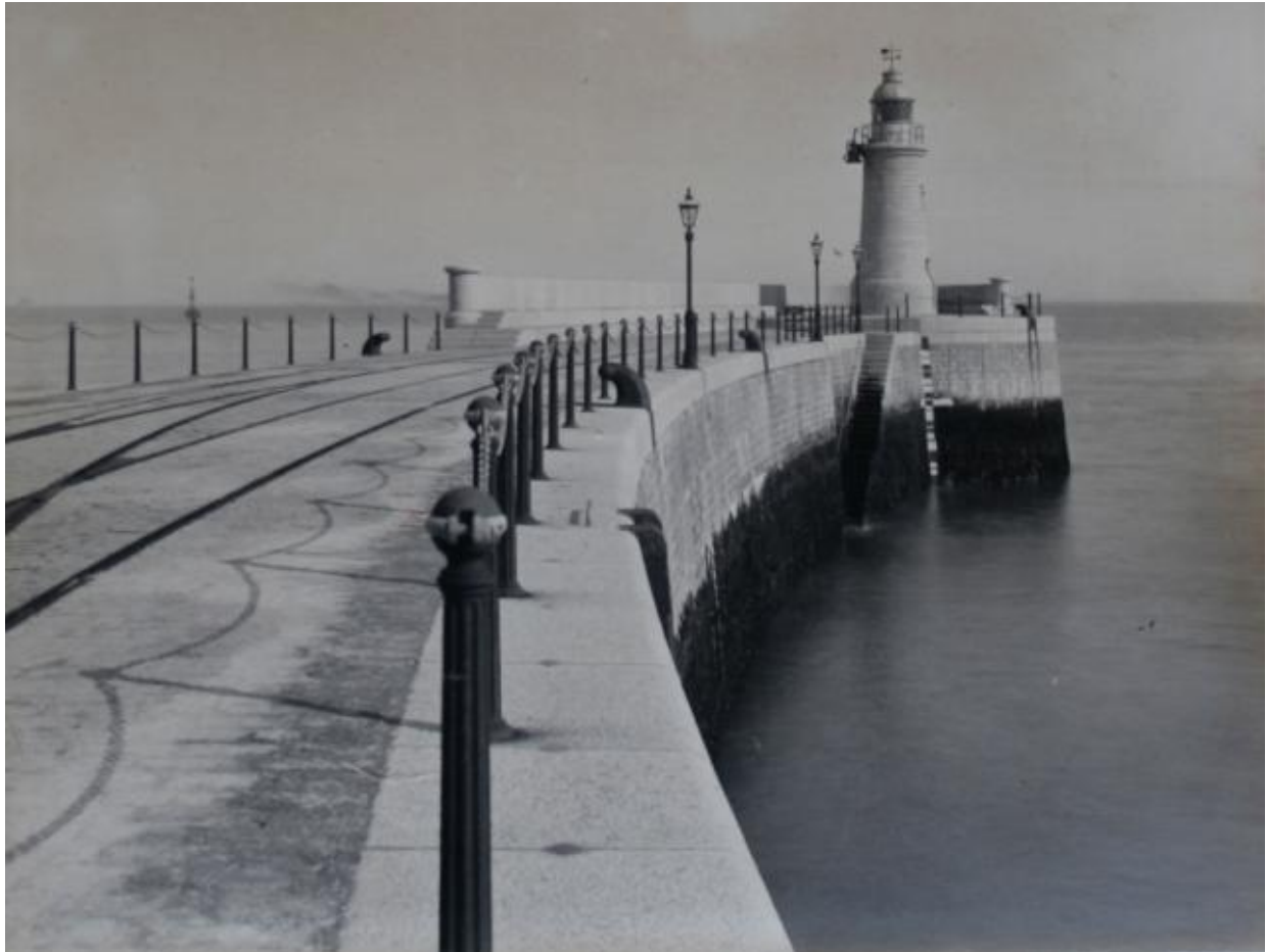
Plate 18- The seaward end of the pier looking towards the newly constructed light house c.1903, Looking south-east, DHB.
