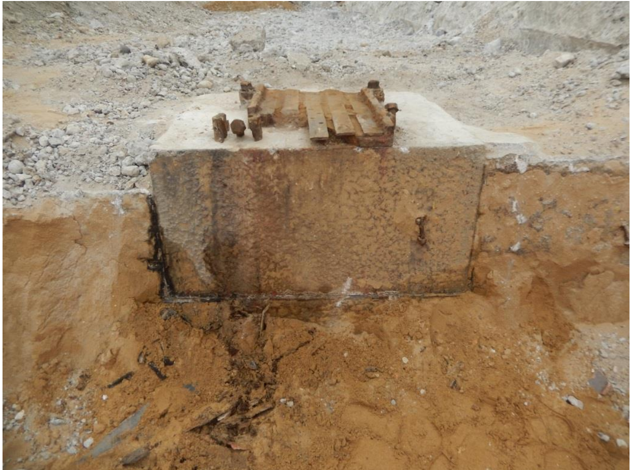
Plate 67: The remaining connecting joist, looking West, 28/7/2016, DHB.
