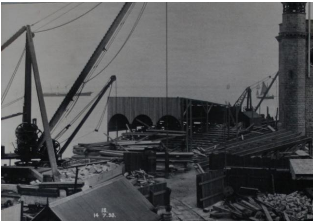
Plate 1- Preparations taking place for the stage work hosting the laying of the stone, 14/07/1893, looking South, DHB.
