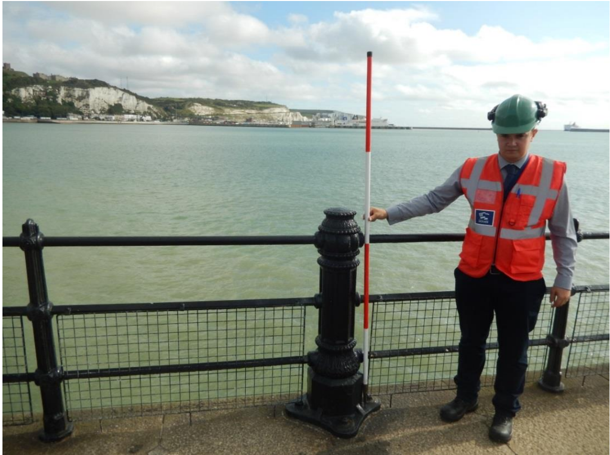
Plate 38: One of the original lamp post bases from c.1900, 02/09/15, looking North, DHB.
