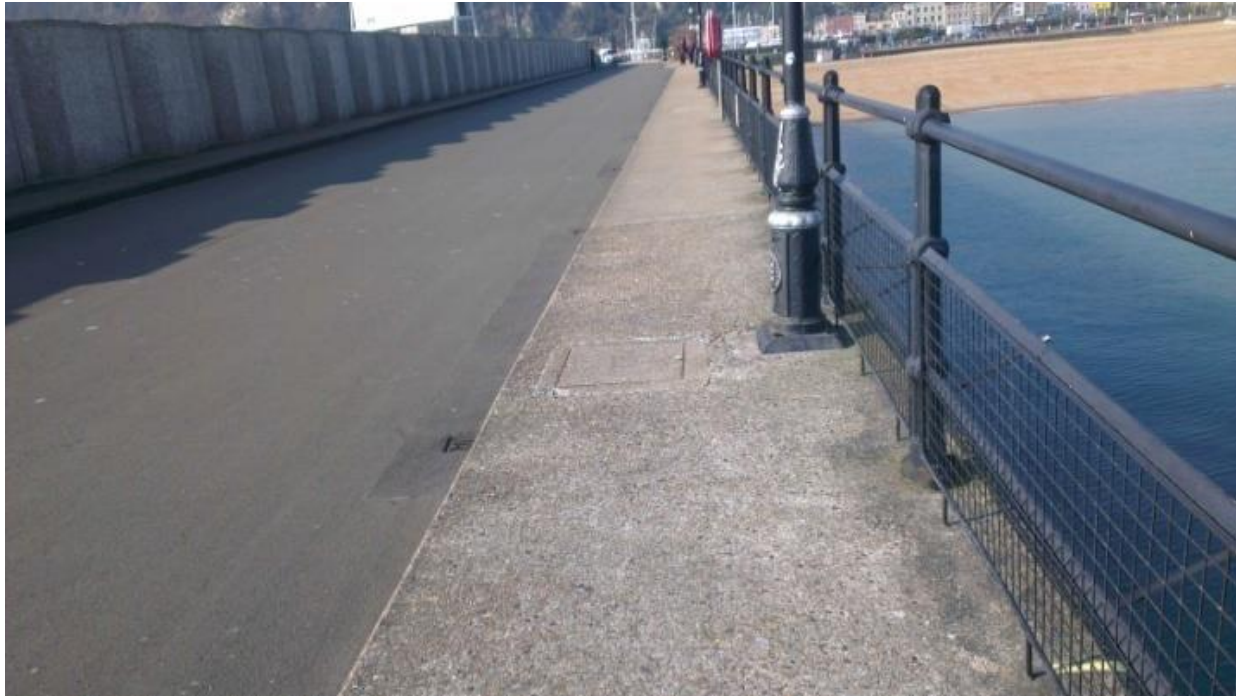
Plate 40: Looking back towards the landward end of the pier and the entrance, looking north-west, Atkins 2014A: 46
