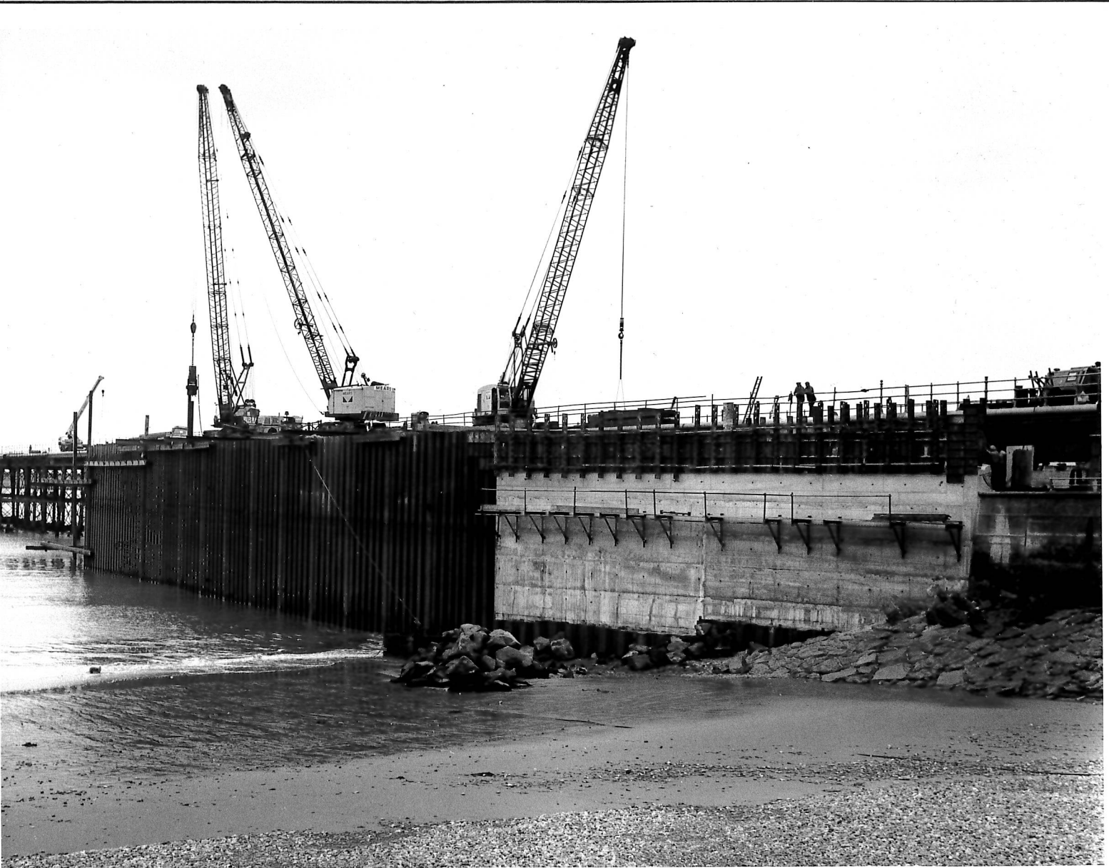
Figure 16: Work has progressed here with the majority of the landward end of the pier being covered, 02/08/1976, DHB.
