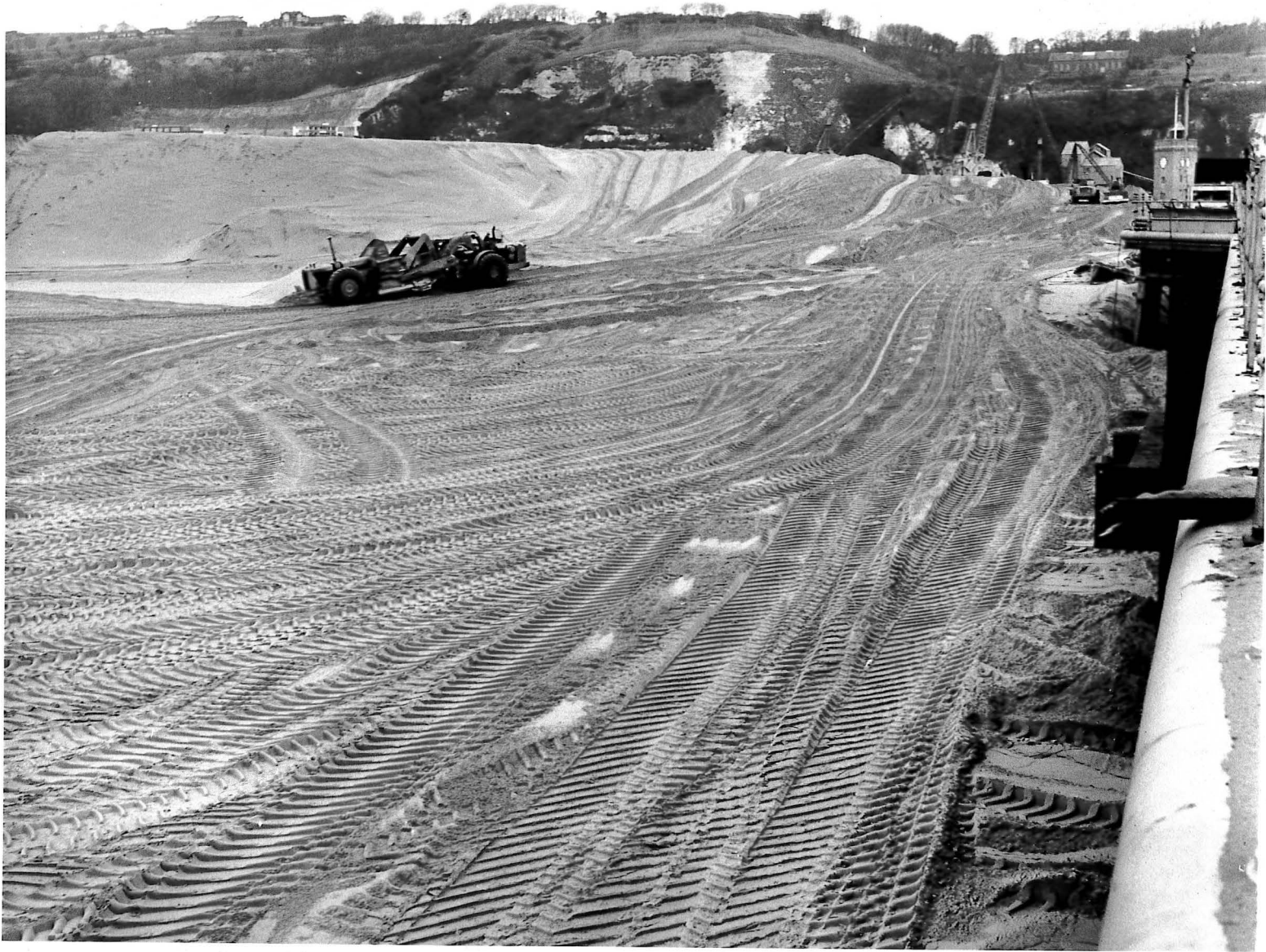
Figure 2: The land which has been reclaimed in order to create a foundation for the rest of the works, looking West, 13/01/1976, DHB.
