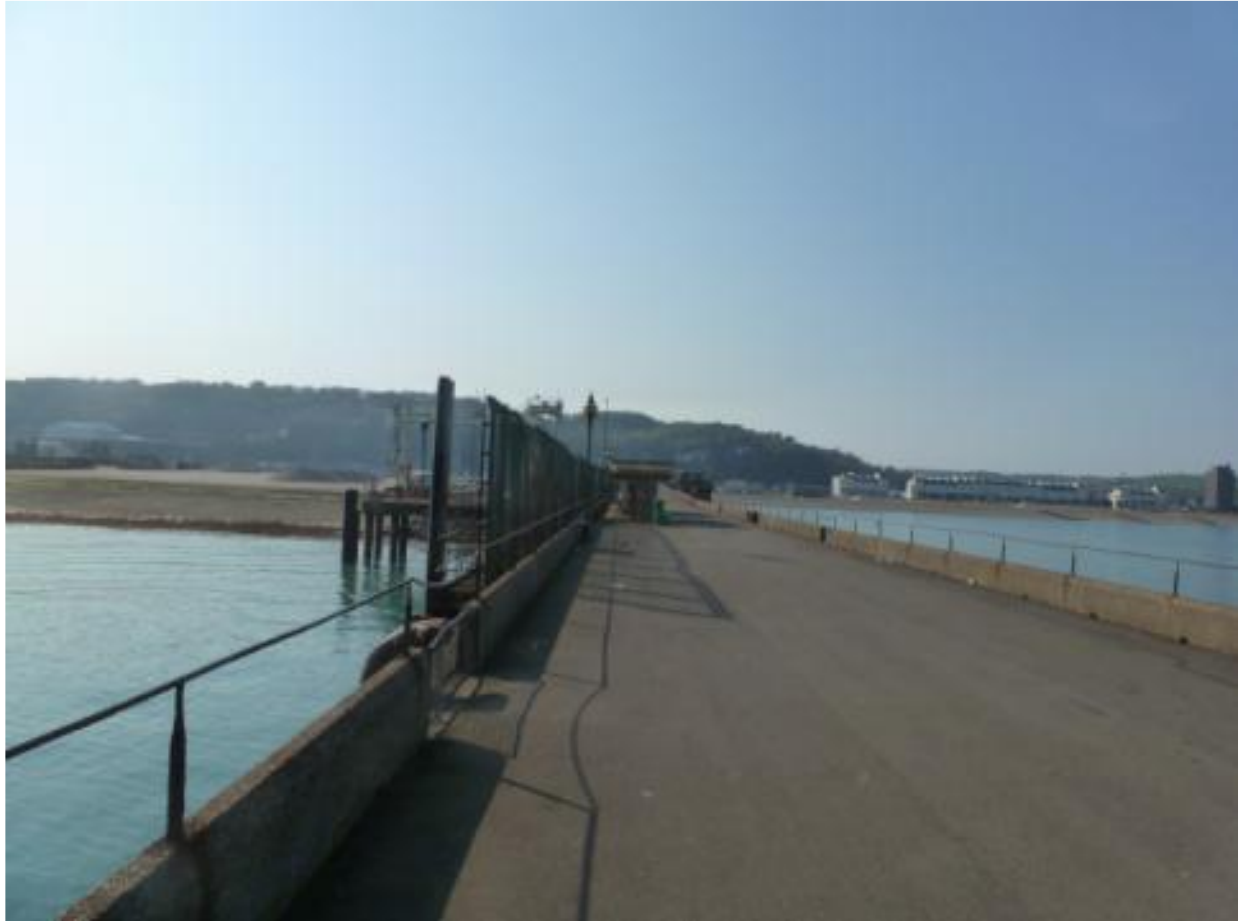
Plate 42: Looking back towards the landward end of the pier, also with the Hoverport to the left, looking West, Atkins 2014B: 17.
