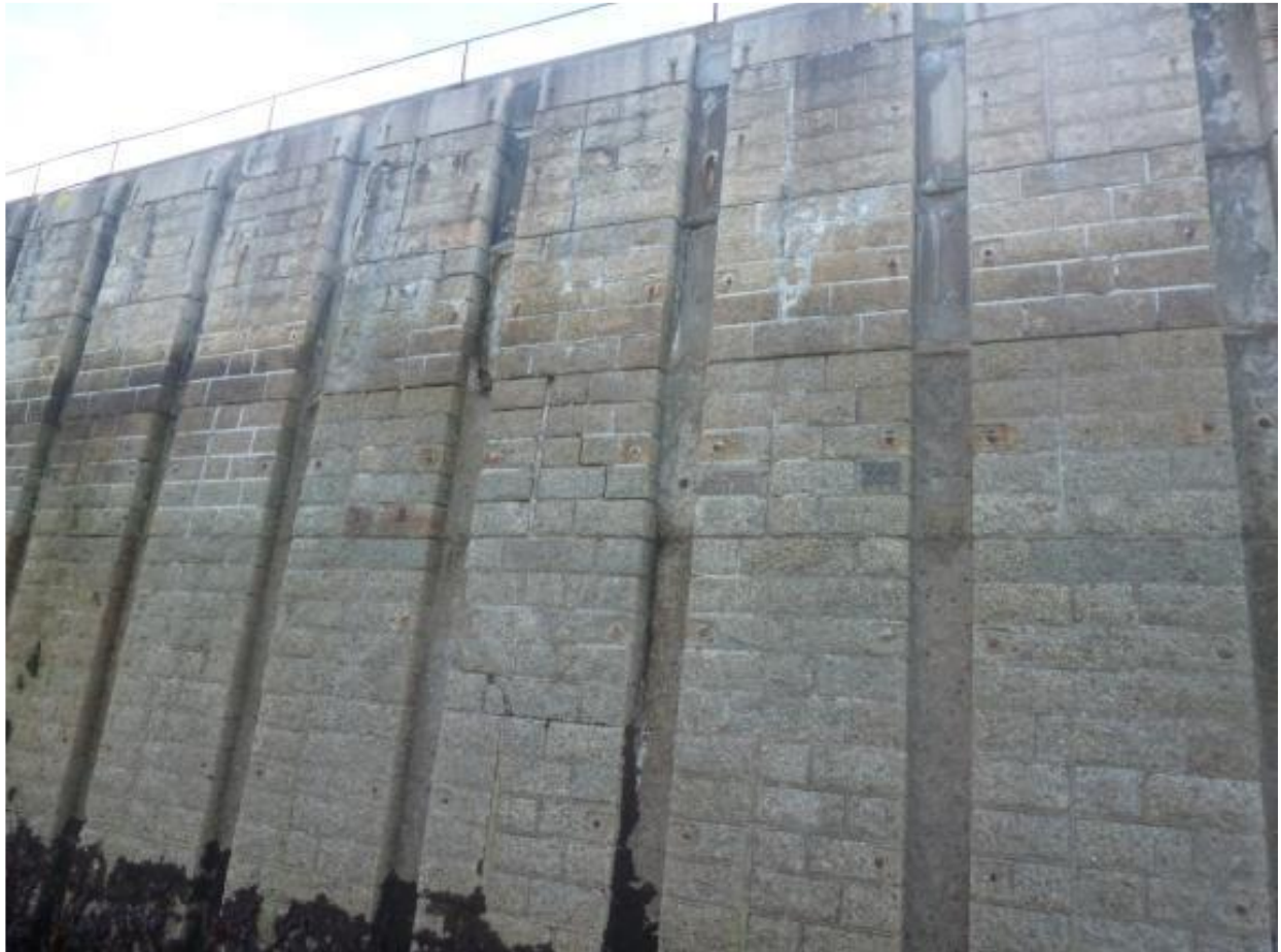
Plate 32: Recesses of previous timber fenders, no longer in use, Atkins 2014B: 32.
