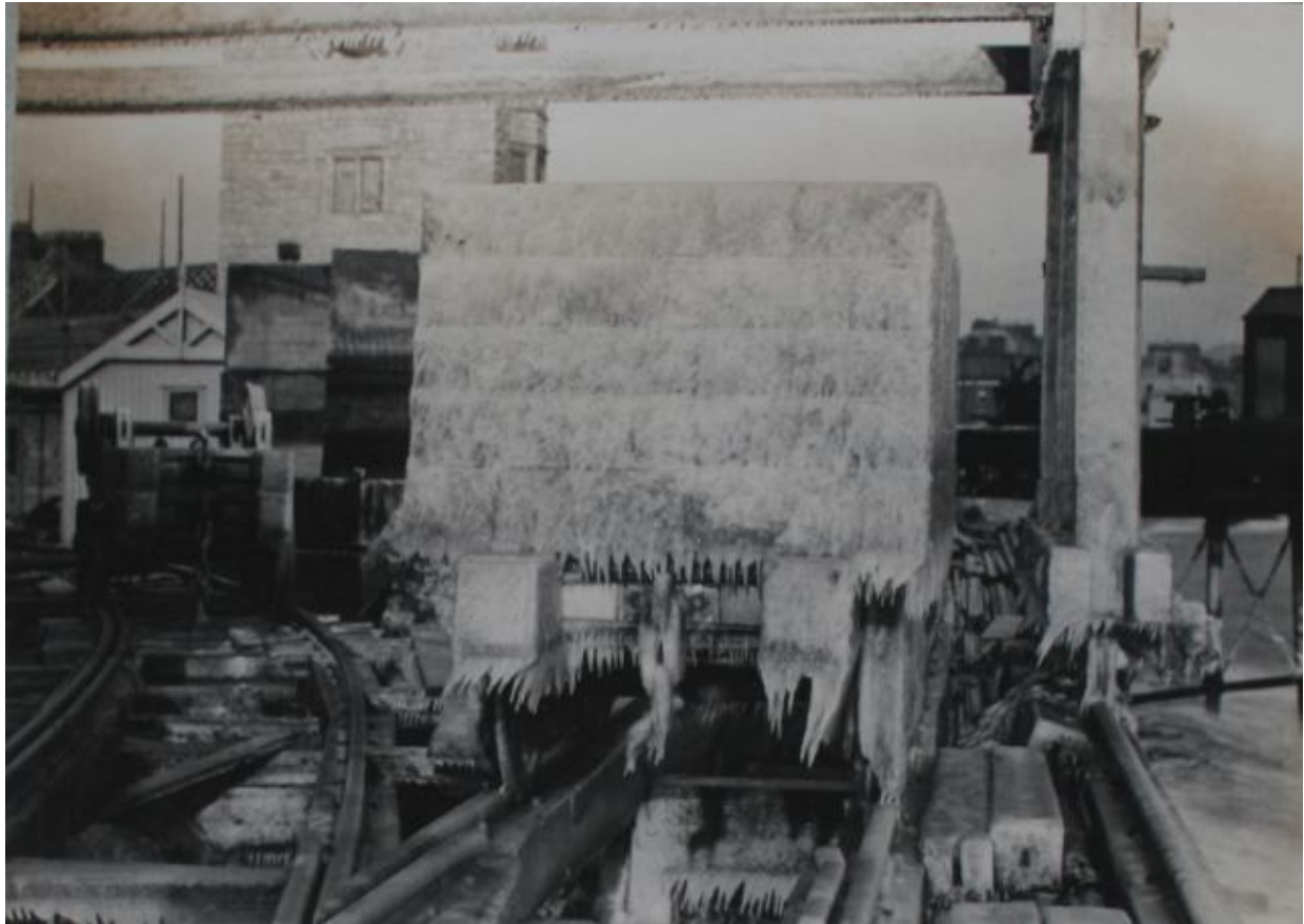
Plate 7- A cold spell during the construction, the clock tower can be seen in the background, 1893, DHB.
