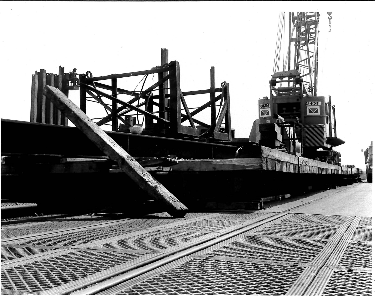
Figure 12: Site works for the Hoverport development, looking north-east, 18/06/1976, DHB.
