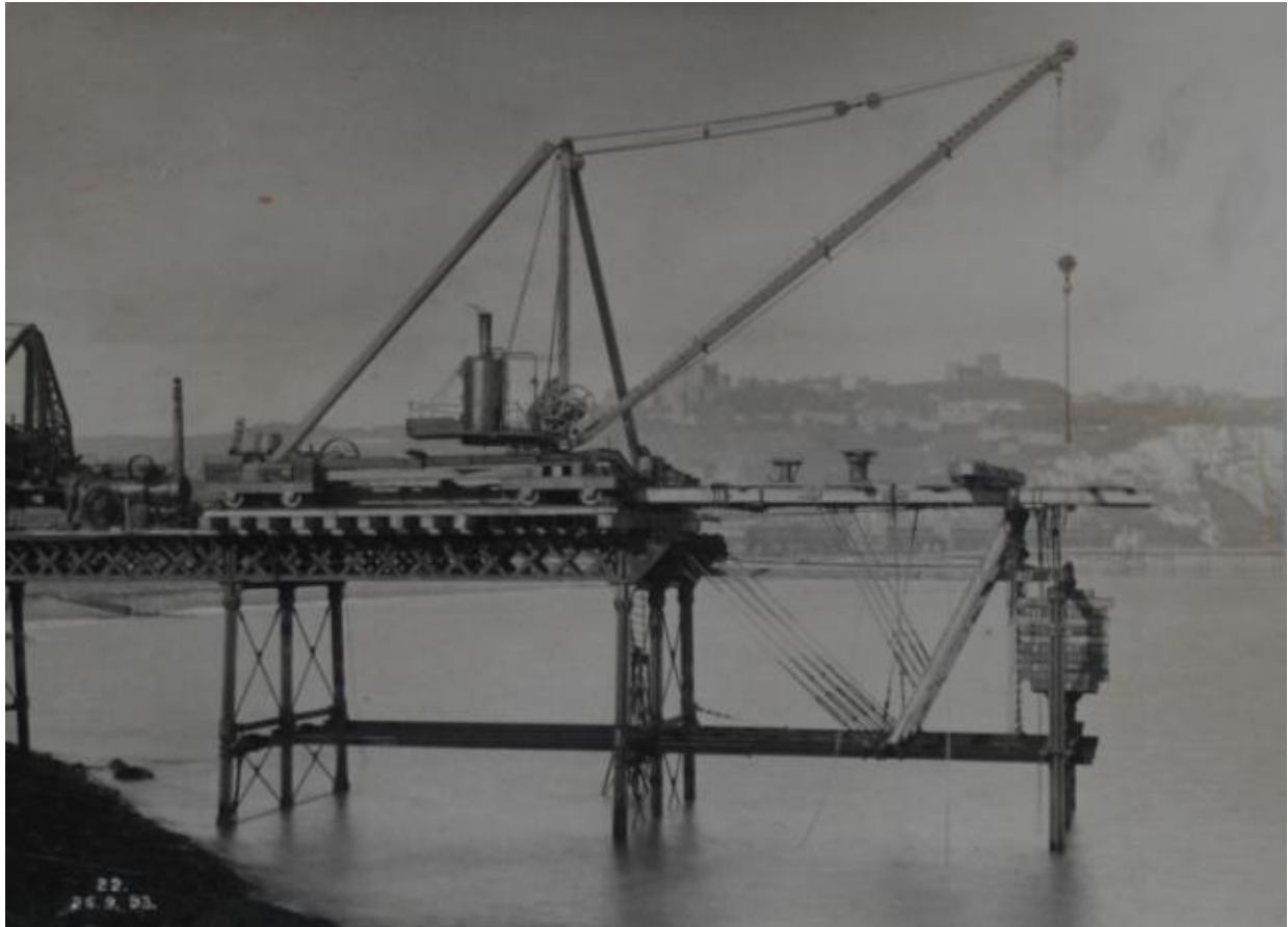
Plate 5- An old steam crane working on the foundations of the Prince of Wales Pier, 1893, looking north, DHB.
