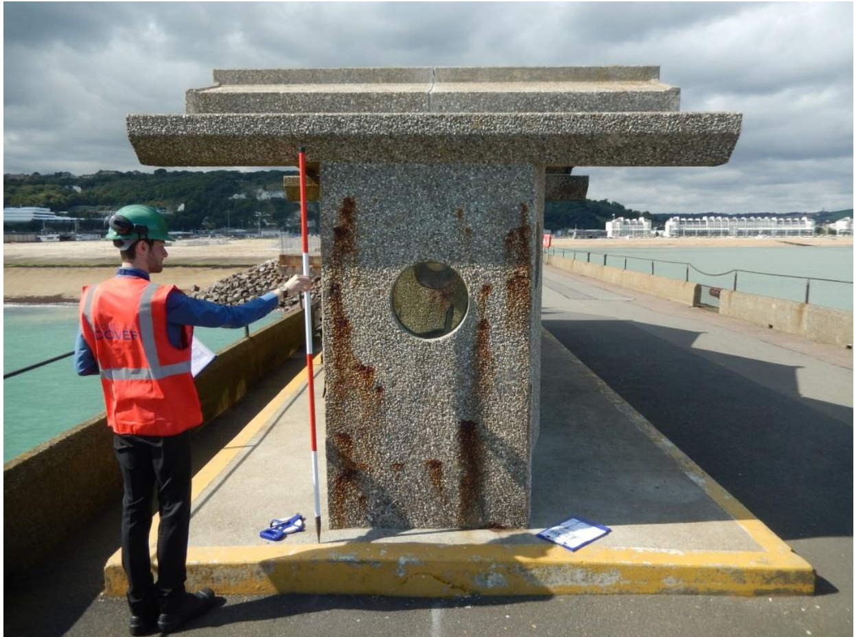
Plate 44: Concrete shelter to the left hand side of the Prince of Wales Pier, The Hoverport can be seen on the left and Waterloo Crescent on the right, 08/09/2015, looking north-west, DHB.
