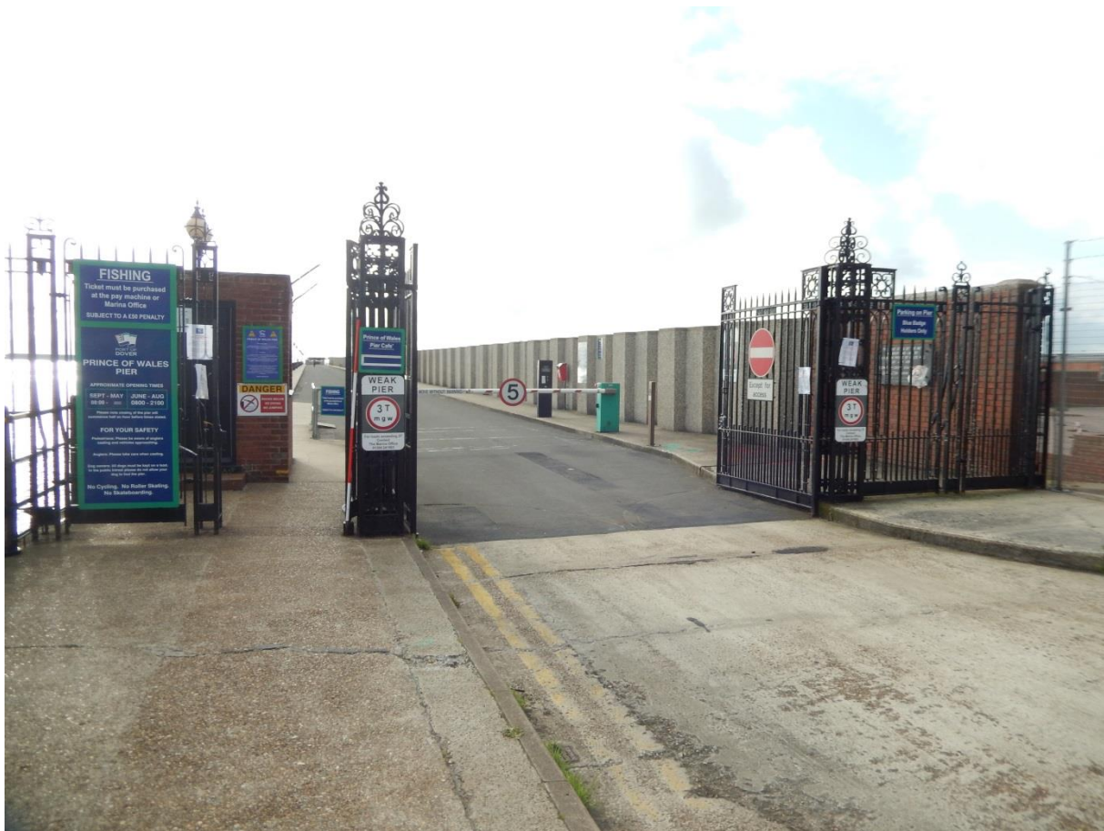
Plate 36: The Entrance to the Prince of Wales Pier, Looking South, 02/09/15, DHB.
