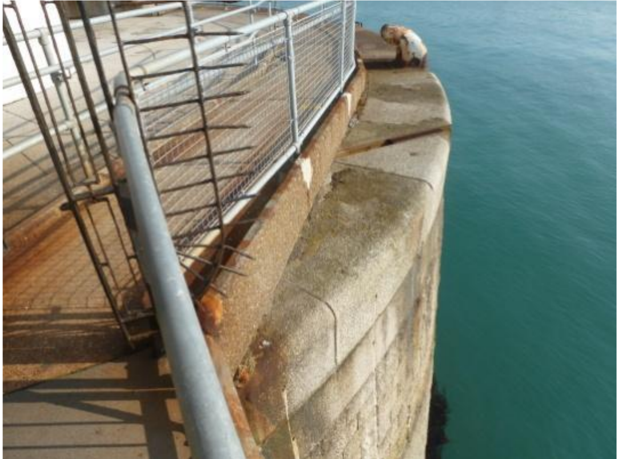
Plate 49: Roundhead stone at the end of the pier, also the supporting foundations for the lighthouse formed of granite blocks, Atkins 2014B: 21.
