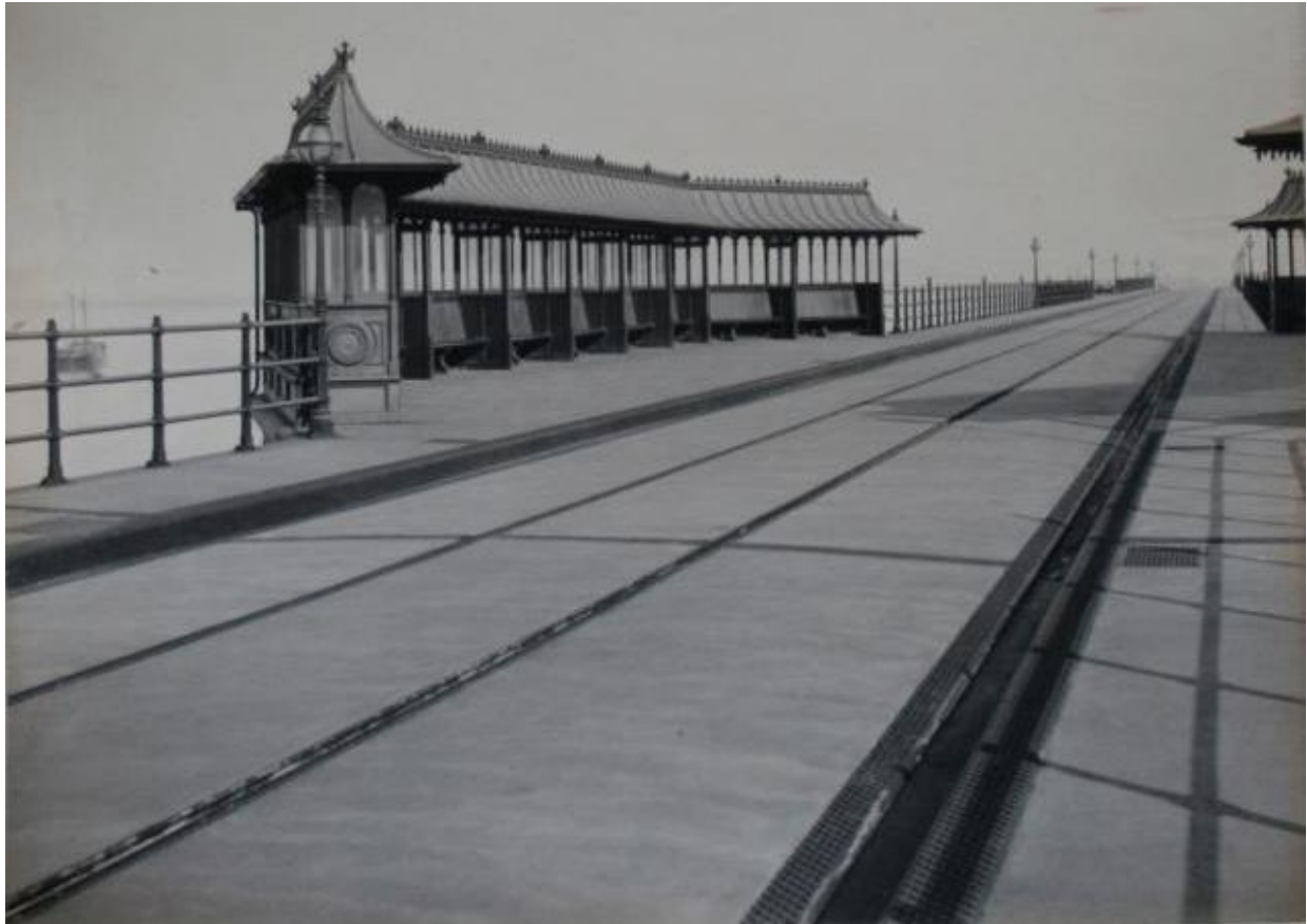
Plate 21- The shelters which were installed on the pier to encourage those walking to look back at the harbour and the castle, the train line can also be seen c.1903, Looking north-east, DHB.
