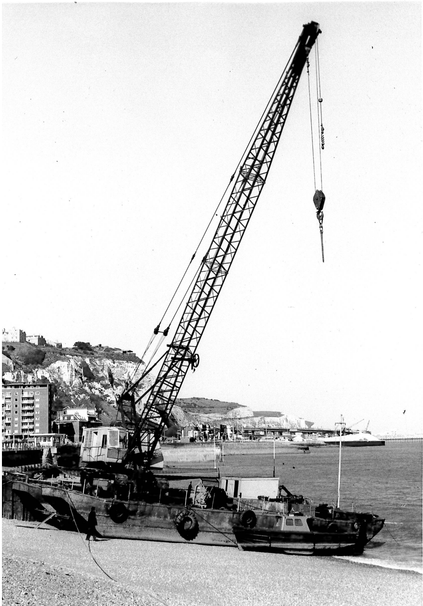
Figure 8: Lifting cranes for use within the construction of the Hoverport, looking North, 28/4/1976, DHB.
