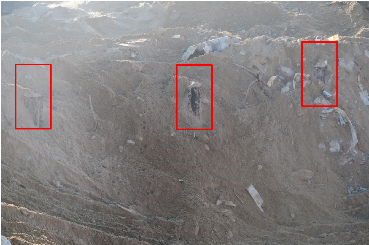
Plate 63: Three of original pile foundations for the Prince of Wales Pier in context with one another, highlighted in red, 26/10/16, DHB.
