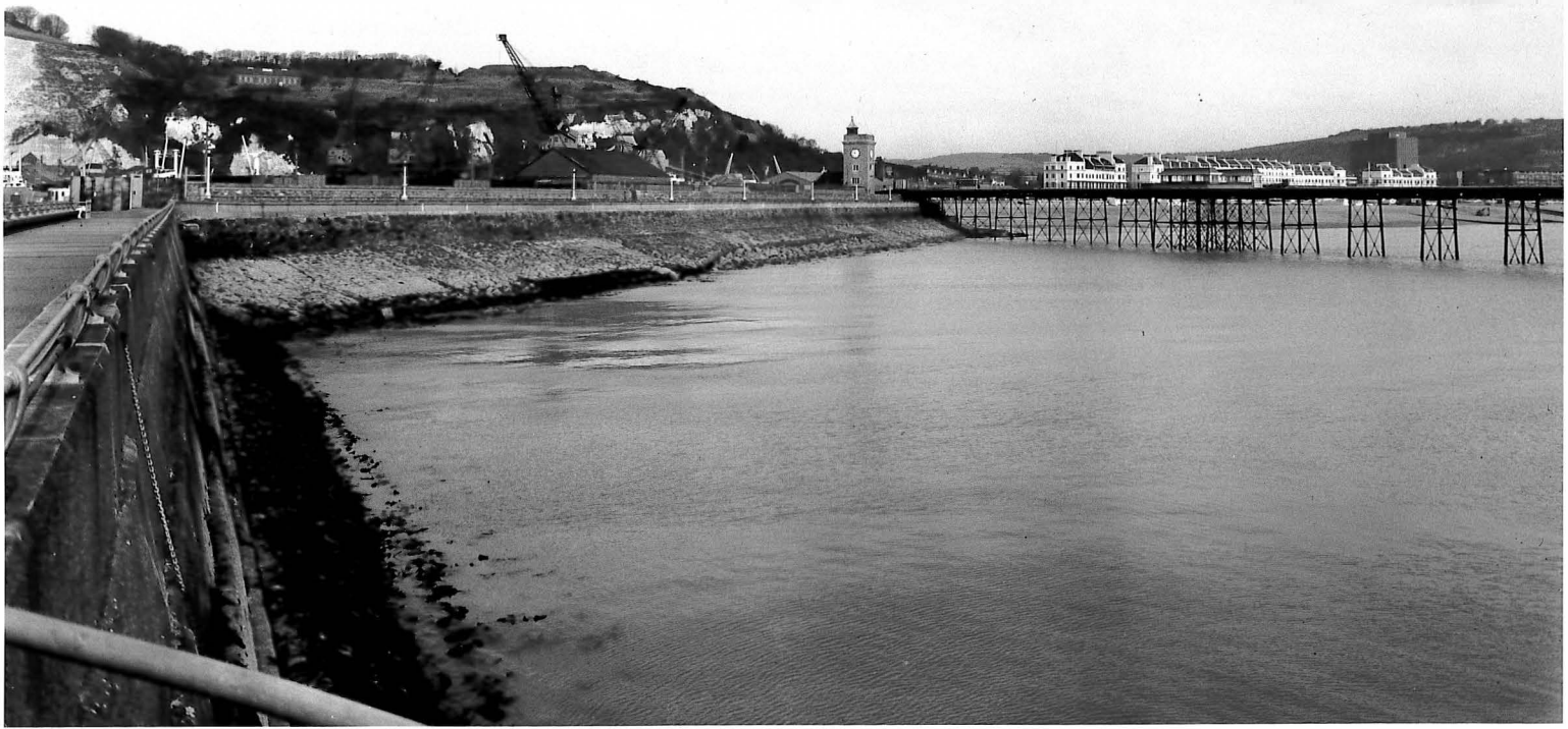
Figure 5: Looking back on sea that will be reclaimed whilst standing on the North pier, looking West, 05/04/1976, DHB.
