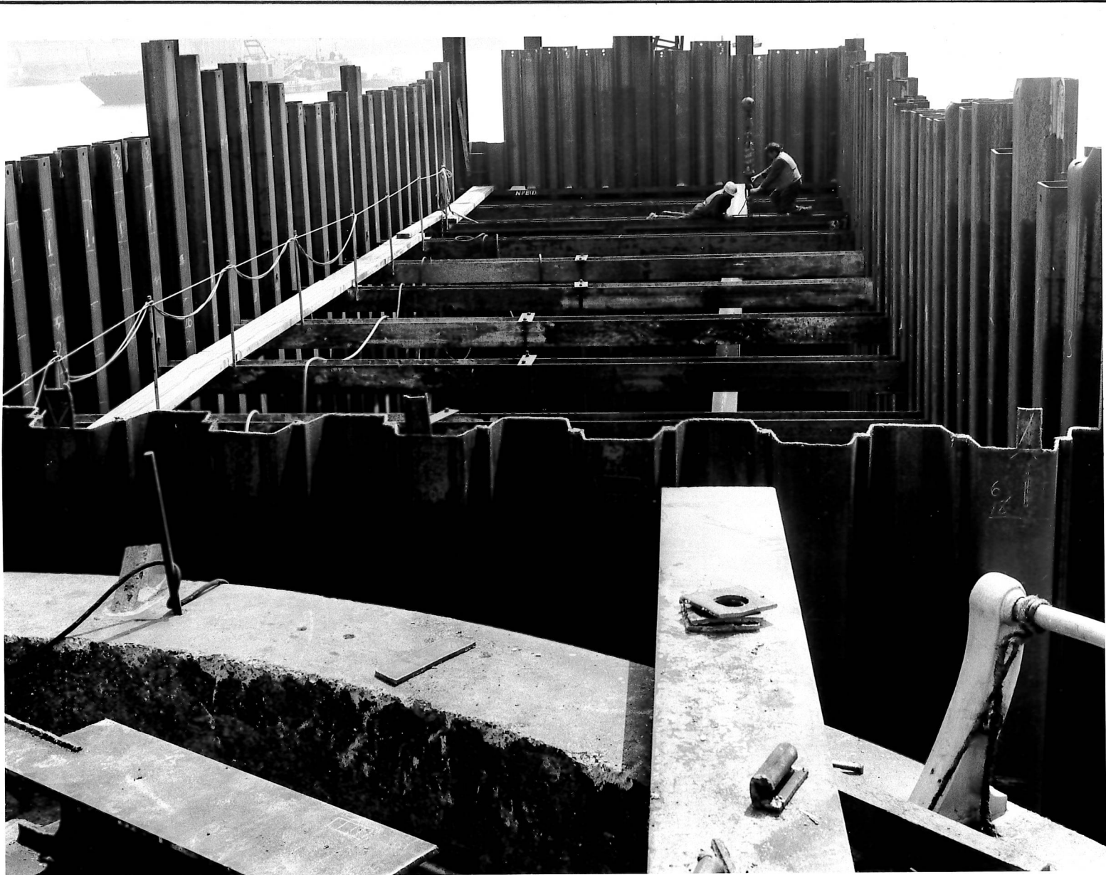
Figure 14 Piling preparation works, 18/06/1976, DHB.
