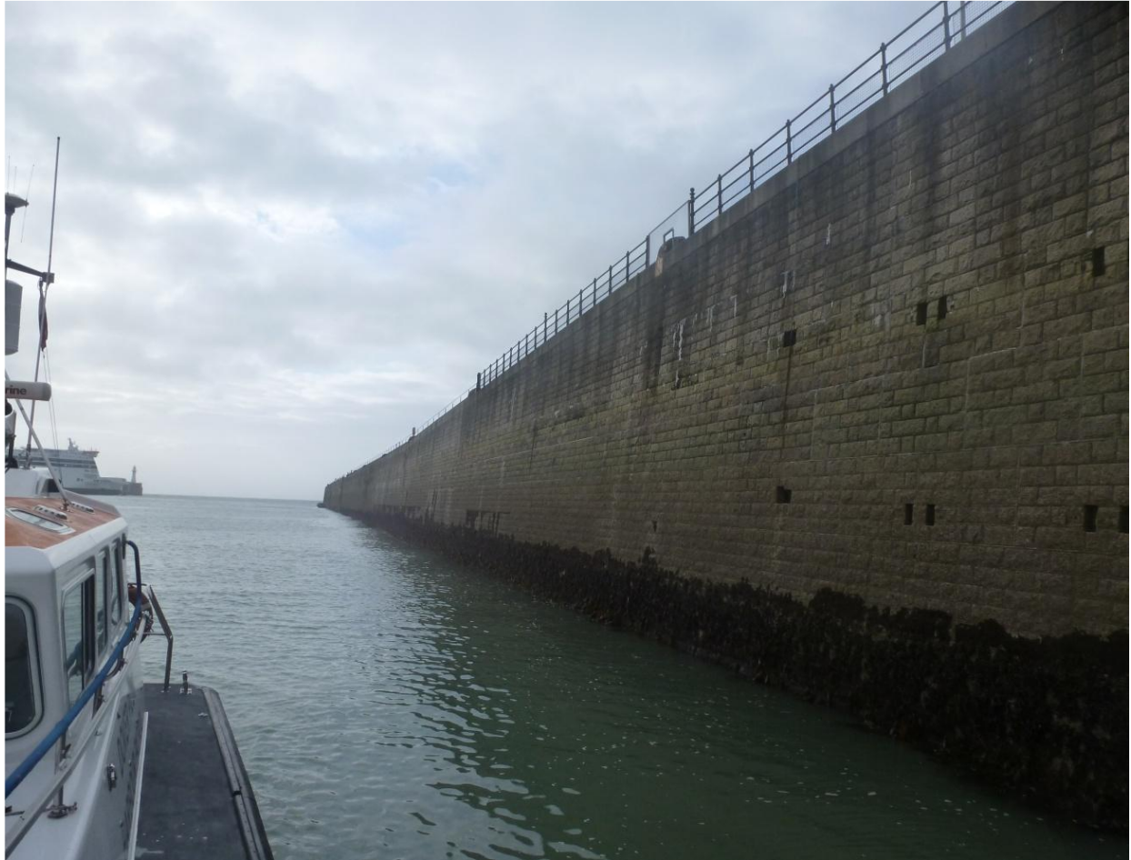
Plate 35: General view of the masonry section of the Prince of Wales Pier, looking East, Atkins 2014B: 9.
