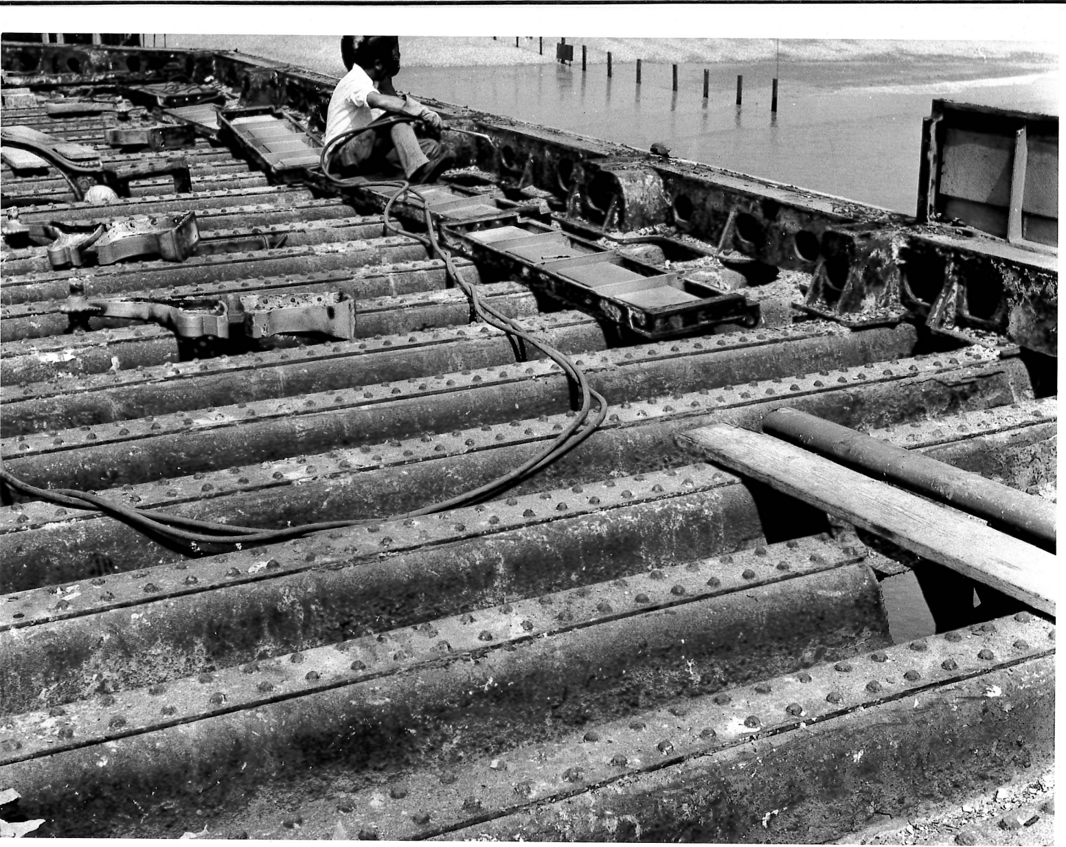
Figure 13: Pile foundations, looking North, 18/06/1976, DHB.
