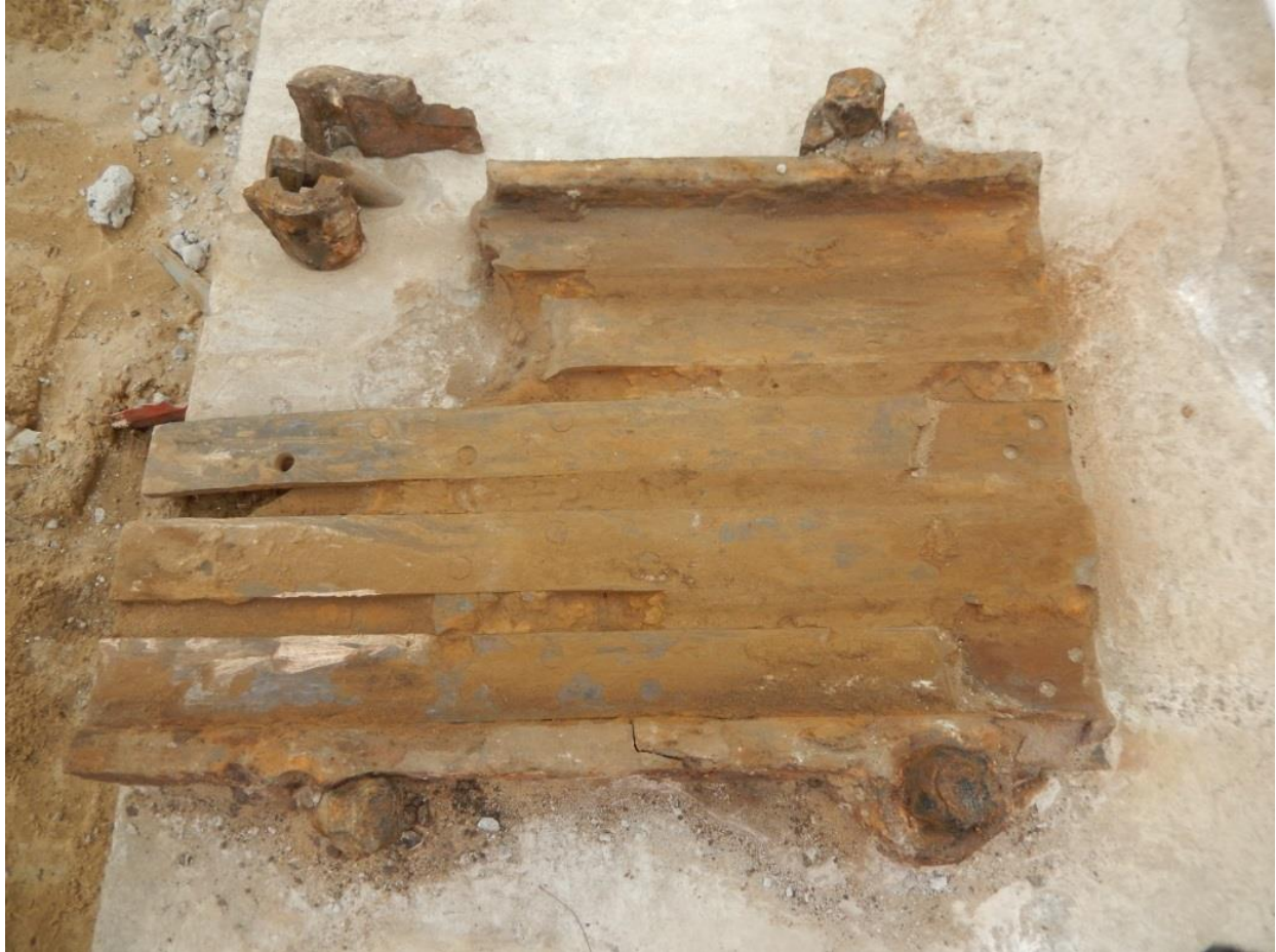
Plate 69: A detail of the remaining connecting joist, 28/7/2016, DHB.
