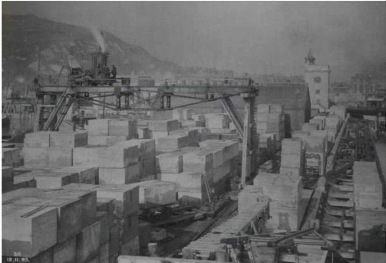
Plate 11- The brick yard was being used to store materials before they were ready to be used in the construction 18/11/1895, Looking North, DHB.
