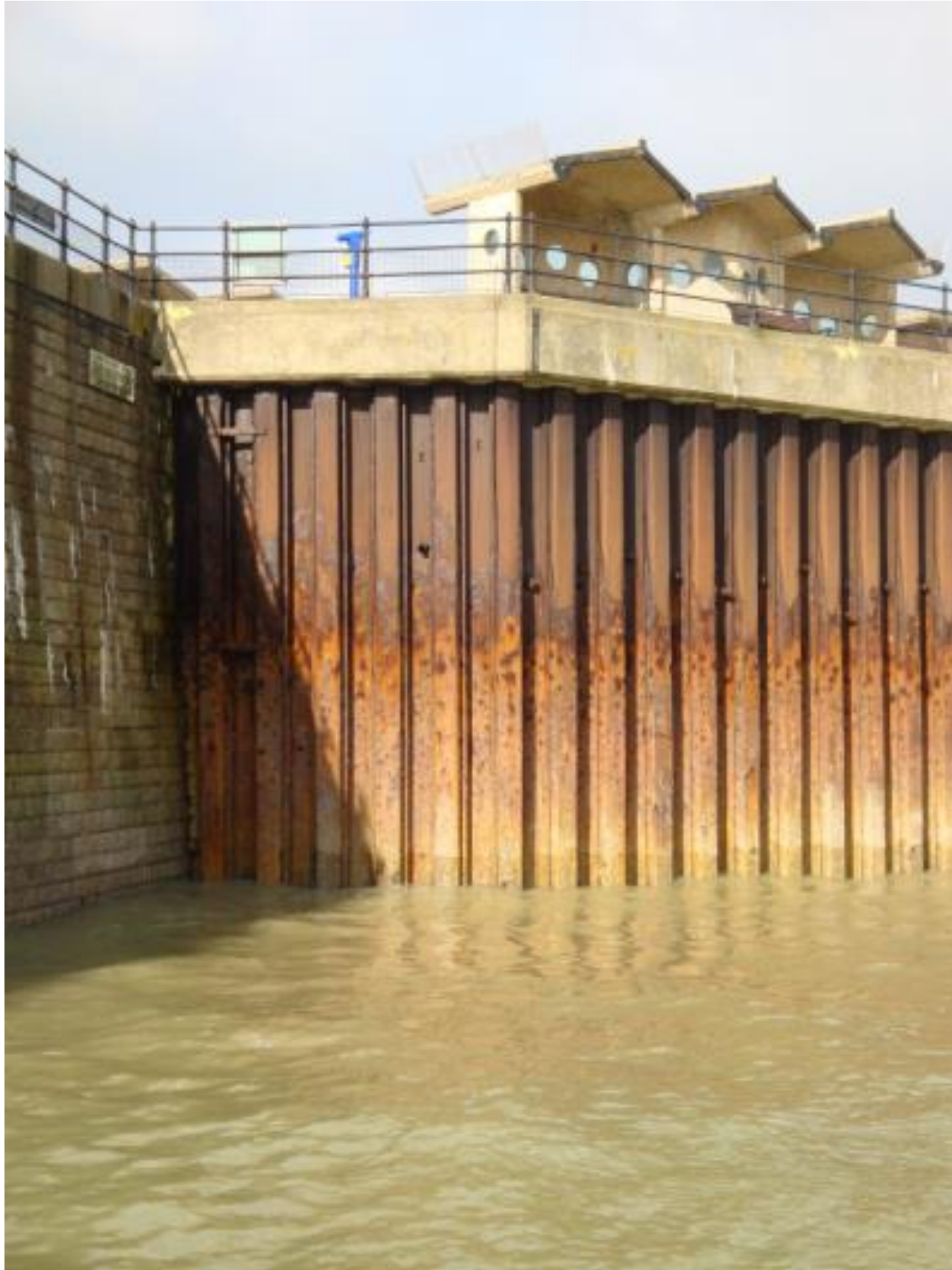
Plate 29: The connecting junction between the sheet piling and the masonry section of the pier, the piles change direction here, looking West, Atkins 2014A: 61.
