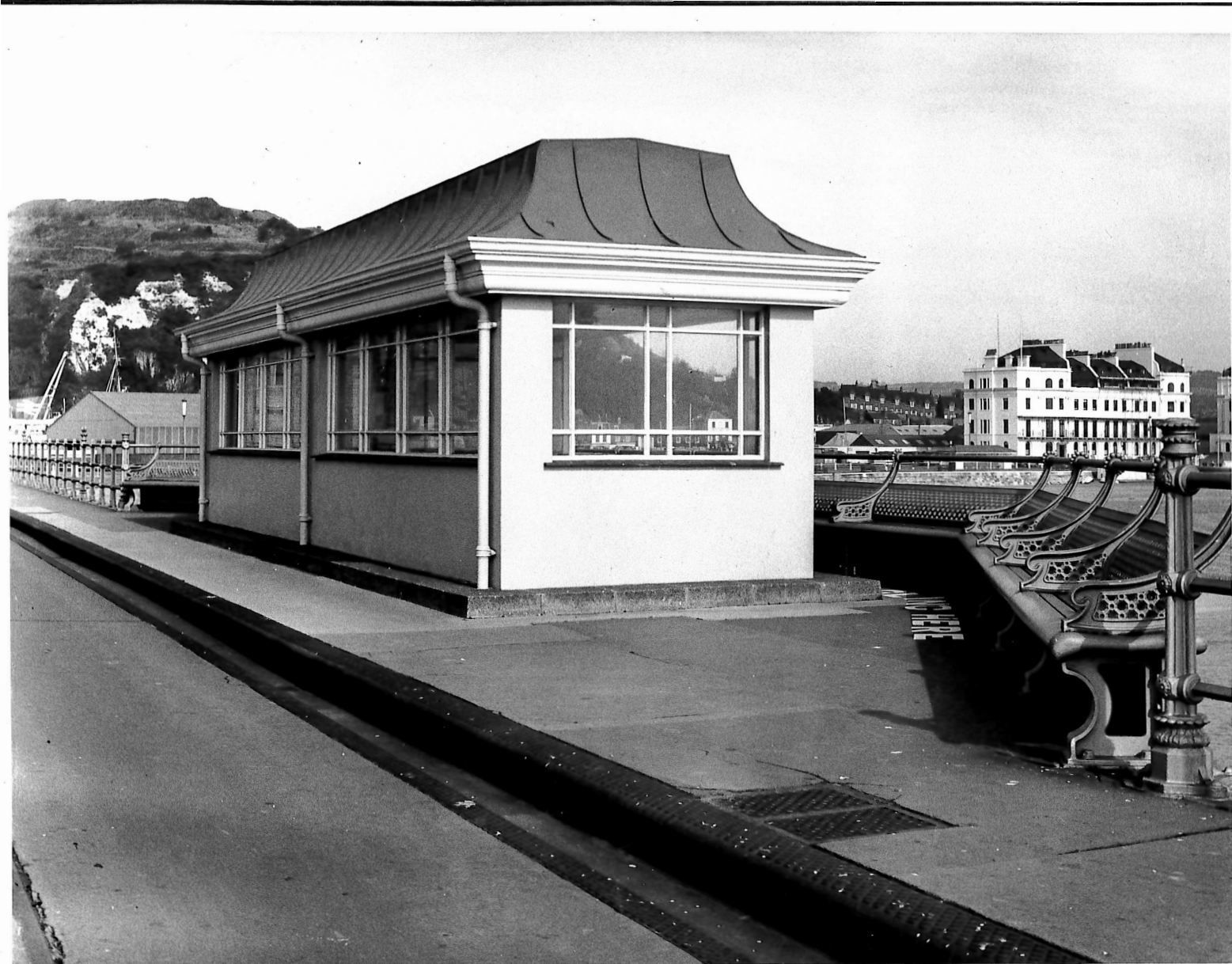
Figure 7: One of the shelters present on the pier, the original design for the seating can also be seen here, looking north-west, 05/04/1976, DHB.
