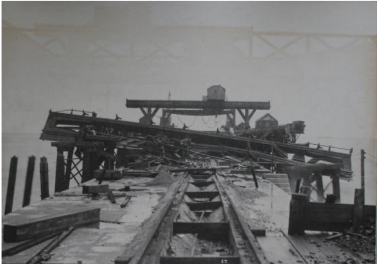
Plate 13- Some of the lifting equipment has collapsed, c.1895, Looking south-east, DHB.
