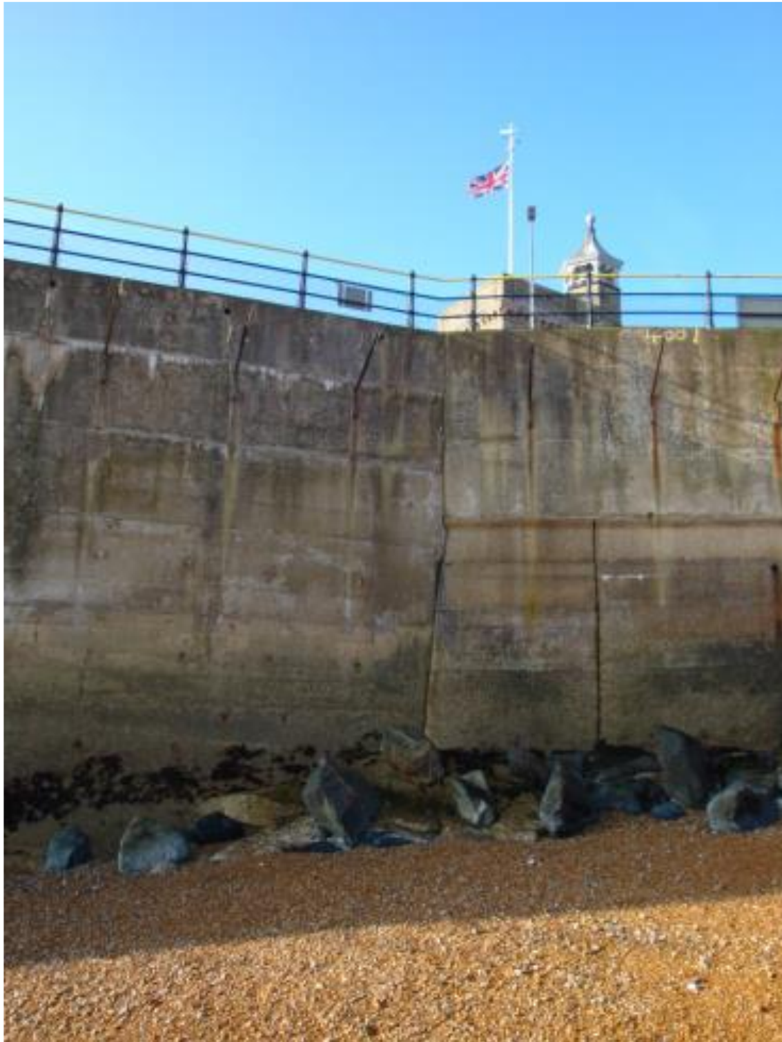
Plate 26: Sea wall and entrance ramp to the Prince of Wales Pier, looking West. Atkins 2014A: 100.
