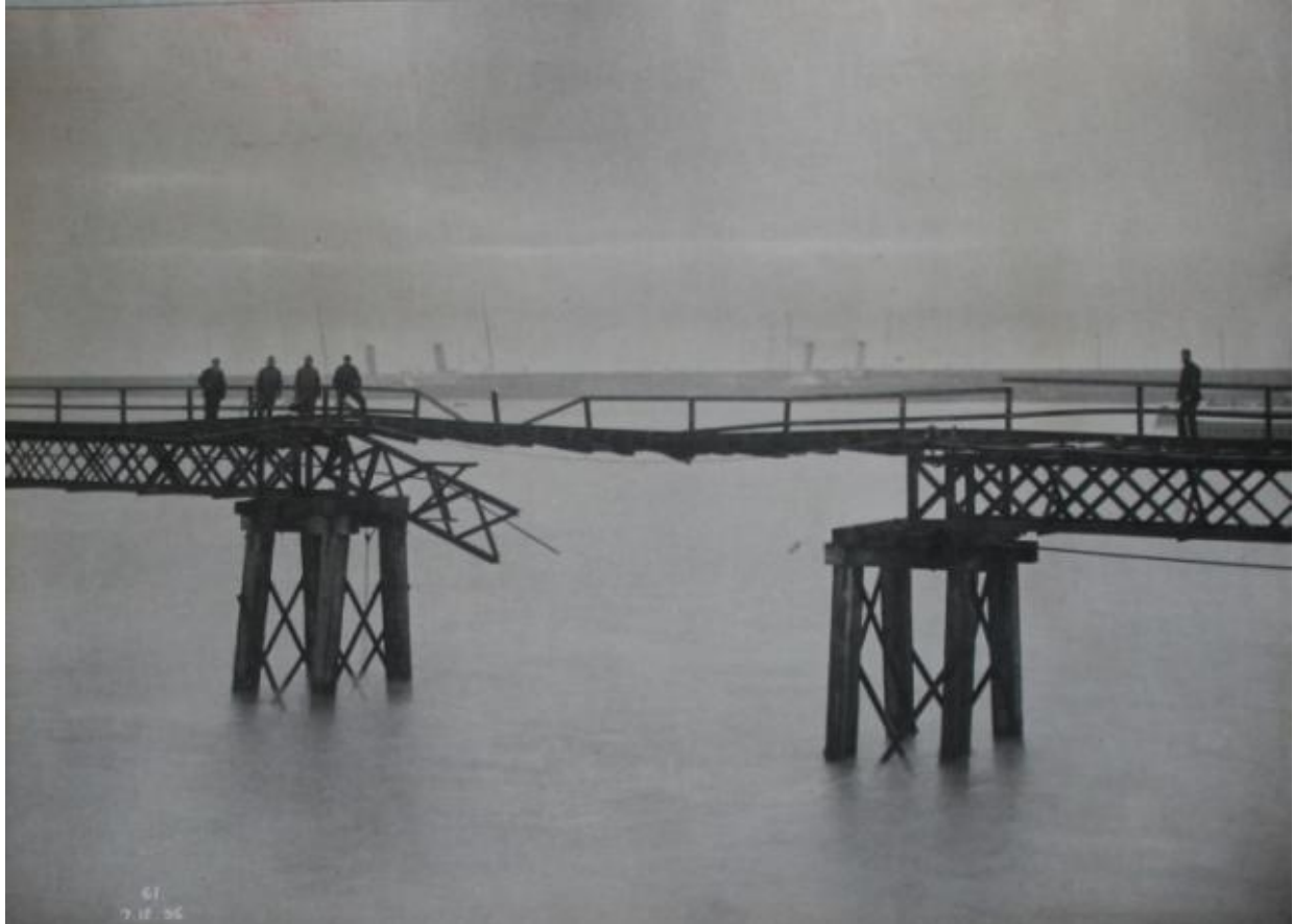
Plate 14- A partially collapsed gangway c.1895, Looking north-east, DHB.
