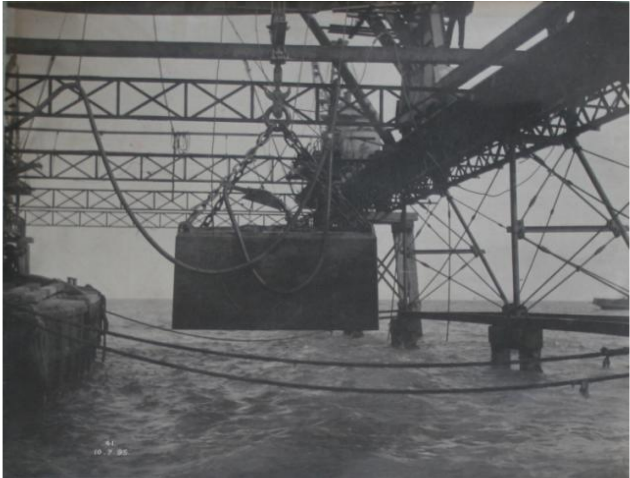
Plate 10- Thought to be a diving bell to allow men to work on the sea bed c.1895, DHB.
