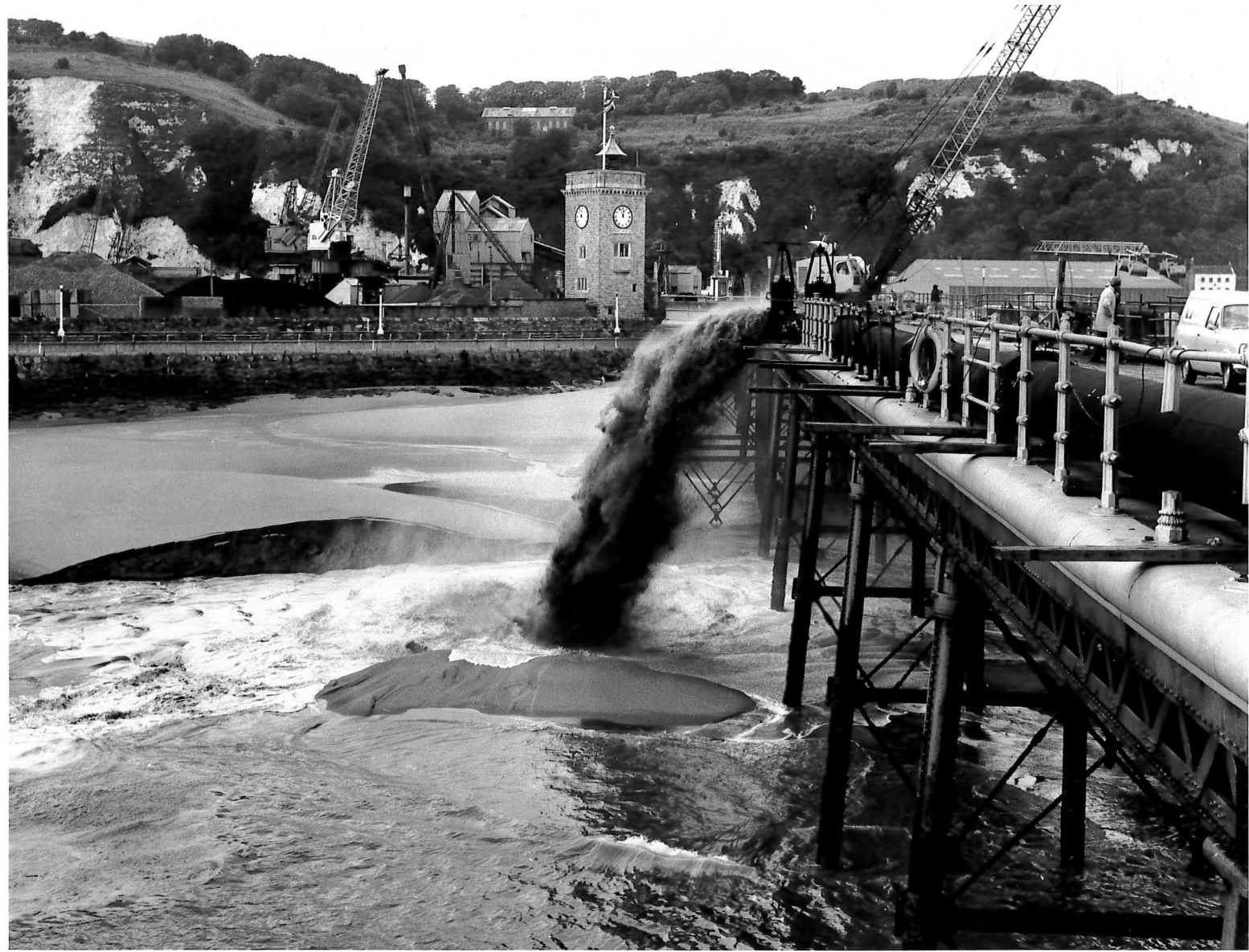
Figure 20: Sand being unloaded into the space to be reclaimed behind the Prince of Wales Pier, looking West, 14/09/1976, DHB.
