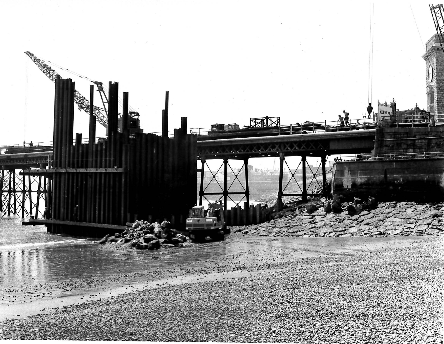
Figure 9: The beginnings of the sheet piling being installed to cover the original structure, looking South, 18/06/1976, DHB.
