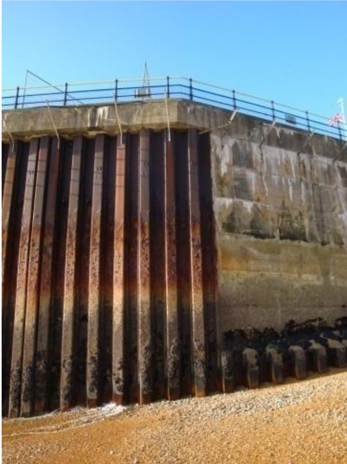
Plate 27: The point where the masonry work ends and the iron sheet piling begins on the East side of the pier, some sheet piling can also be seen at beach level, looking south-west, Atkins 2014A: 98.
