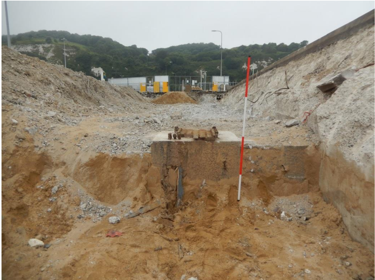
Plate 66: The position of the remaining connecting joist, looking West, 2m Scale, 28/7/2016, DHB.
