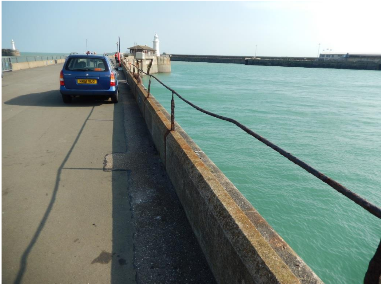
Plate 45: View looking seaward down the Prince of Wales Pier, towards the lighthouse, 09/09/2015, DHB.
