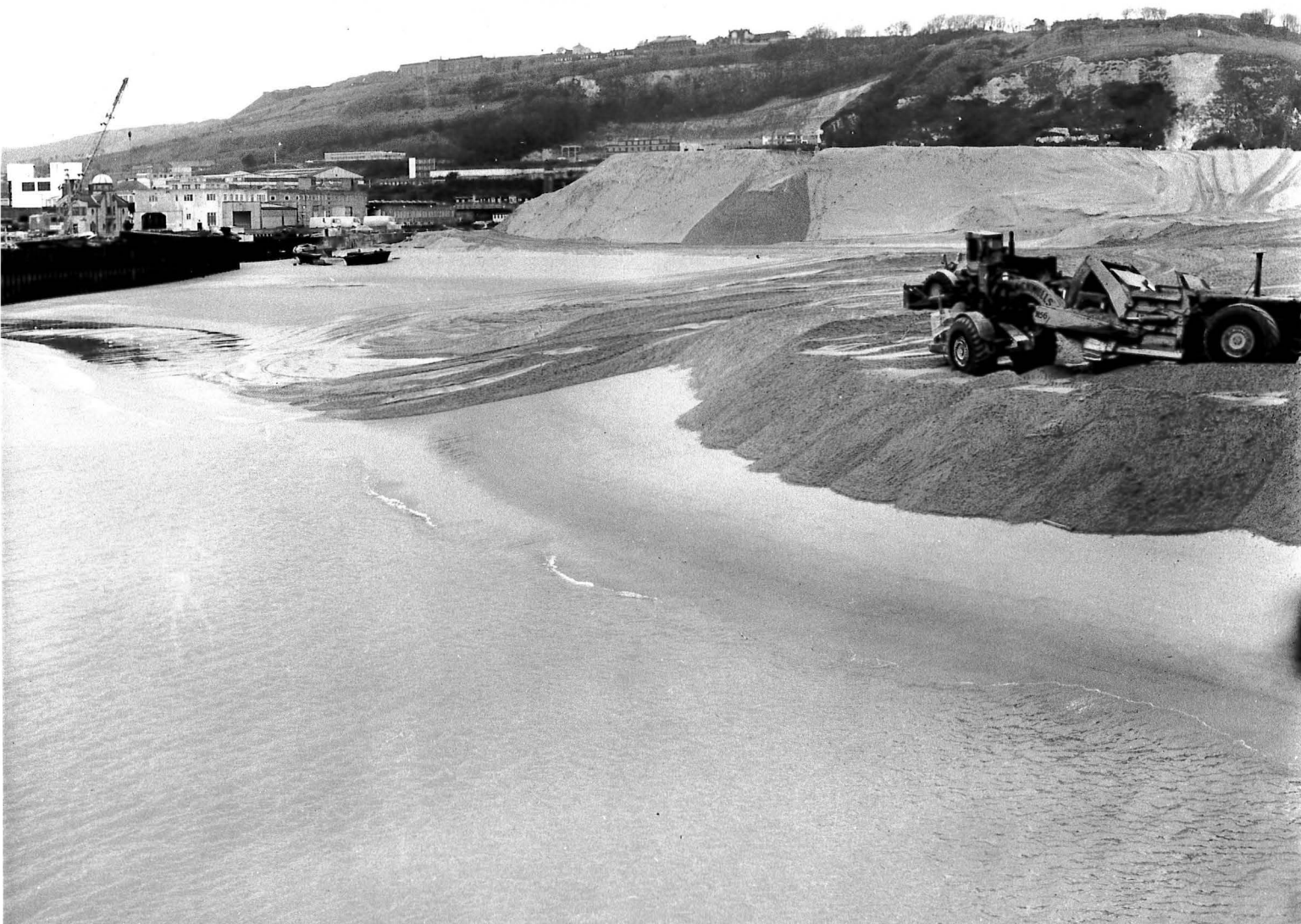
Figure 1: The reclamation of land with the use of sand before the main construction of the hoverport apron could start, looking north-west, 13/01/1976, DHB.
