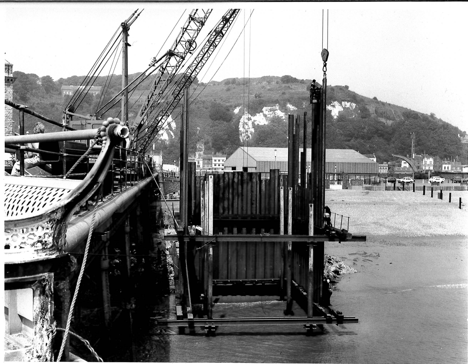
Figure 10: Sheet piling being put into place, seating is again visible here, looking West, 18/06/1976, DHB.
