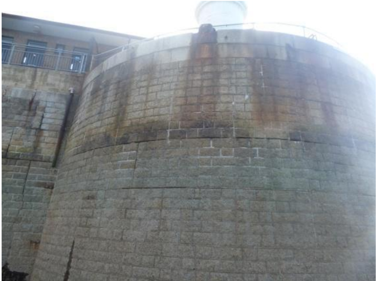
Plate 33: The side view of the roundhead seaward ending of the pier, with a galvanised steel hand rail, looking North, Atkins 2014B: 34.
