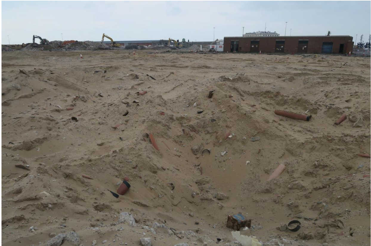
Plate 61: One of the original pile foundations for the Prince of Wales Pier can be seen in the foreground, with the context of the Lord Warden House, looking South, 26/10/16, DHB.
