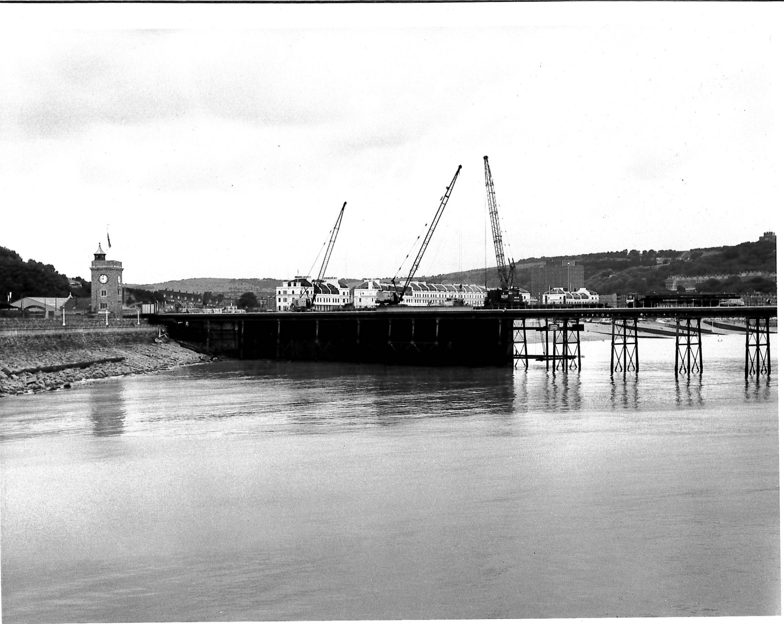
Figure 17: Sheet piling has been installed, the clock tower and waterloo crescent are also visible here, looking north-west, 02/08/1976, DHB.
